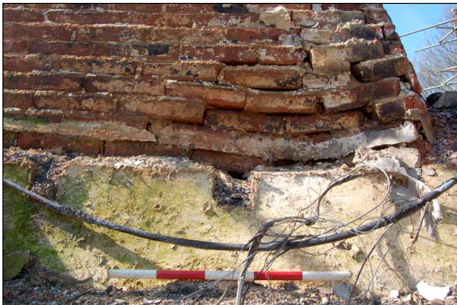
Plate 10 Stack brickwork bonded with earth mortar
