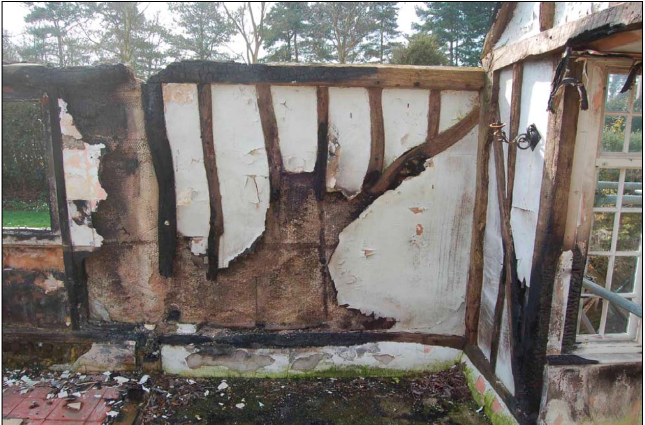
Plate 6 Primary-braced studwork in south-west bay
