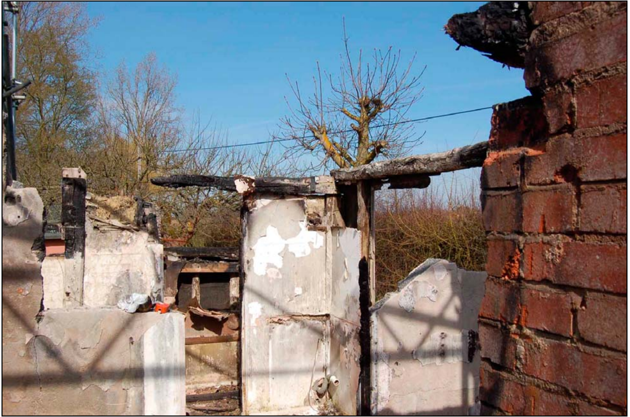
Plate 3 North-east bay viewed to lean-to showing bay post to left
