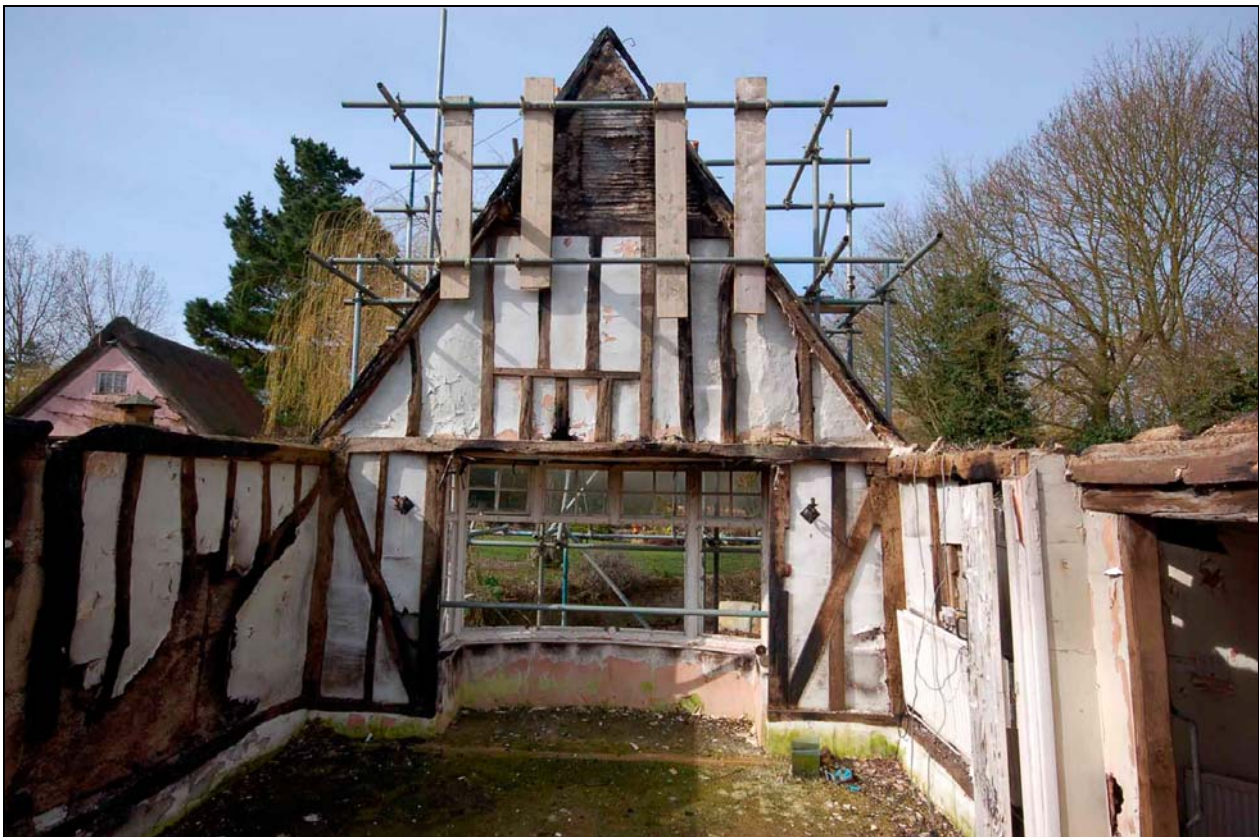
Plate 4 Timber-framing in south-west bay
