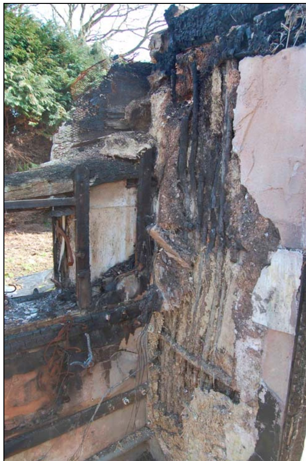
Plate 8 Detail of wall fabric on north-west side of cottage
