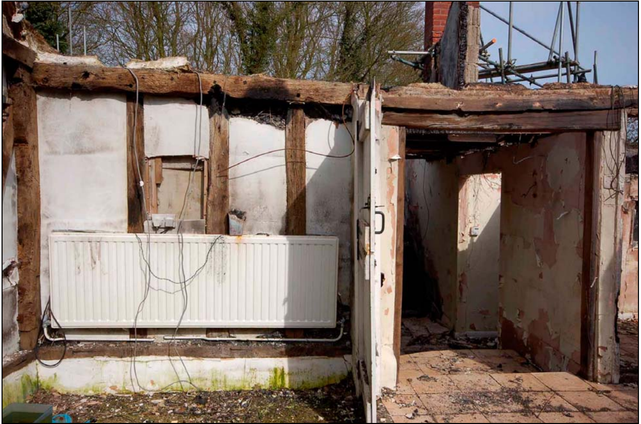
Plate 5 Pegged studwork in south-west bay
