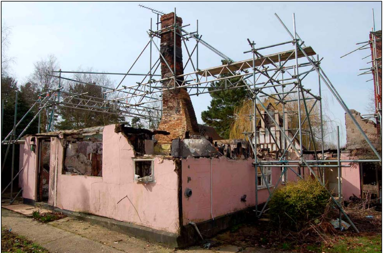
Plate 2 Cottage viewed to south with lean-to in foreground
