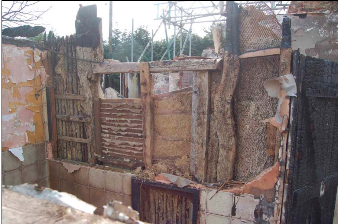
Plate 7 Exposed features on north-west wall of cottage
