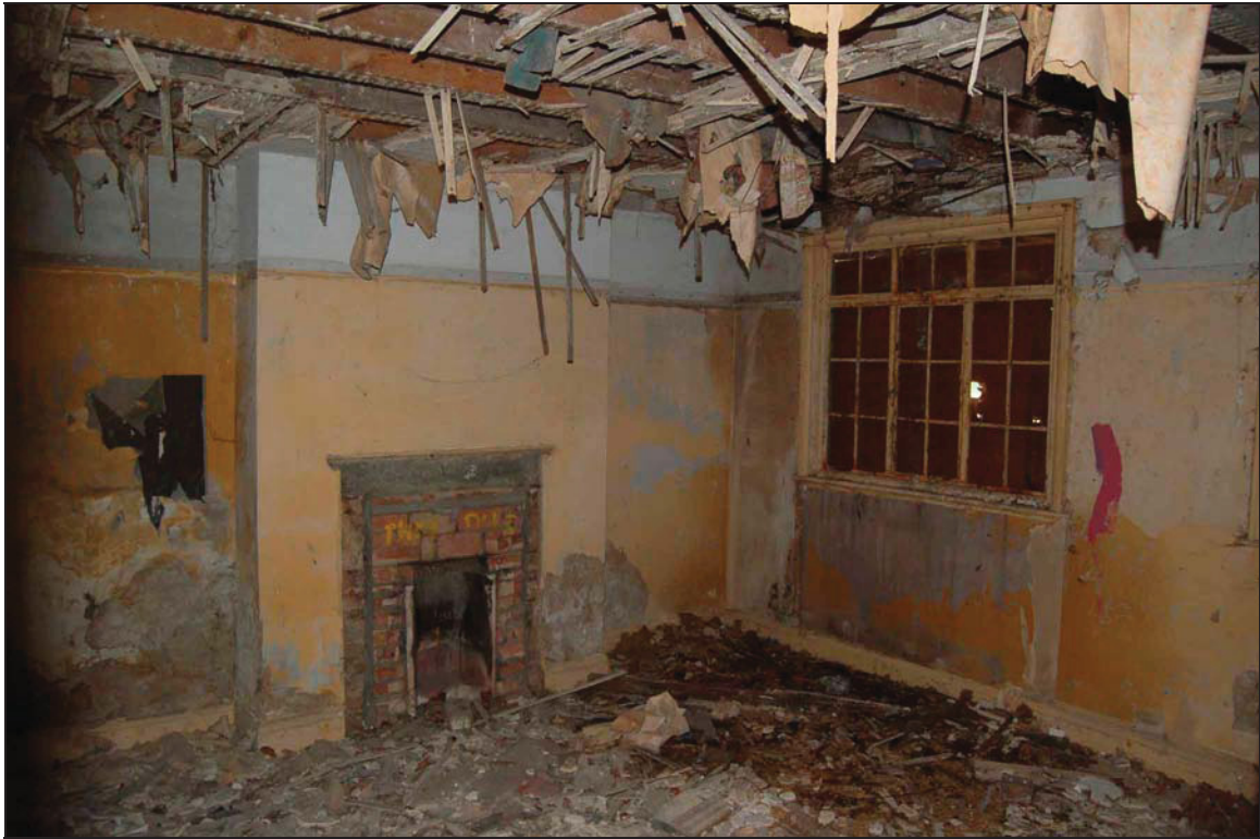
Plate 26 Front room inside Church Cottage
