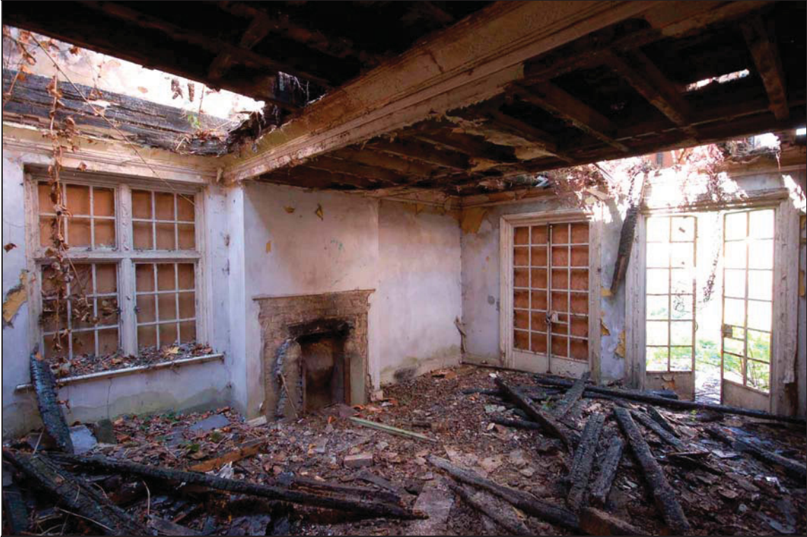
Plate 9 View to veranda and former entrance inside Church House
