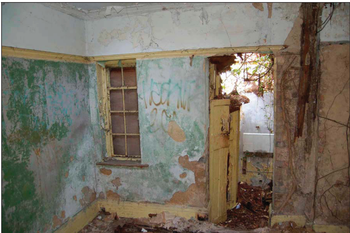
Plate 22 Back room in extension viewed towards western annex
