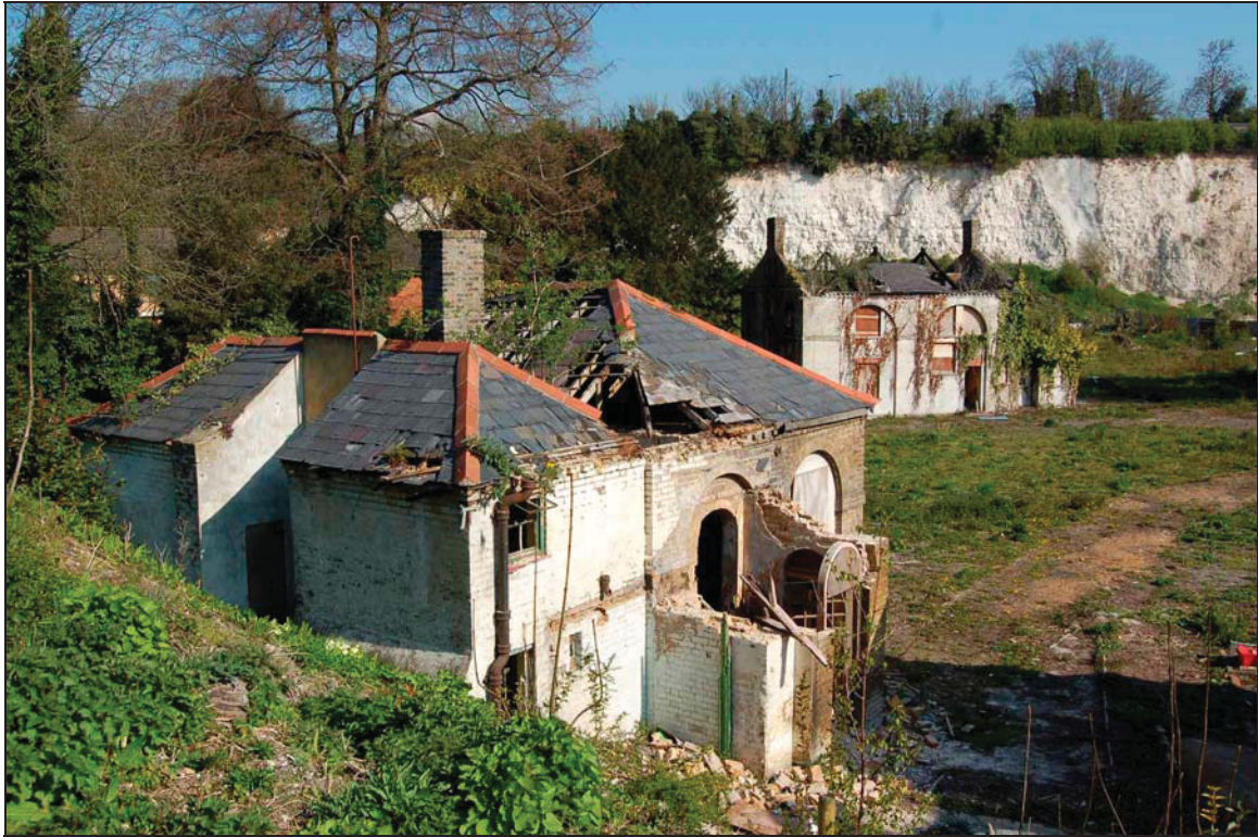
Plate 15 Church Bungalow viewed to north-west with Church House in background
