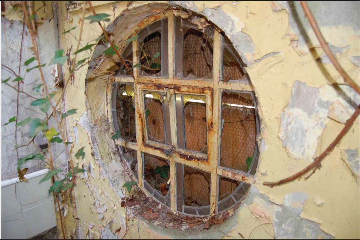
Plate 23 Round leaded window in western annex
