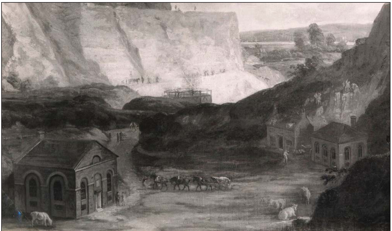
Plate 2 Detail of Church Hollow viewed south-eastwards from Tank Lane in 1796
