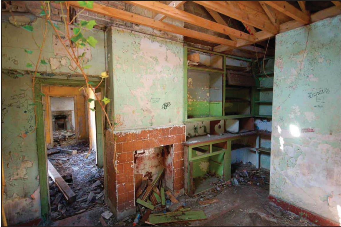
Plate 11 Kitchen annex at Church House in former vestry
