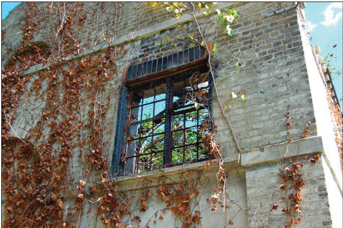
Plate 6 Inserted metal-framed window on right side of chapel door
