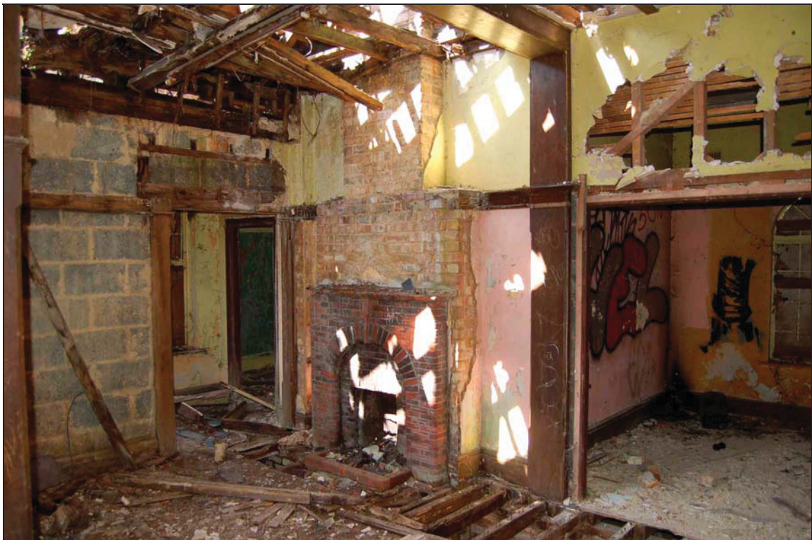
Plate 18 View across classroom into extension and other room
