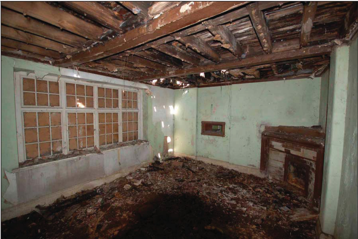
Plate 10 View to former doorway into vestry
