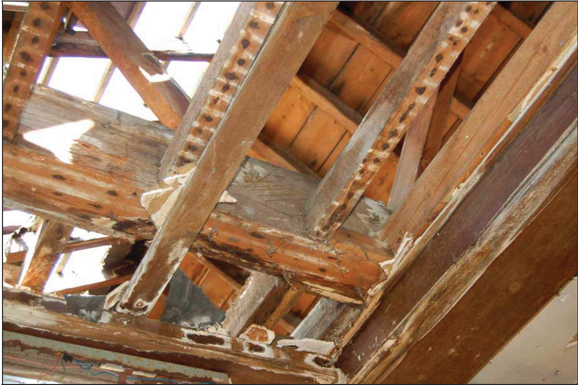
Plate 21 Suspended ceiling in classroom with carpenter's mark (XIII) on 18th century beam
