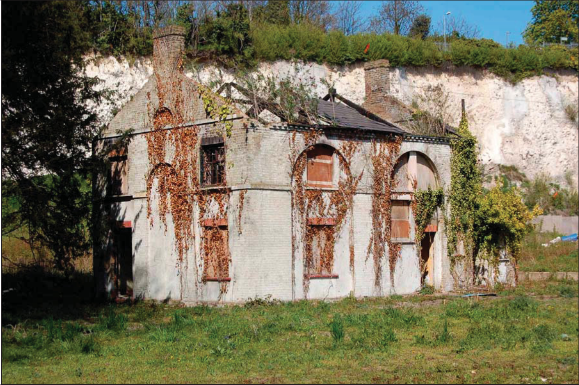
Plate 3 Church House viewed to north
