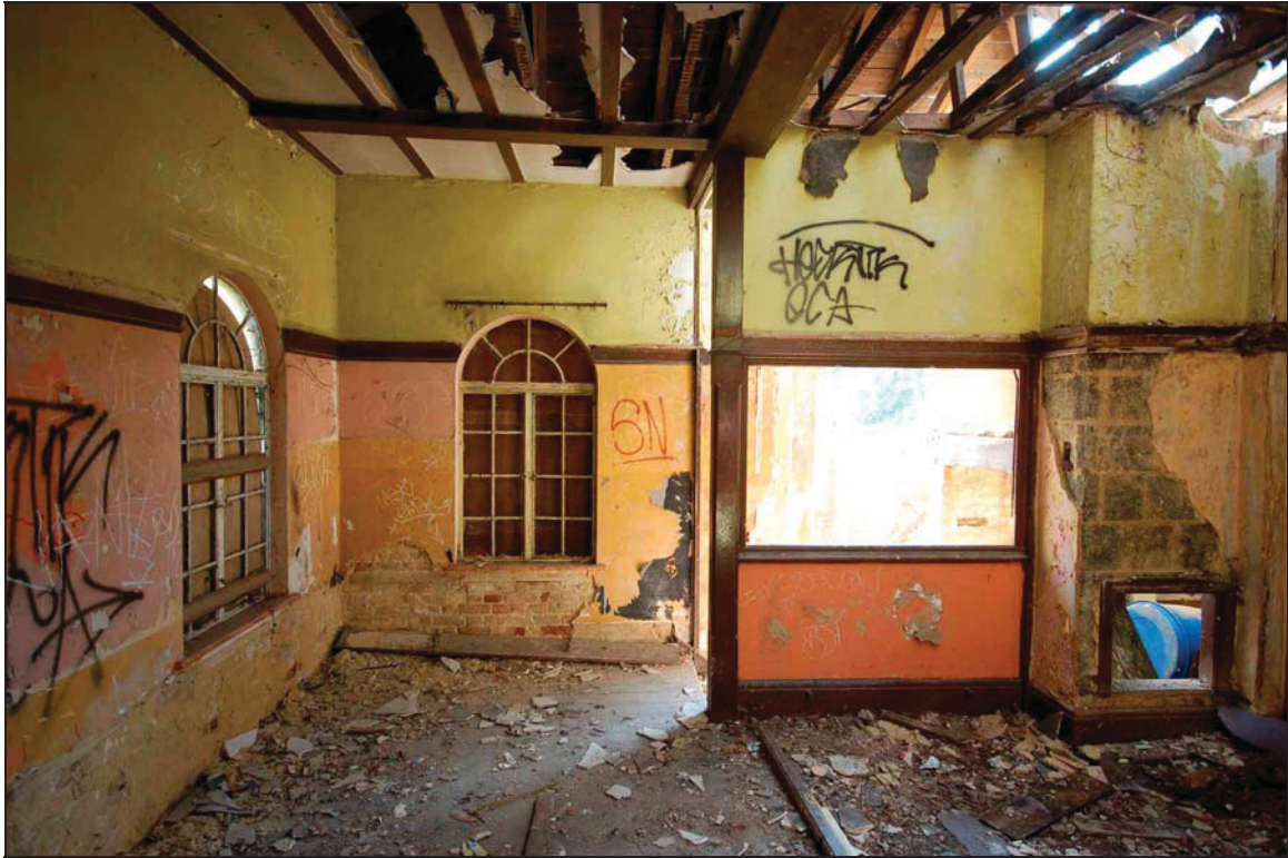
Plate 19 View across classroom to entrance (east)
