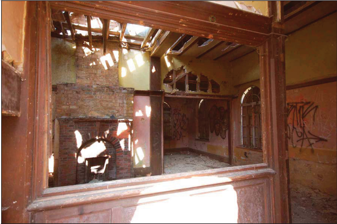
Plate 17 View from entrance to Church Bungalow into former classroom
