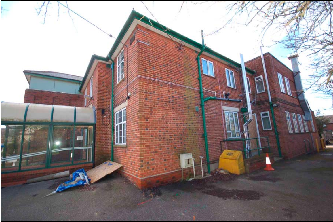
Plate 3 North elevation viewed to south-west
