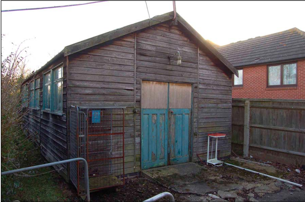
Plate 29 Shed viewed to south-west
