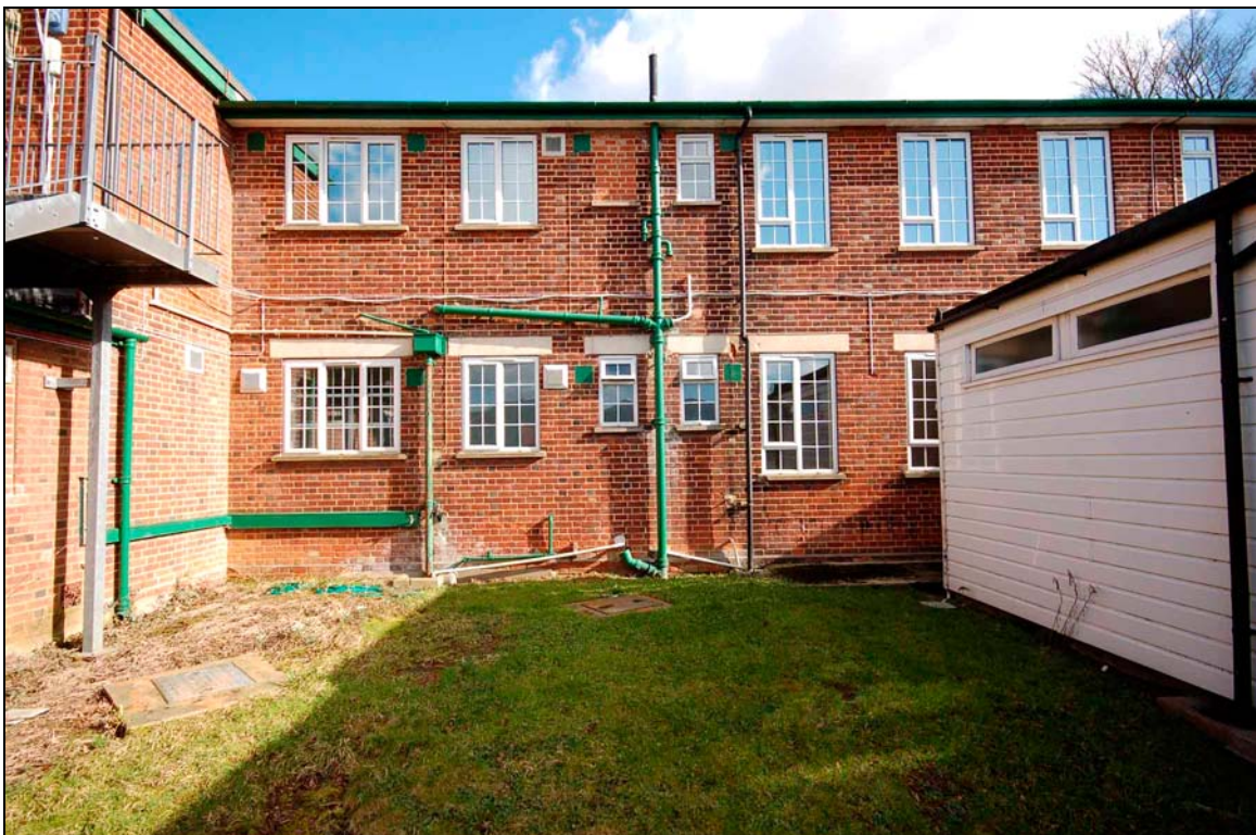
Plate 8 West elevation of hospital between later extensions
