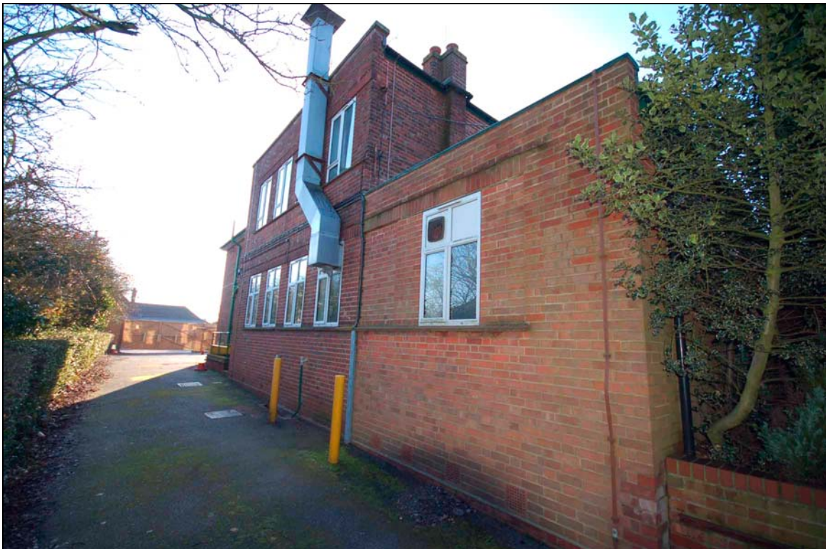
Plate 4 North elevation viewed to south-east
