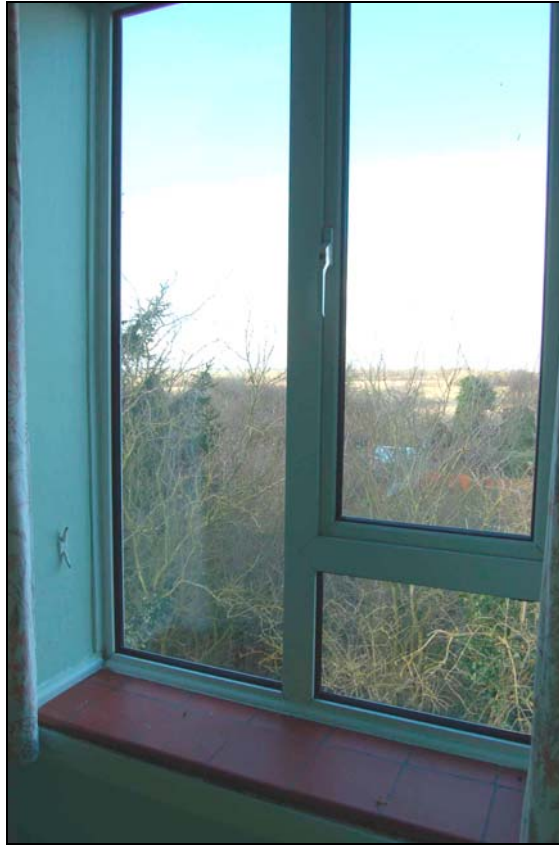
Plate 27 Window in day room
