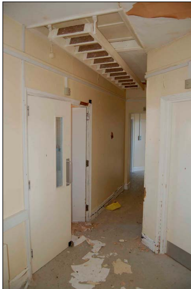
Plate 22 1933 corridor and loft hatch
