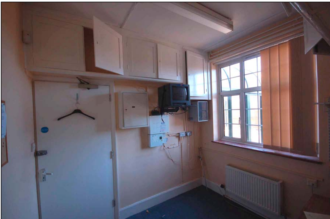
Plate 12 Office in admin. block
