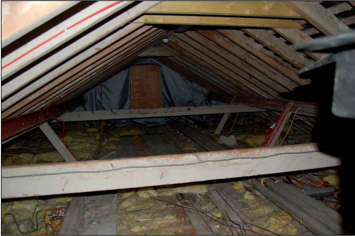
Plate 23 Roofspace viewed to south
