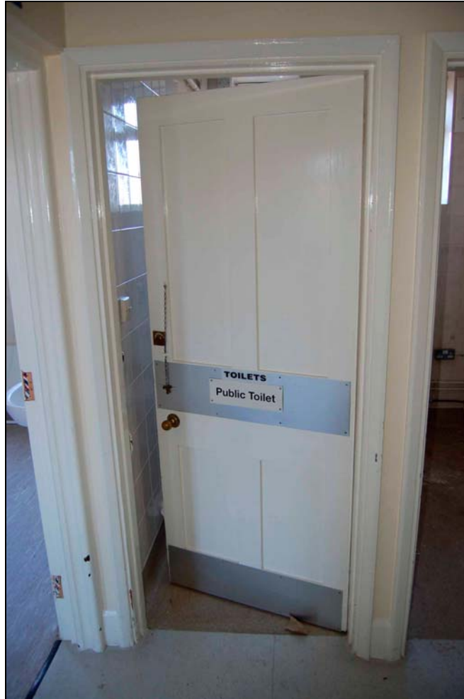
Plate 15 Original door to ground floor public toilet
