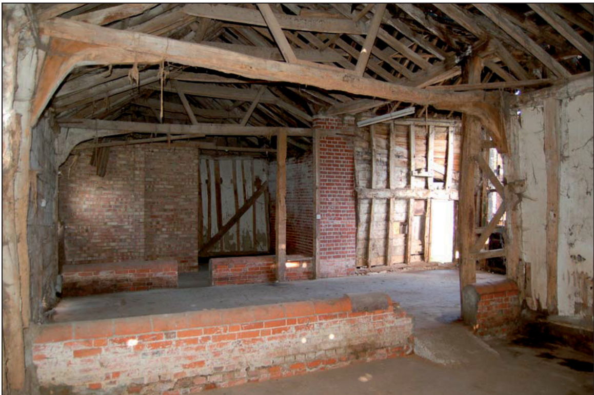
Plate 8 Interior of barn viewed to north
