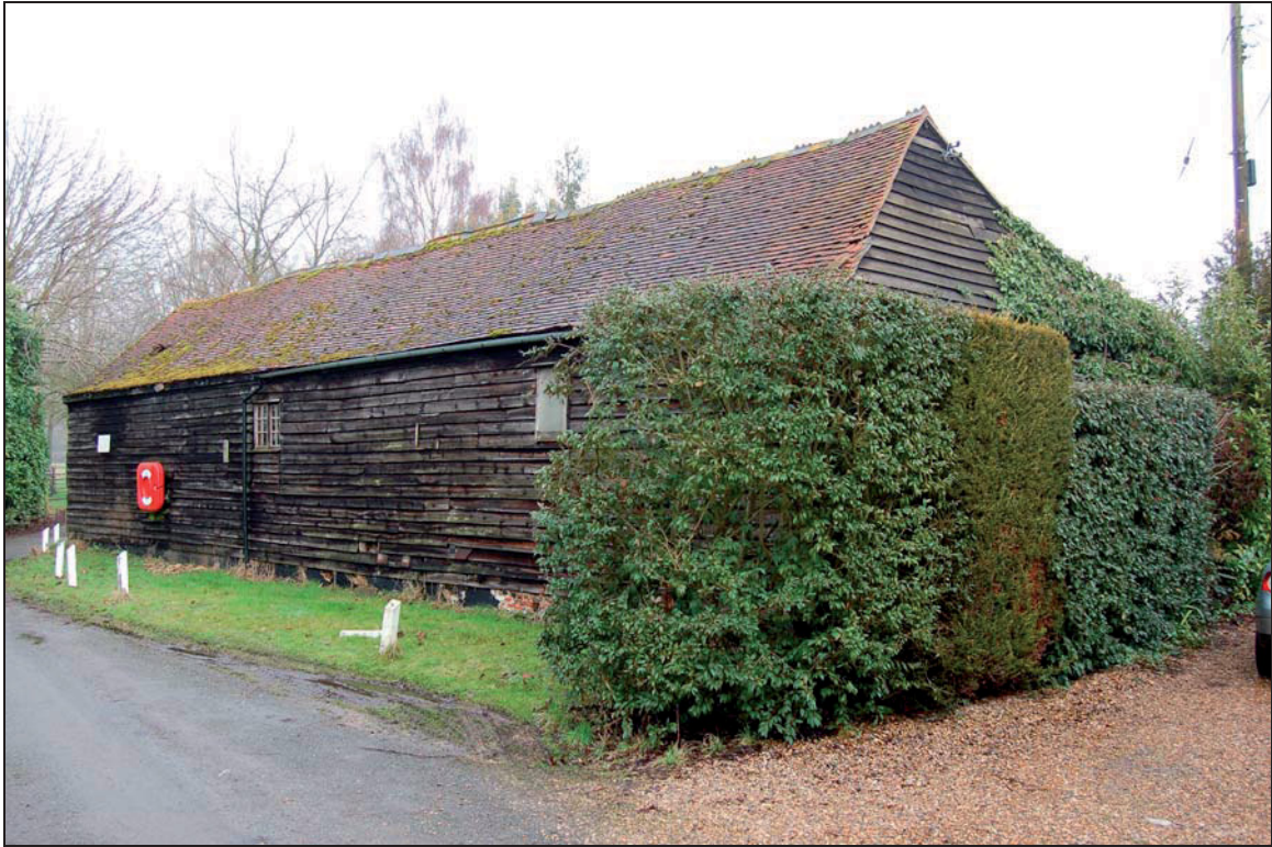
Plate 5 Rear of barn viewed to north
