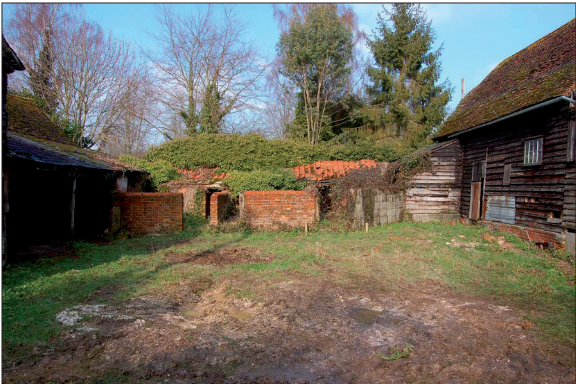
Plate 18 Piggeries viewed to north from yard
