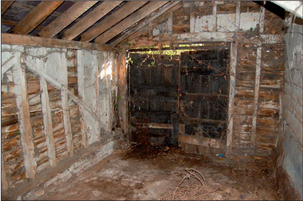
Plate 17 Interior of loose box 5 viewed to south
