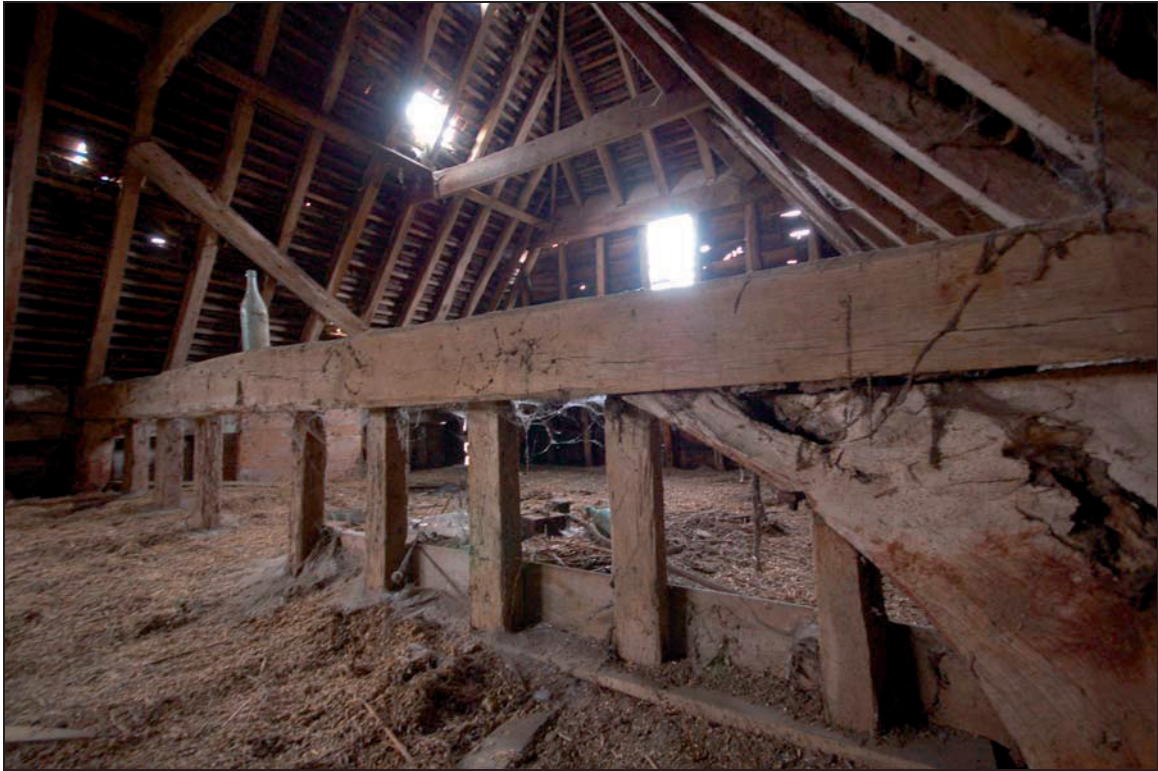
Plate 25 Chaff store viewed to south, showing low partition
