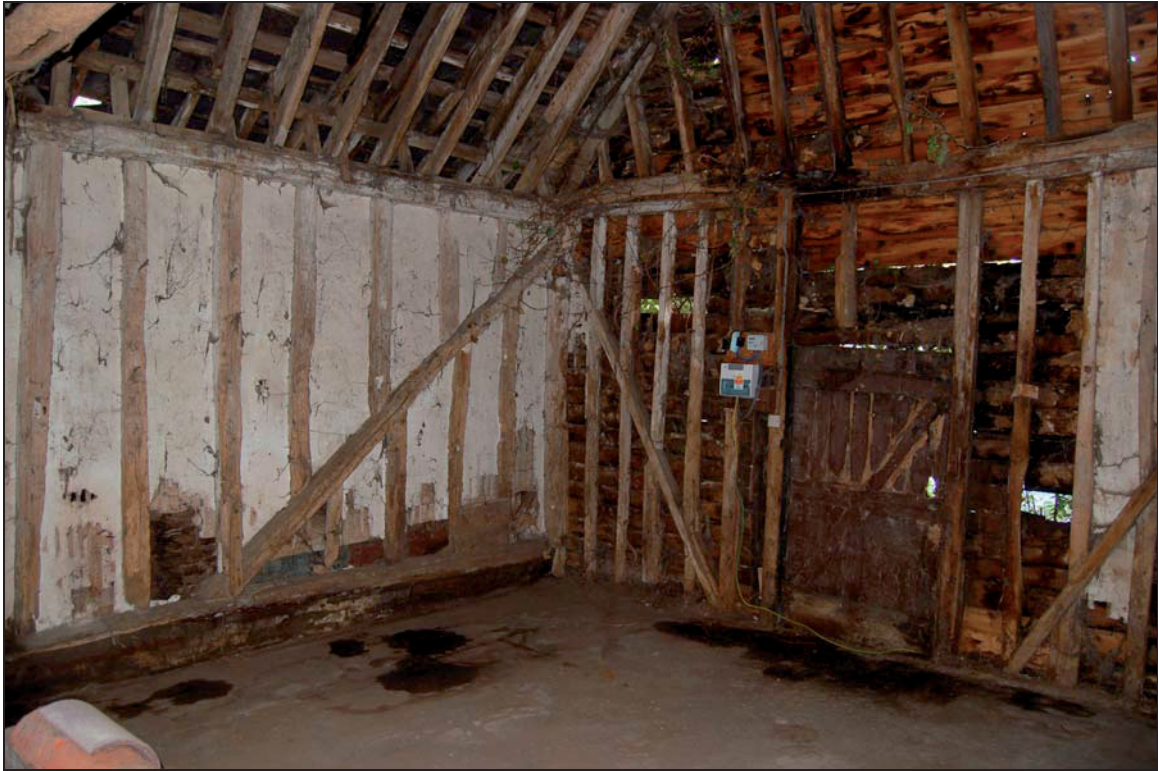
Plate 11 Wall-framing detail viewed to south-east
