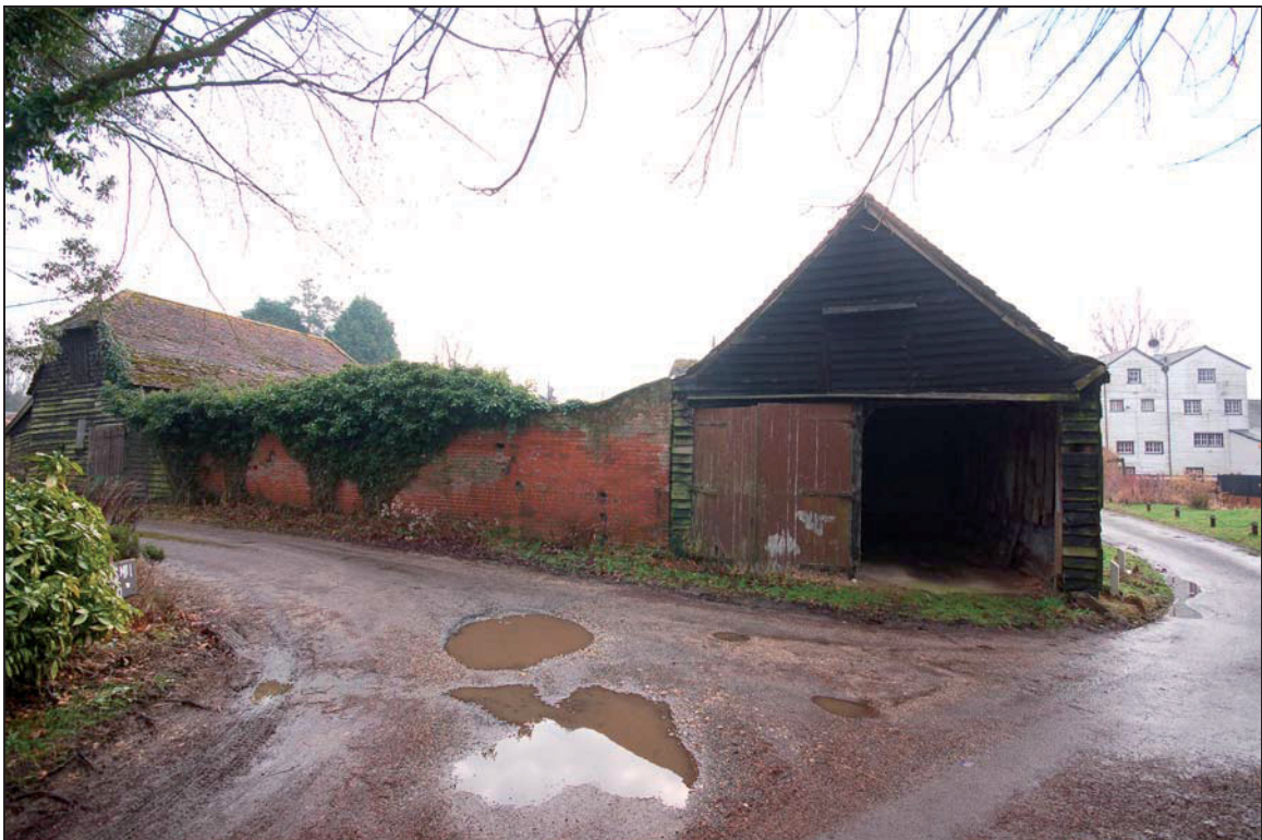
Plate 12 Wagon lodge and Listed brick wall viewed to south
