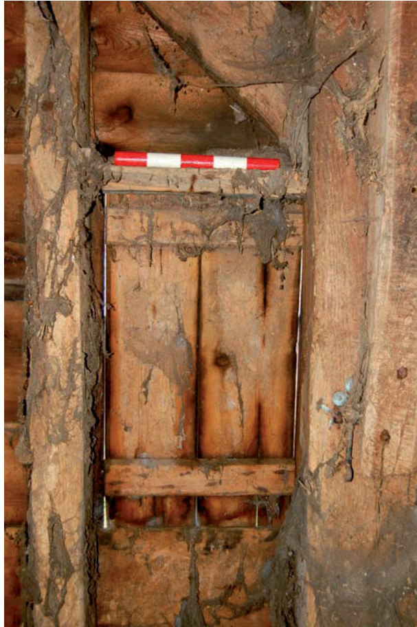
Plate 23 Stable vent on west wall (25cm scale)
