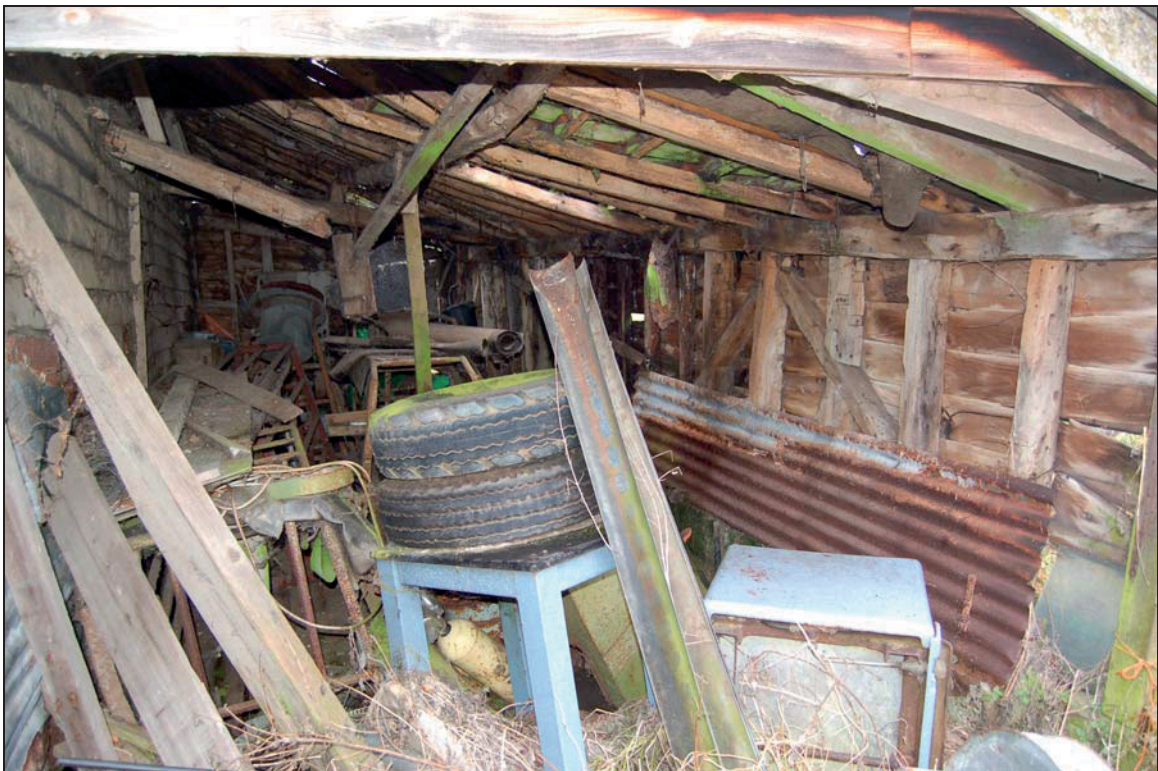
Plate 26 Interior of lean-to 8 viewed to north
