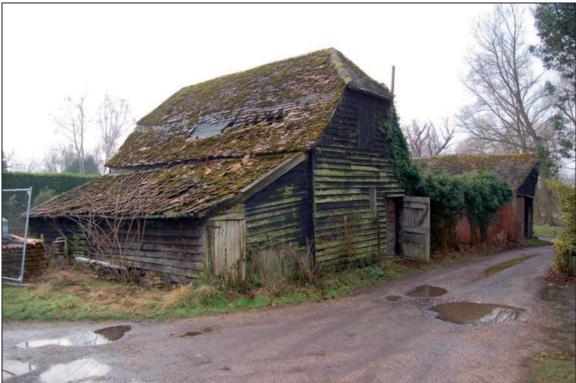
Plate 20 Stable and lean-to 8 viewed to south-west
