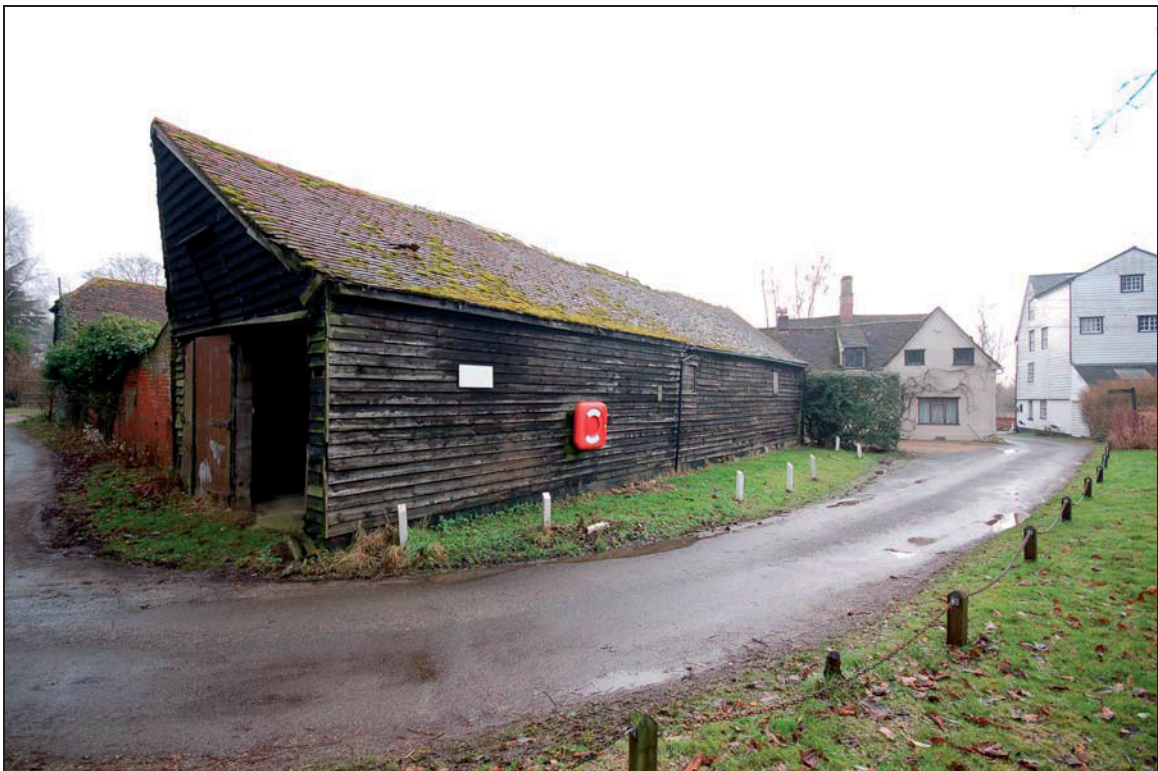
Plate 6 Barn viewed to south with former farmhouse and mill in background
