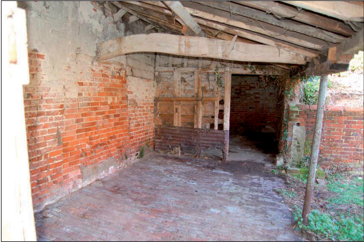
Plate 15 Interior of cow shed 3 viewed to north
