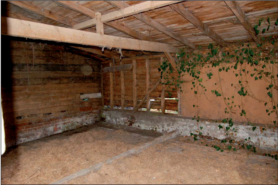
Plate 27 Interior of cow house viewed to north-east
