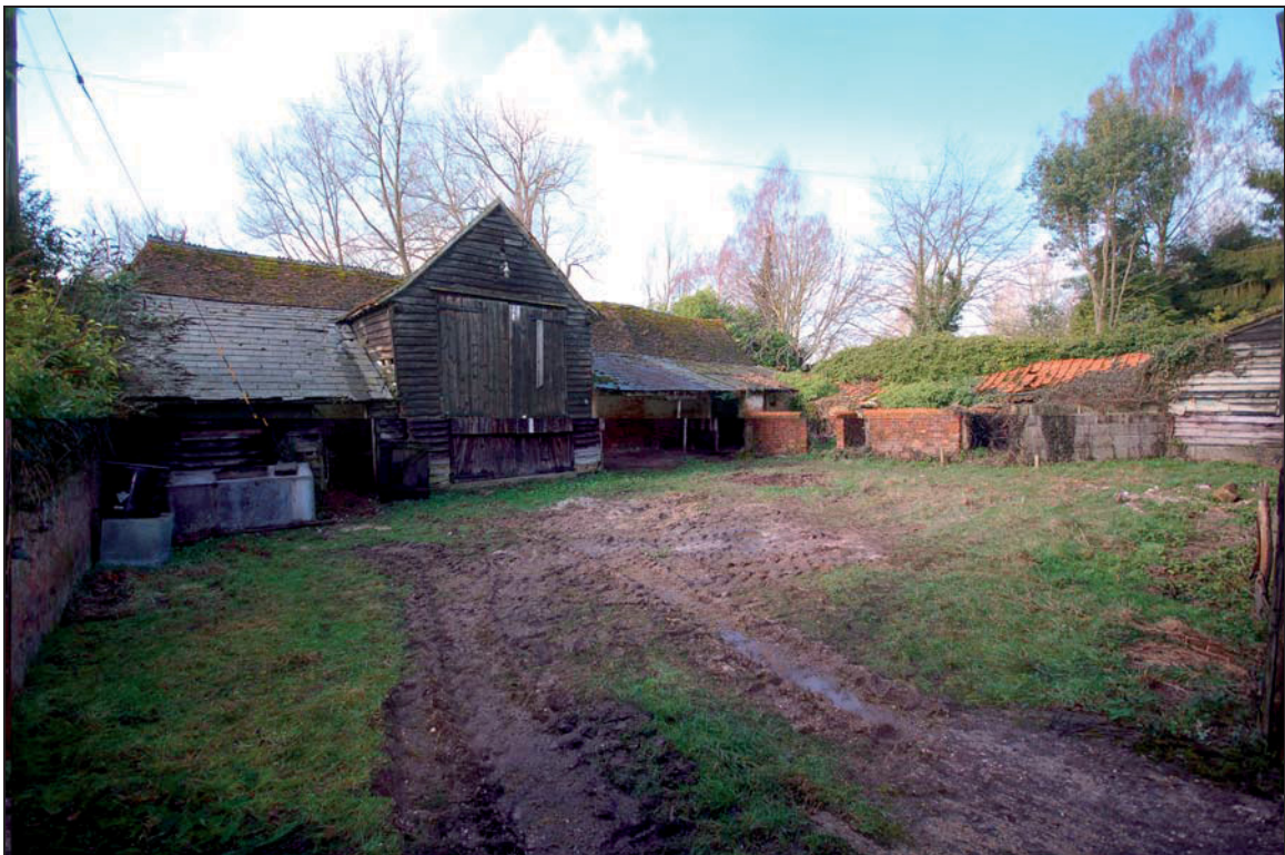
Plate 2 Main barn range
