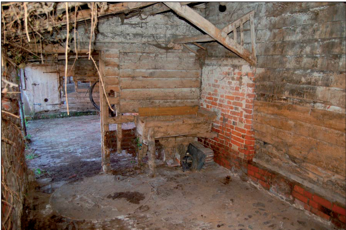
Plate 16 Interior of loose box 4 viewed to south
