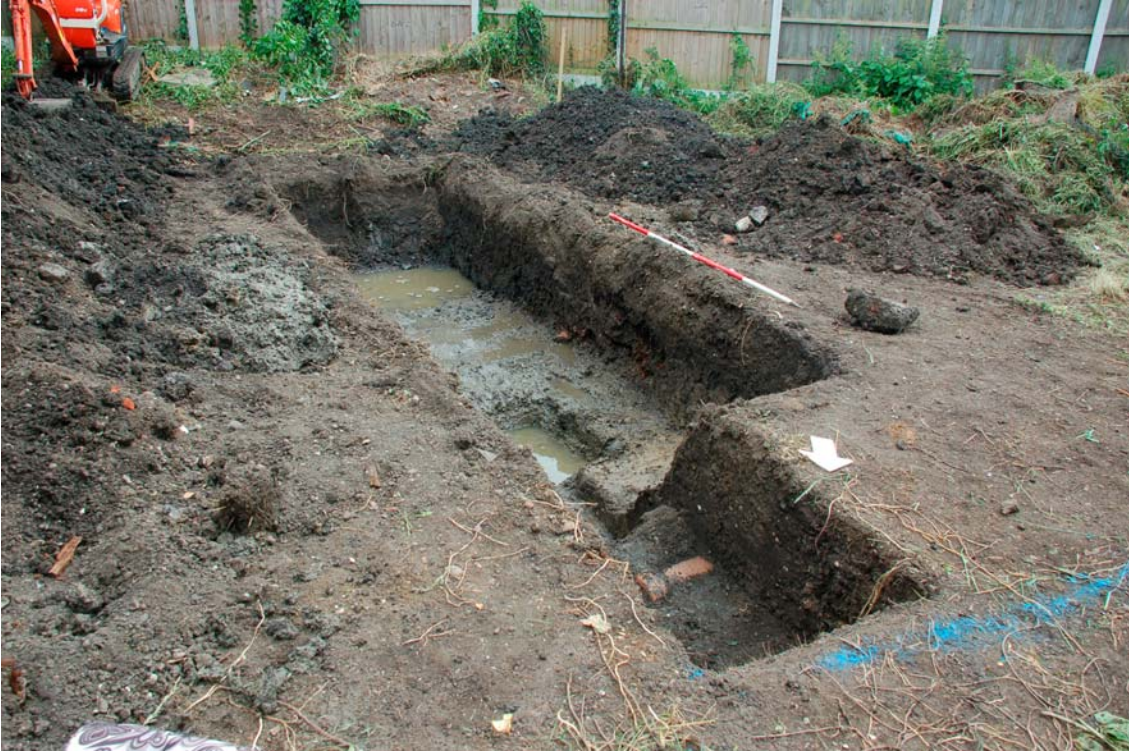
Plate 3. Trench, looking south. 2m scale.
