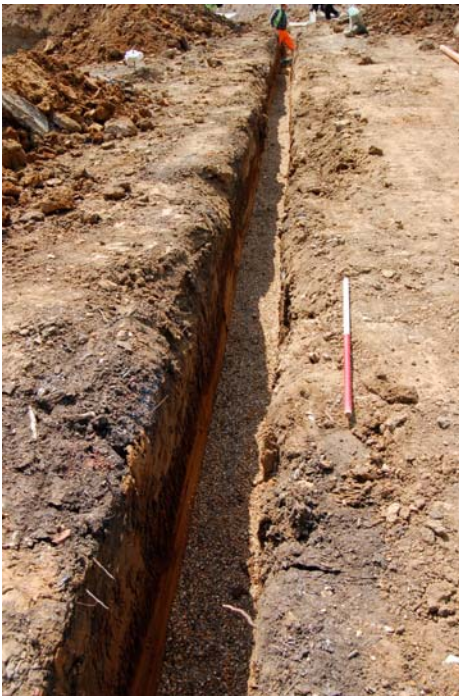
Plate 3. Drain run, looking north. 1m scale
