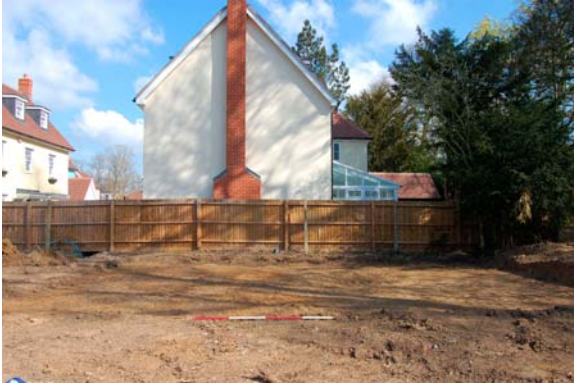
Plate 1. Shallow footprint, north-eastern corner. Looking north. 2m scale.
