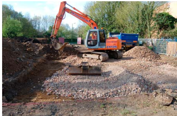
Plate 6. Partially backfilled footprint, looking south
