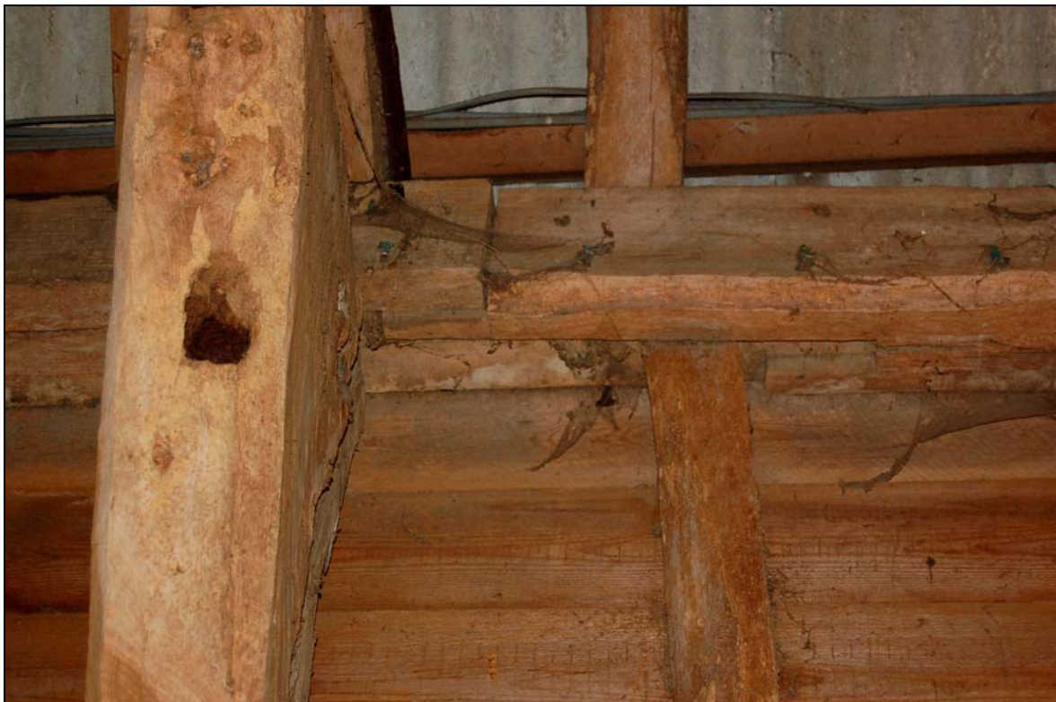
Plate 16 Bladed scarf joint on east wall of stables
