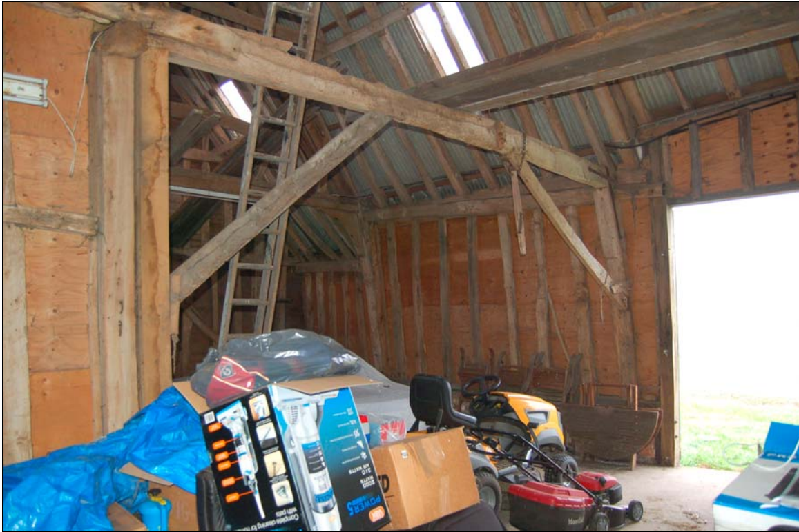
Plate 9 Open truss between midstrey and western bay and north door
