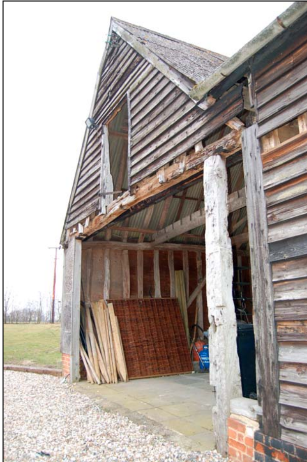
Plate 11 Cartlodge entrance, with stable built up to it, viewed to north-east
