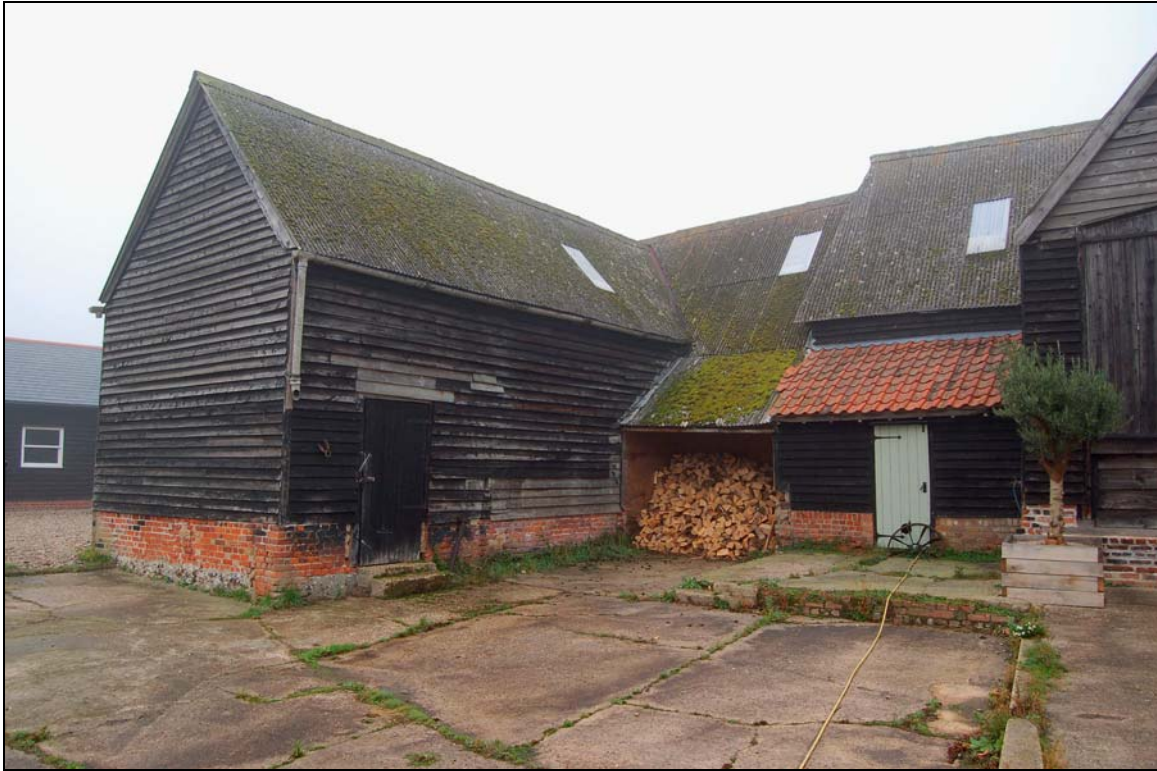
Plate 5 Stables and former pig sty viewed to north-west
