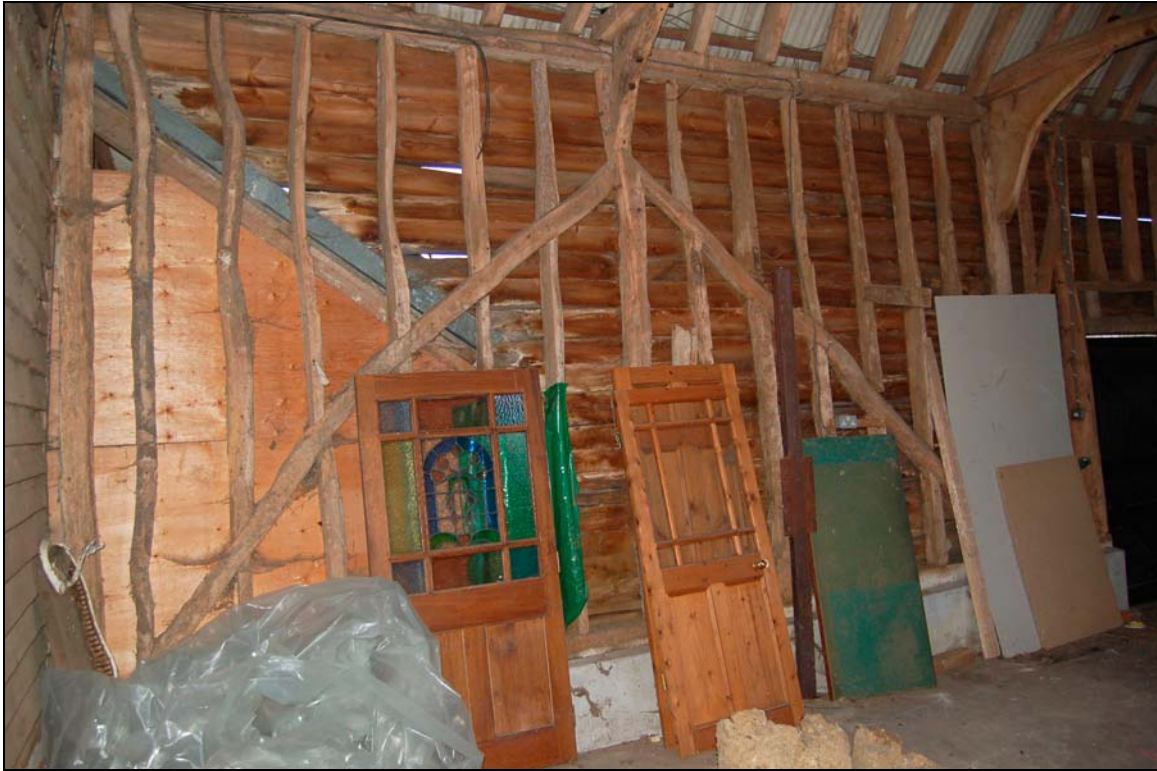
Plate 15 Wall-framing on west wall of stables
