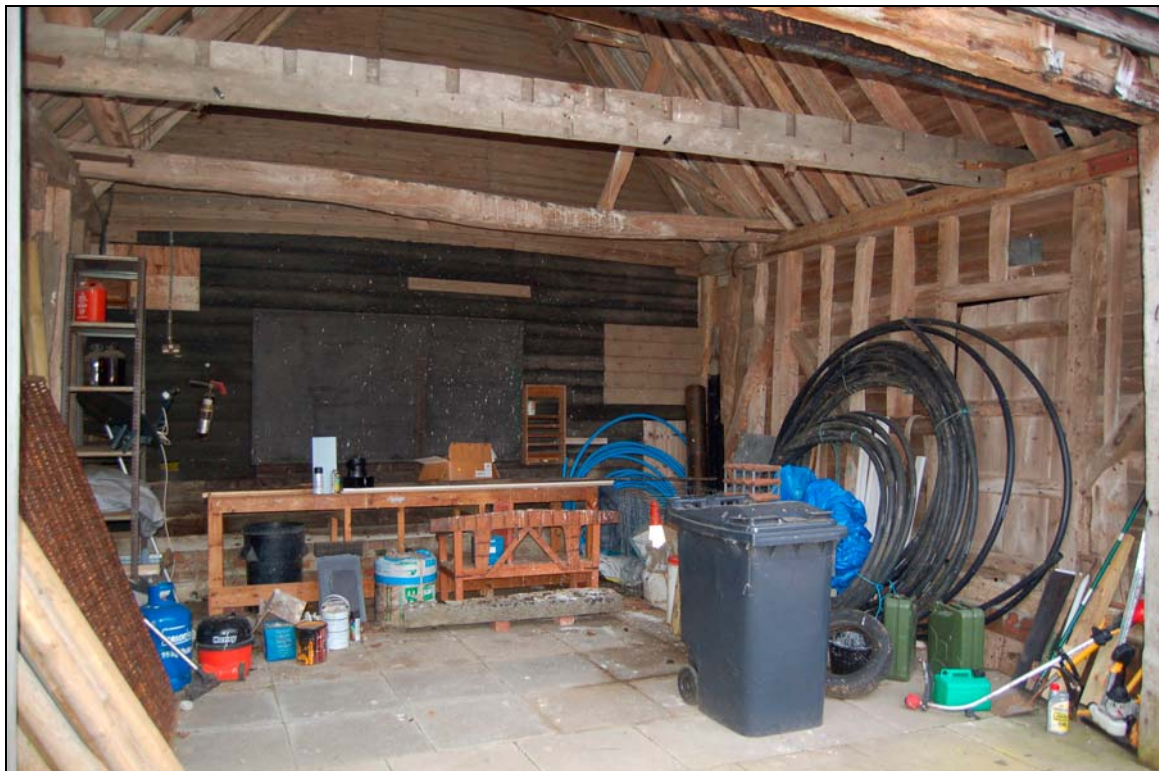
Plate 12 Interior of cartlodge viewed to east
