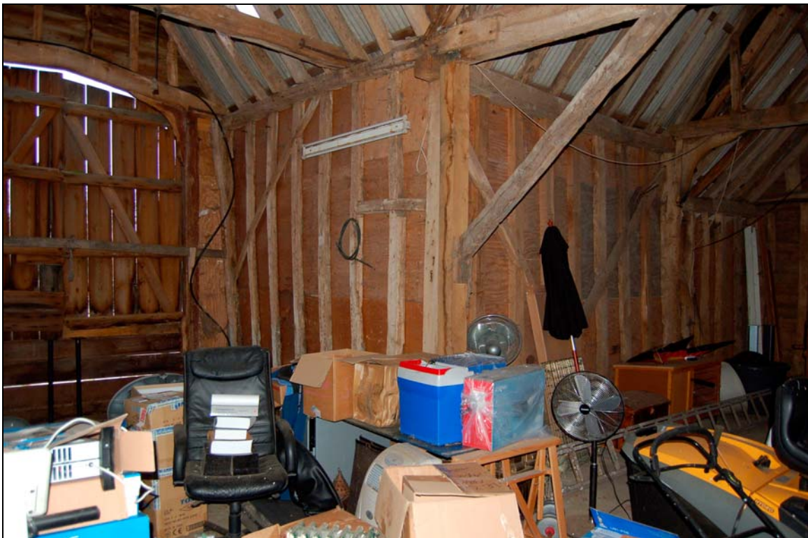
Plate 8 View across midstrey to porch (south-west)
