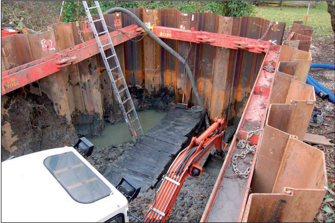
Plate 3 Chunker viewed to south-east from top of coffer dam
