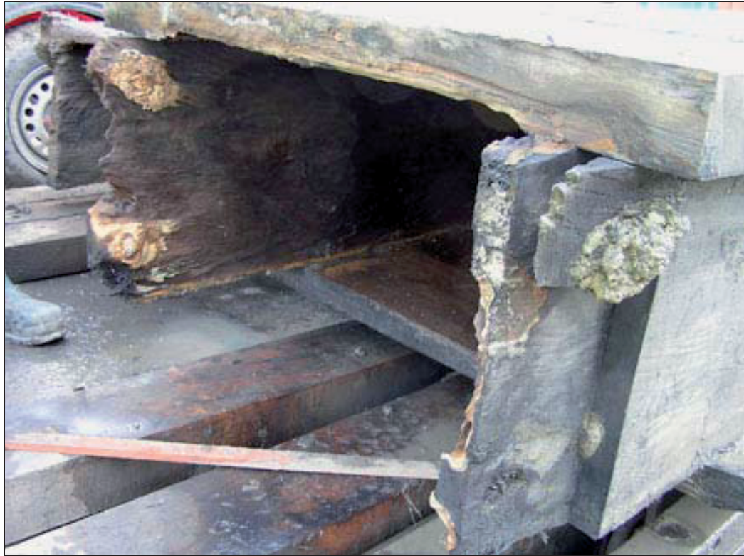
Plate 11 Construction detail of second section
