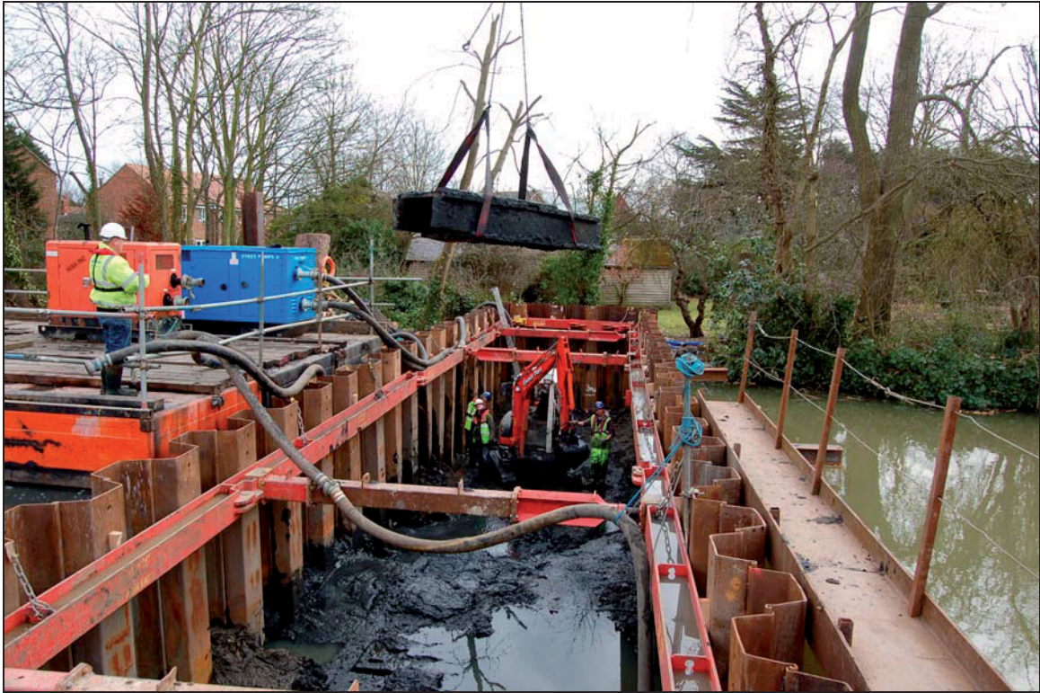
Plate 9 Chunker section being lifted onto pontoon
