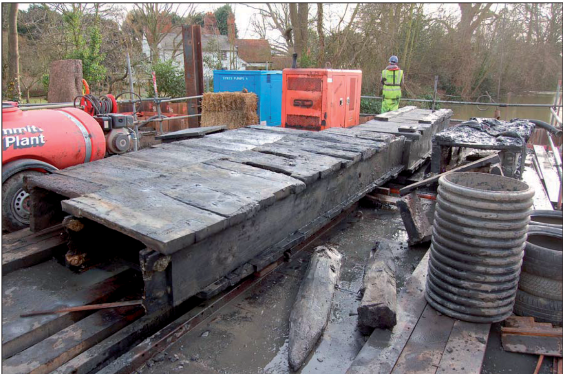
Plate 10 Chunker sections on pontoon
