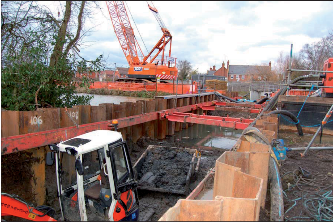
Plate 1 Excavation area viewed to north-west
