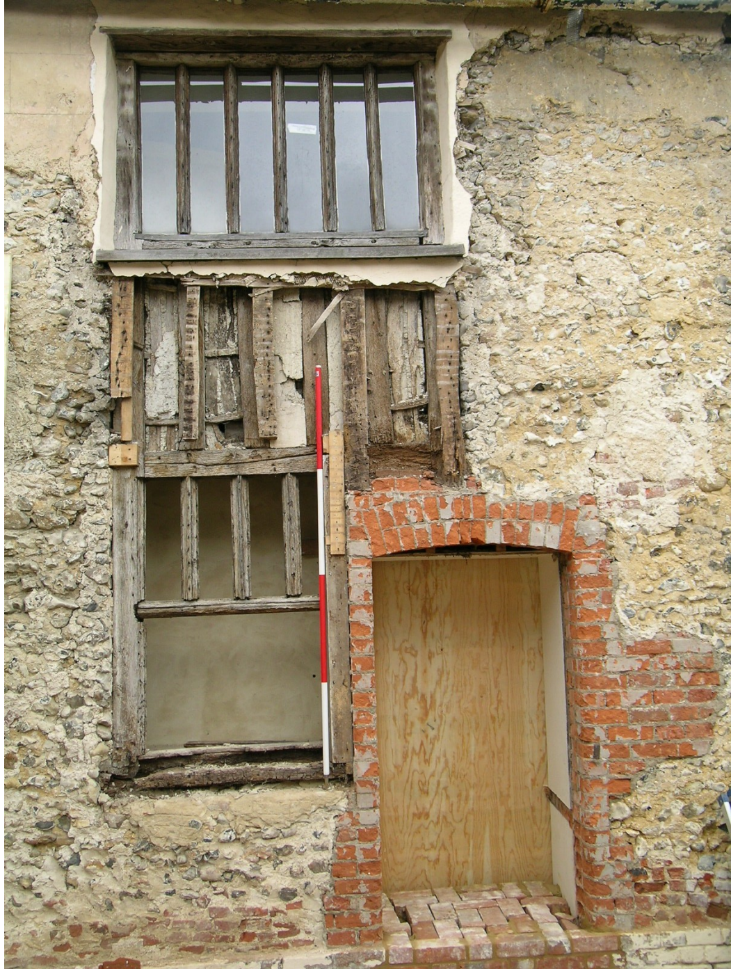
Plate 4 Mullion window (2m scale)
