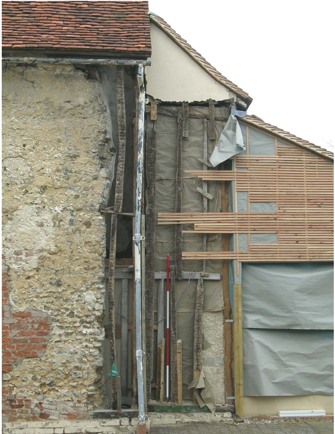
Plate 5 South-east corner of building (2m scale)
