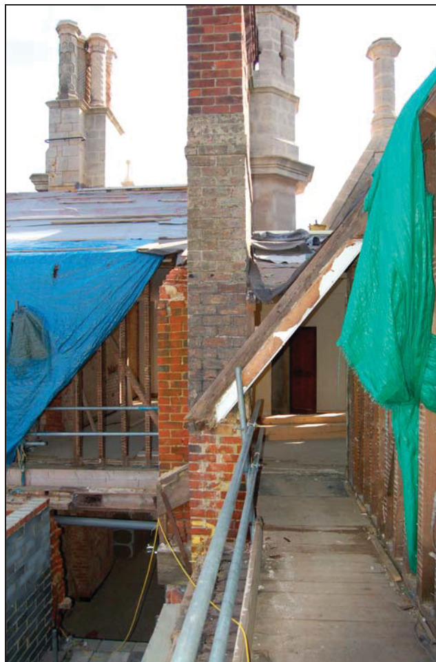
Plate 24 Second floor corridor viewed to south
