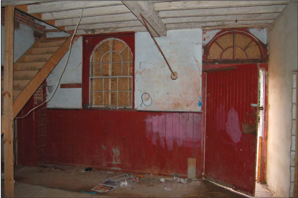
Plate 33 Original panelling and windows in main stable 2
