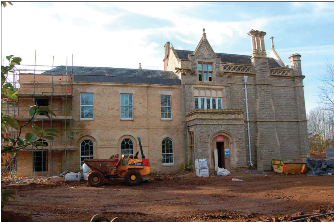
Plate 6 North elevation during survey
