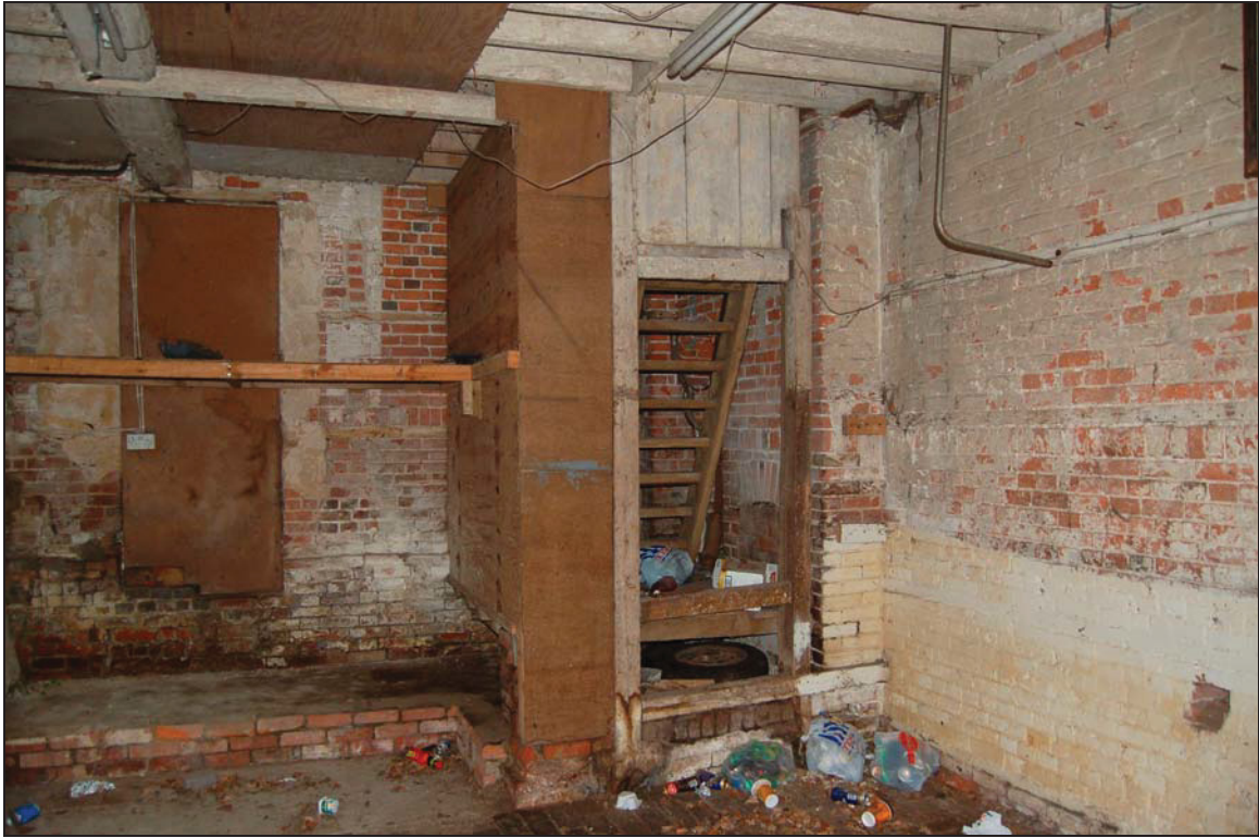
Plate 37 Former ?loose box in stable 3 viewed to east
