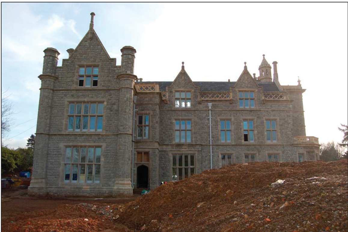
Plate 2 West elevation during survey
