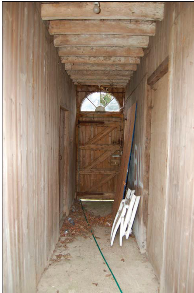
Plate 36 Passage in stable 3 viewed to yard (west)
