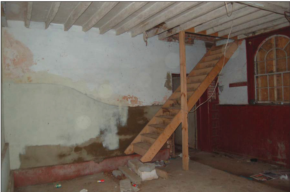
Plate 34 Outline of former stall on dividing wall to stable extension (south)
