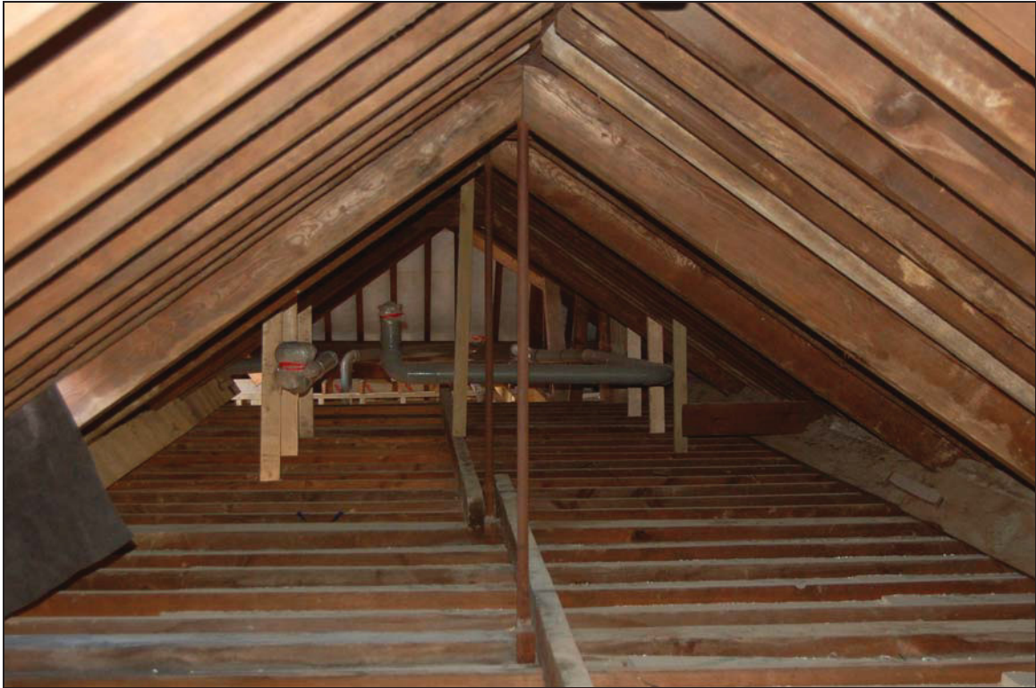
Plate 27 Roof construction over south wing
