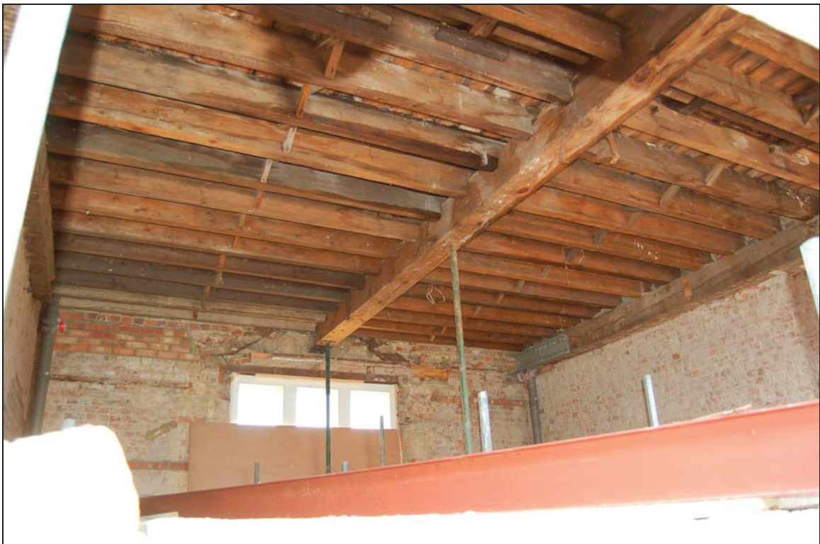
Plate 22 18th century ceiling on first floor over stair hall
