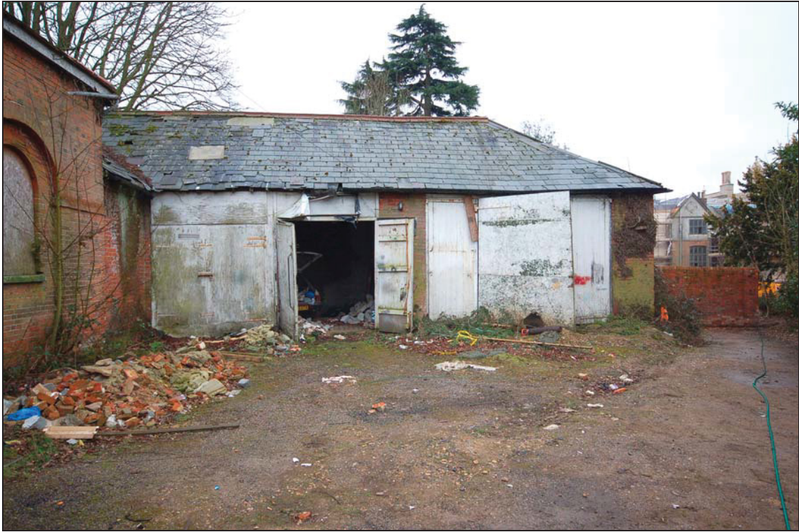
Plate 43 South wing of stable block (6): north elevation
