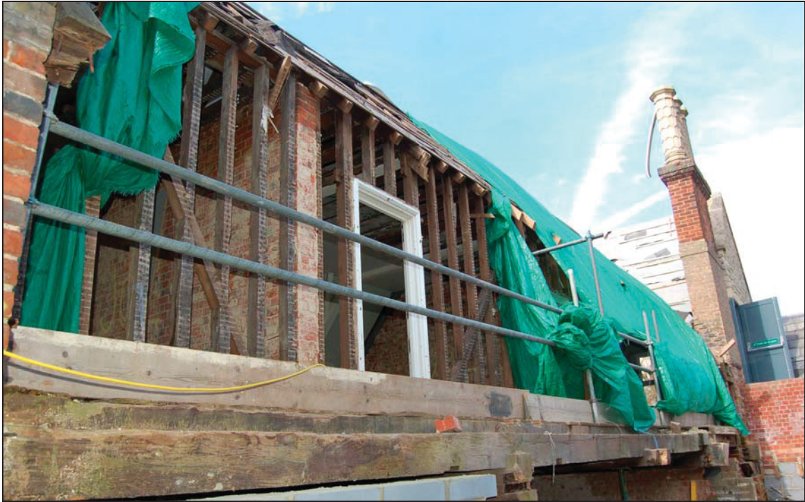
Plate 23 Second floor over west wing (1870) viewed to north-west
