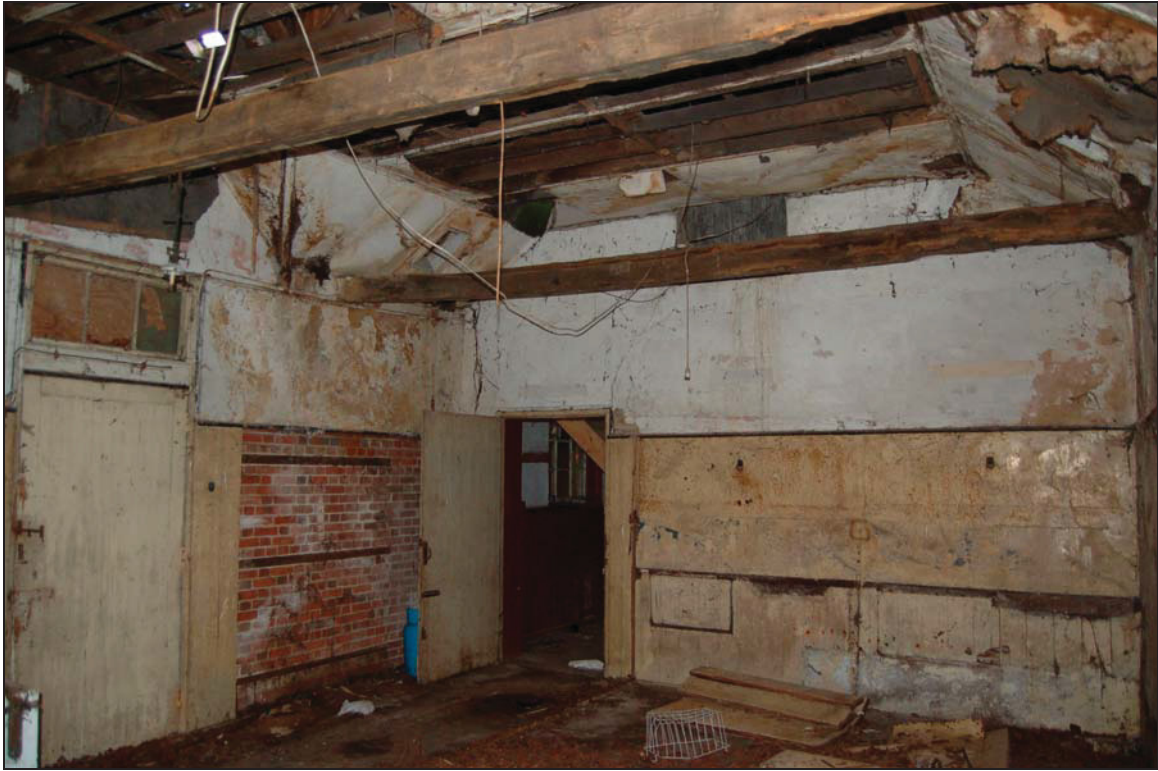
Plate 45 Interior of late 19th century stable extension
