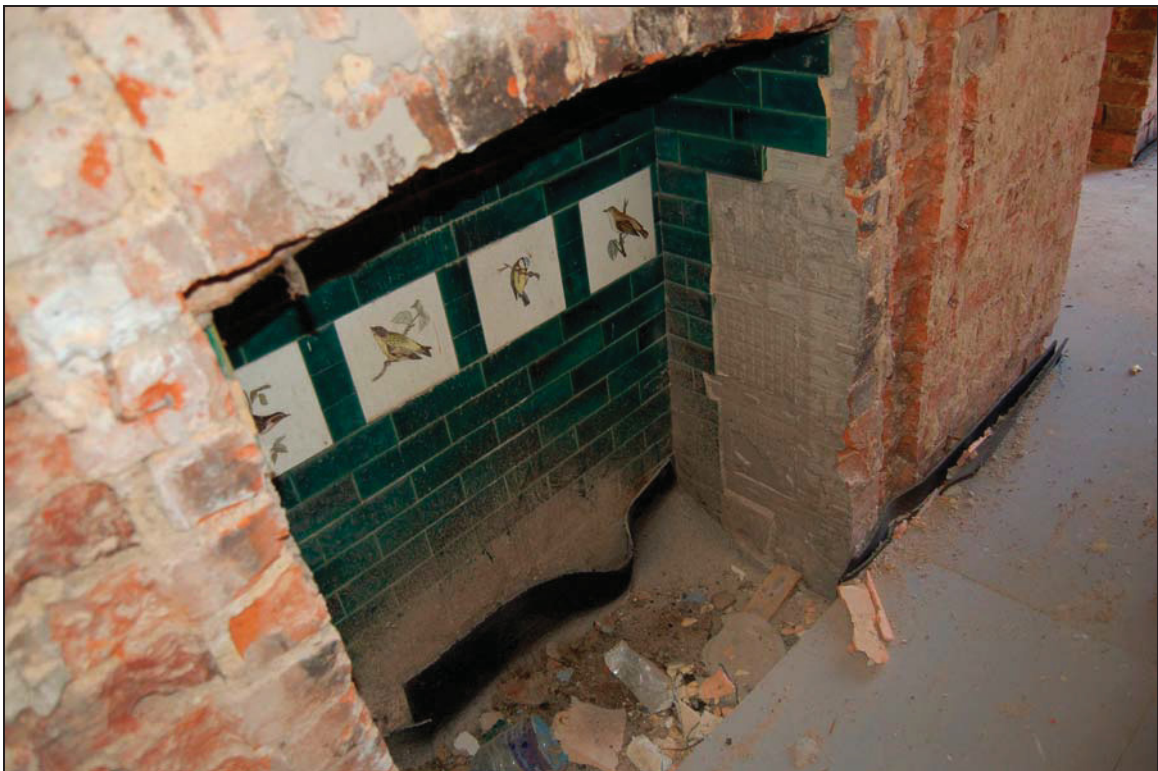
Plate 26 Tiled fireback in second floor bedroom
