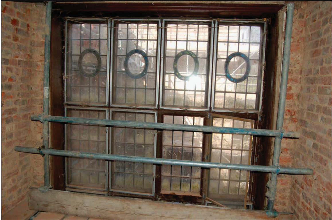
Plate 9 Detail of first floor window of stair tower
