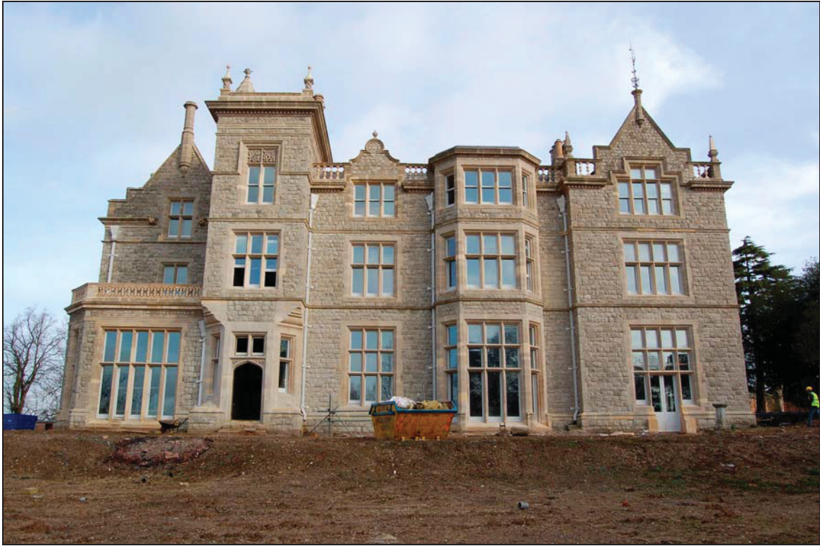
Plate 5 South elevation during survey
