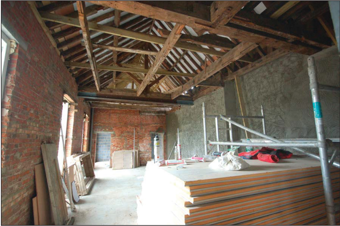
Plate 21 18th century roof in north wing
