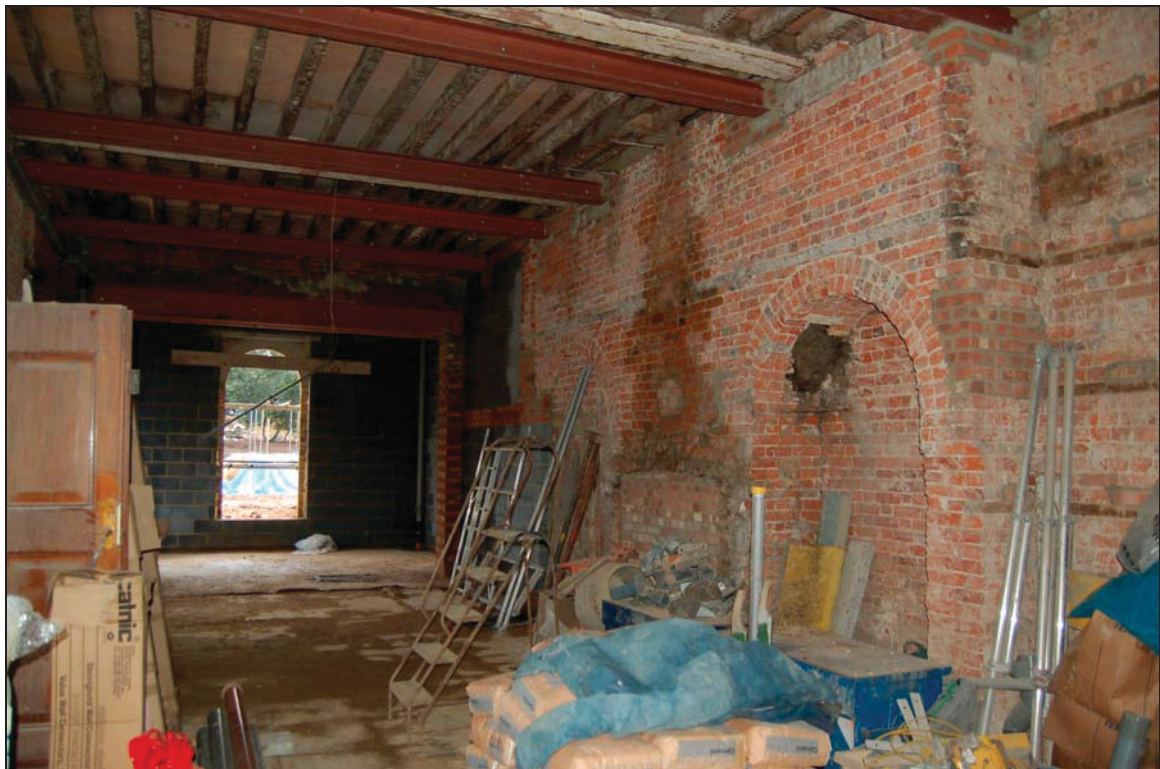
Plate 20 Kitchen/pantry in north wing during survey
