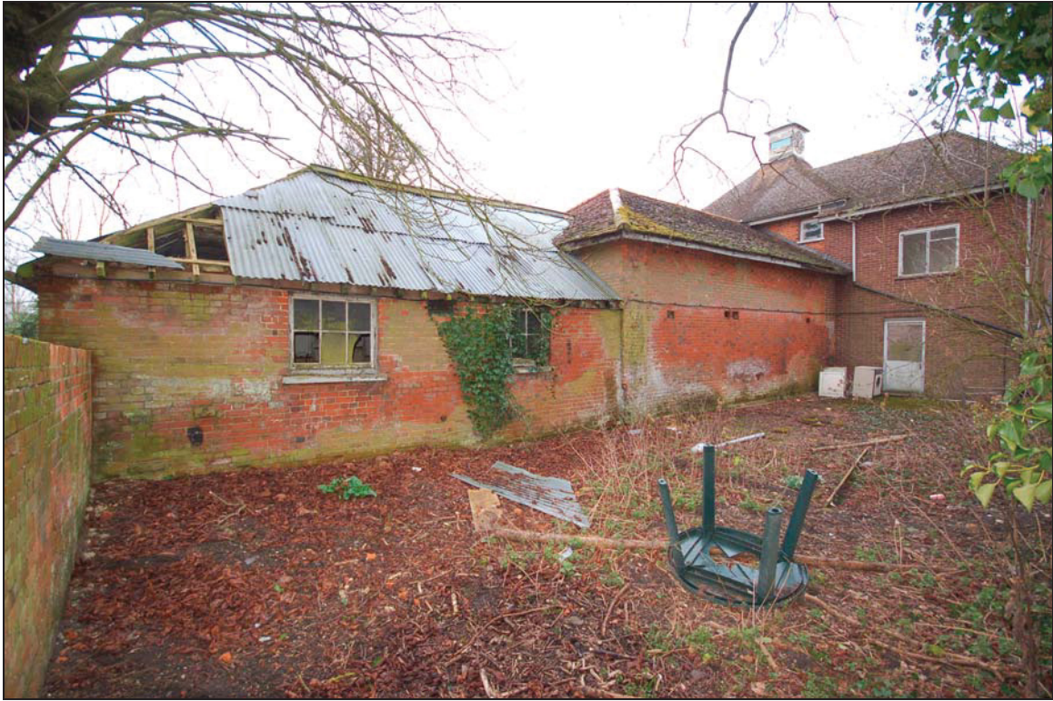
Plate 31 Stable block and house viewed from rear (north-west)
