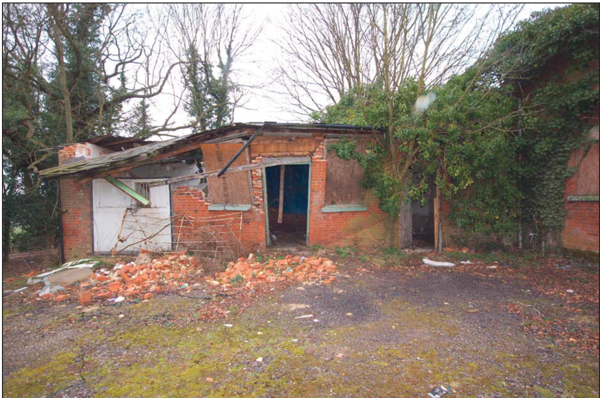
Plate 42 North wing of stable block (4): south elevation
