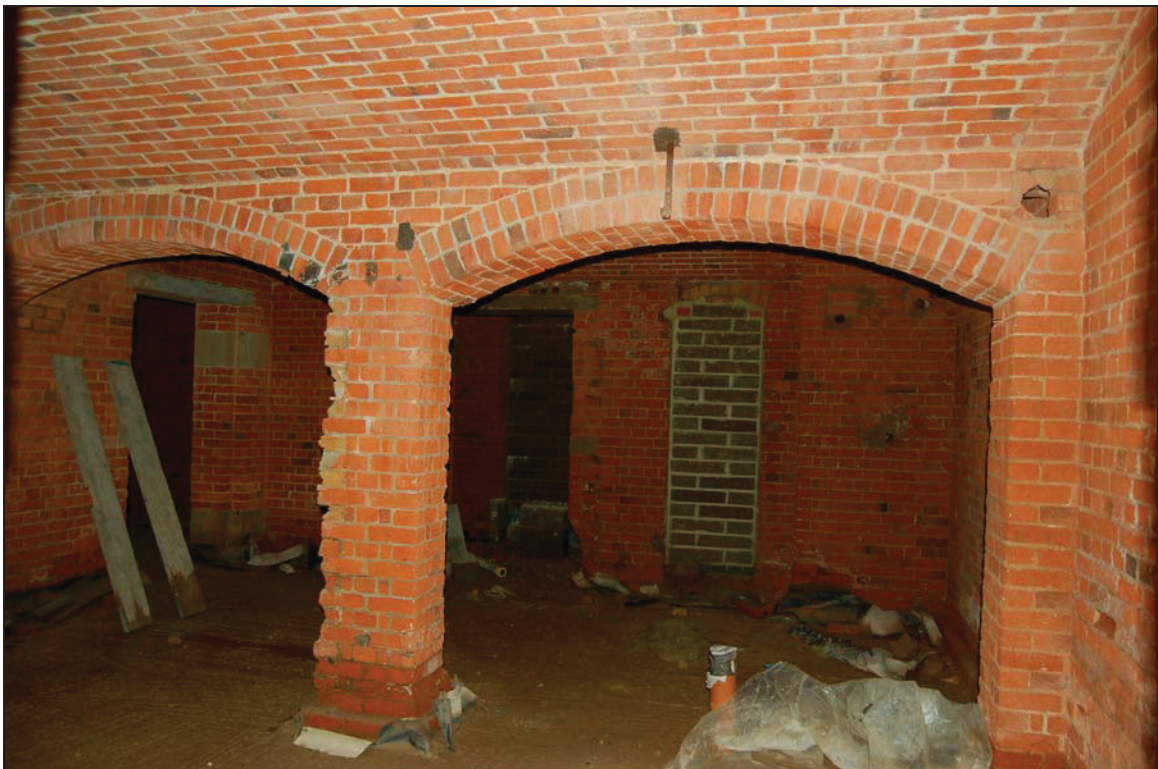
Plate 28 Basement viewed to north during survey
