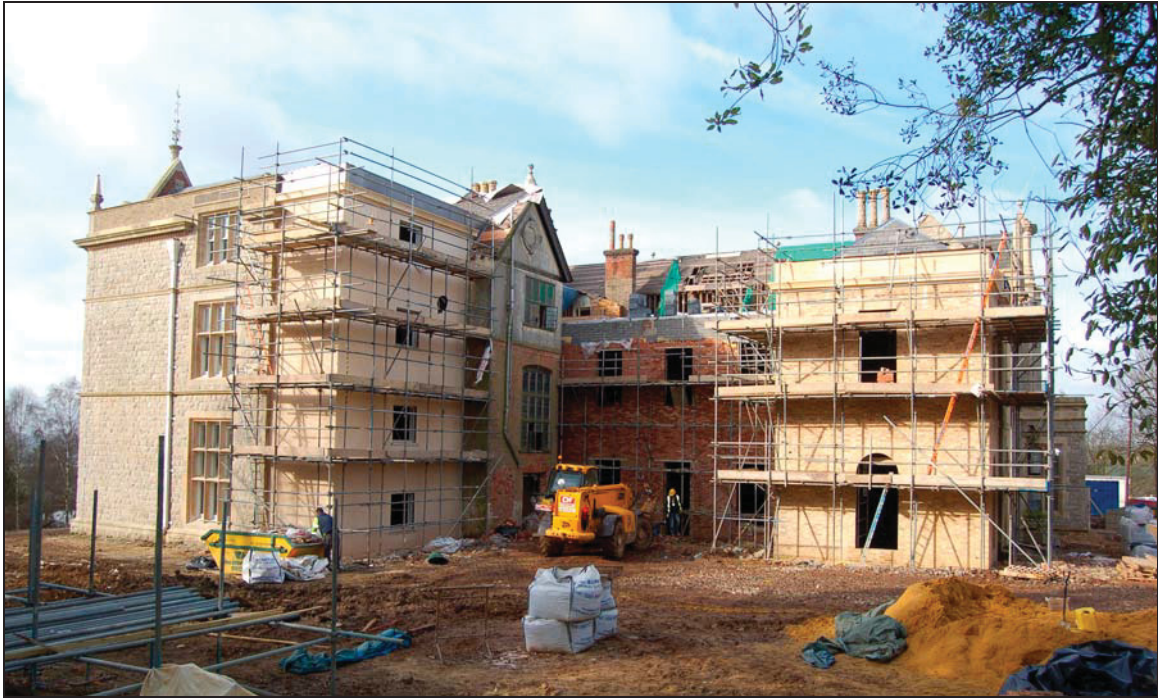
Plate 7 East elevation during survey
