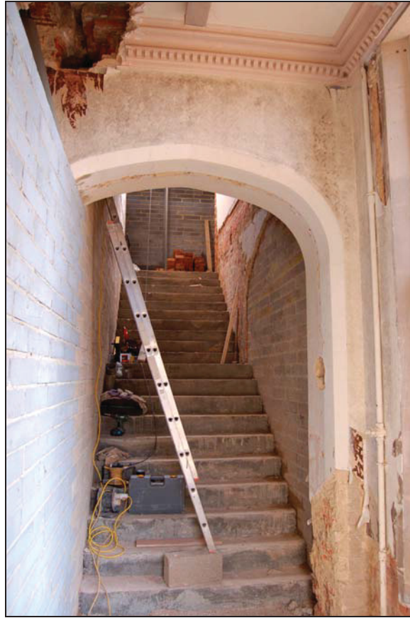
Plate 13 Décor remains in western porch and lobby area (inserted stair)
