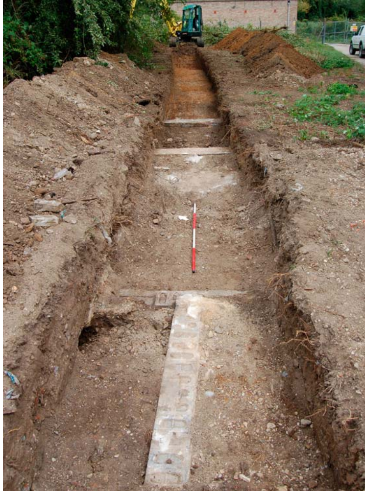
Plate 1. Walls and backfilled chambers (2m scale)
