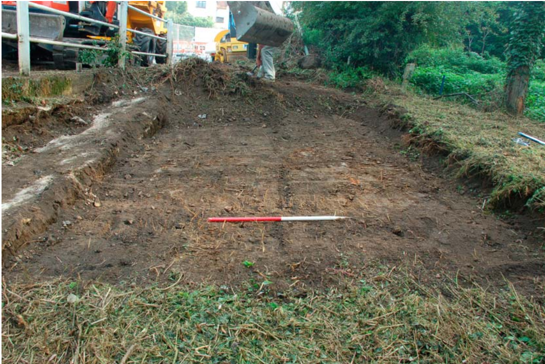
Plate 1. Northern bank stripped of topsoil. Looking north. 1m scale.
