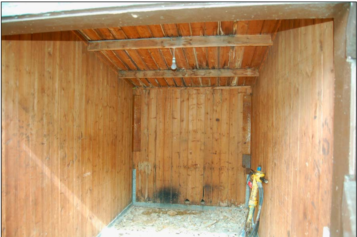
Plate 14 Interior of workshop
