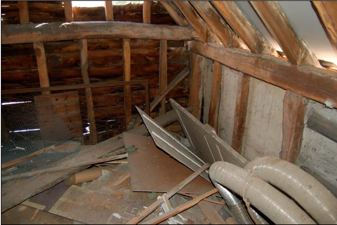
Plate 19 Infill panels and former pitching door on south wall
