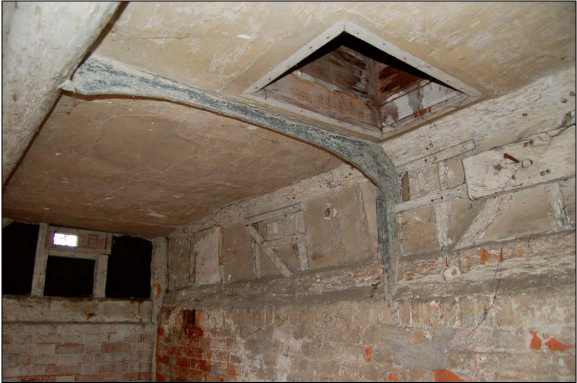
Plate 13 Carved timber and ceiling hatch
