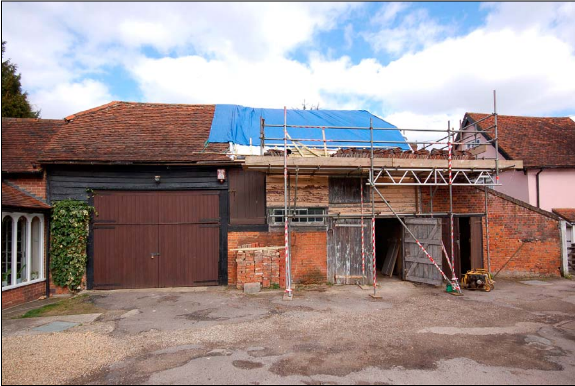
Plate 1 Front (south) elevation of barn
