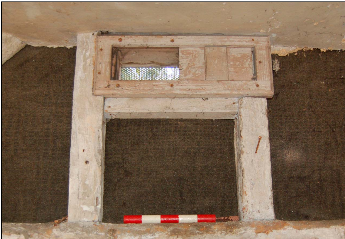
Plate 10 Detail of wooden vent on north wall
