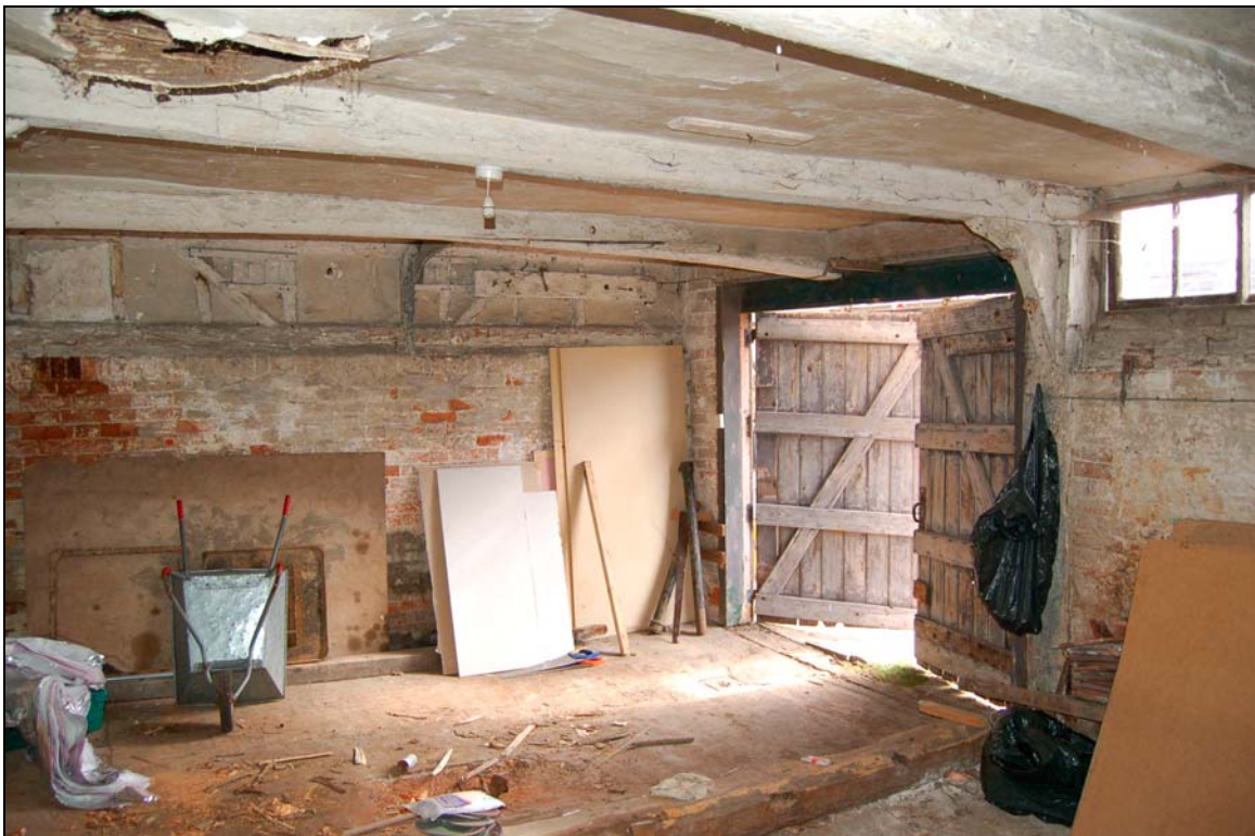
Plate 8 Interior viewed to south-east (cart doors)
