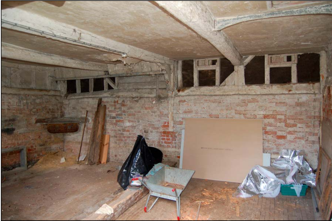
Plate 9 North wall and former partition
