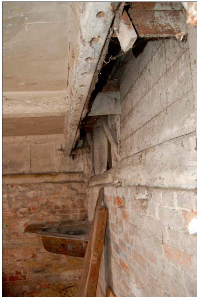
Plate 12 Removed hay feeder and hay chute on north wall
