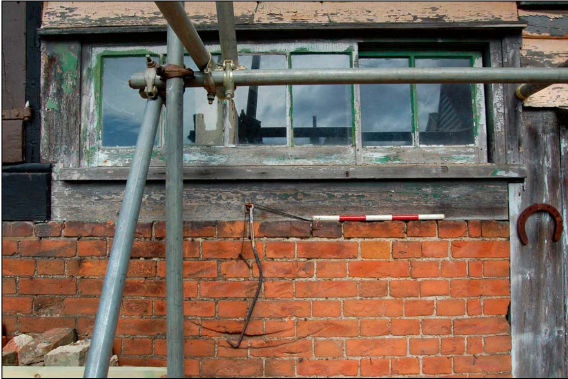
Plate 3 Horizontal sash window and cart door stay-rod
