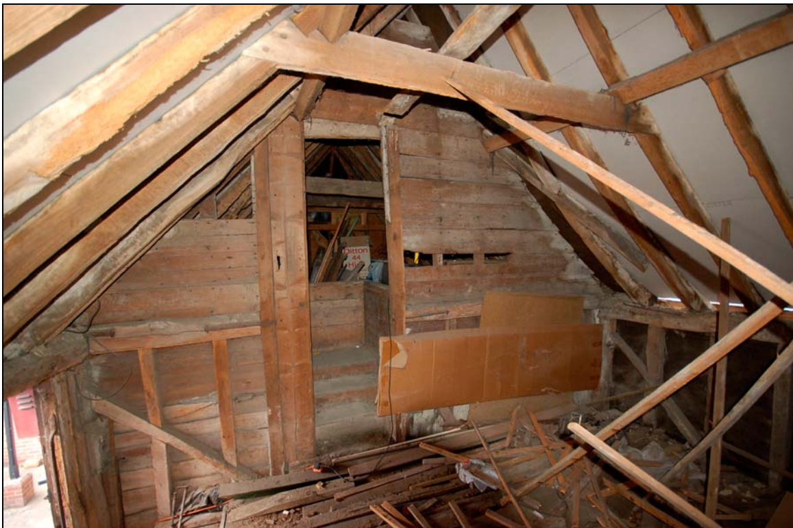
Plate 18 Partition wall between hay loft and feedstore
