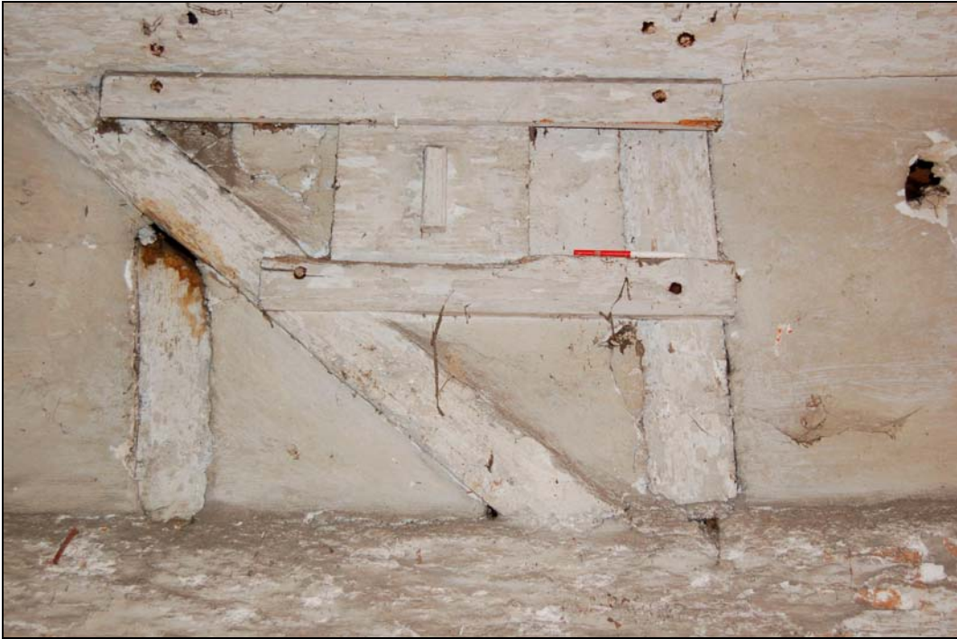
Plate 11 Detail of wooden vent on east wall
