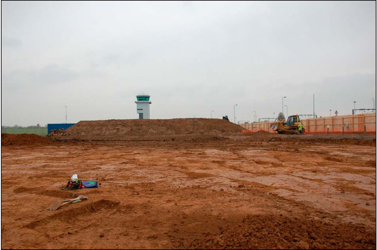
Plate 1. General view of Terminal area, looking north
