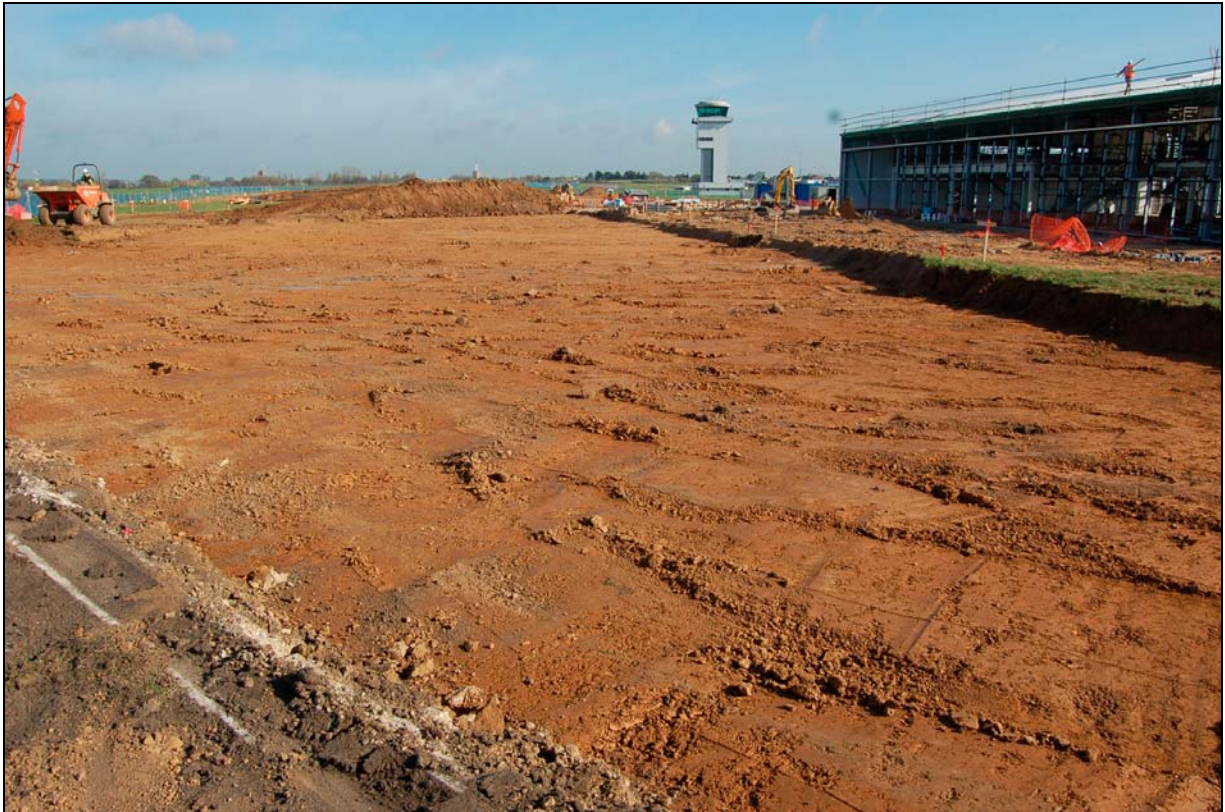
Plate 2. General view of south Apron area, looking north
