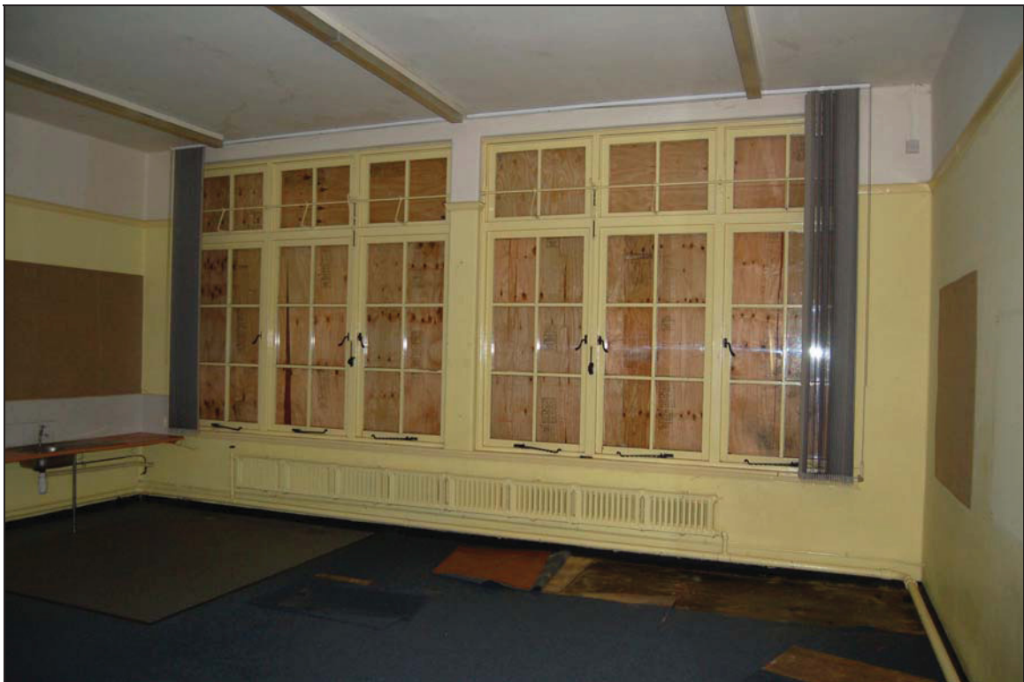
Plate 26 Windows in classroom 4
