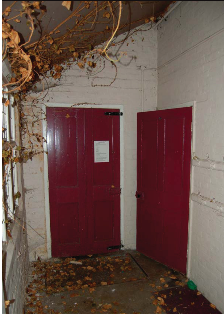
Plate 15 Entrance into boys lobby
