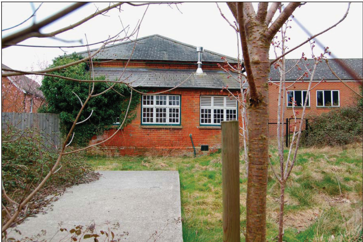
Plate 6 Former boys entrance lobby viewed to south
