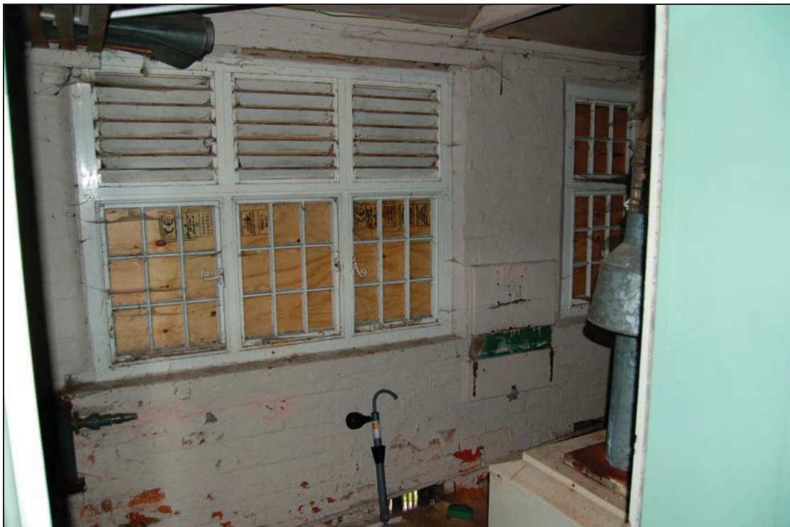
Plate 18 Interior of boiler room viewed to north
