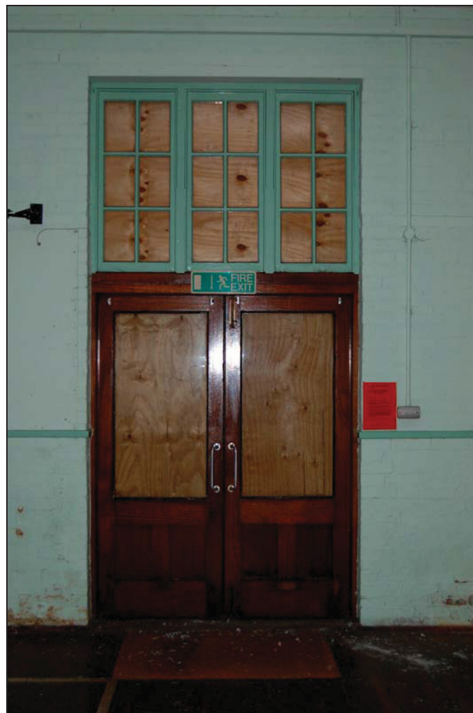
Plate 14 Inserted modern doors and window on western wall
