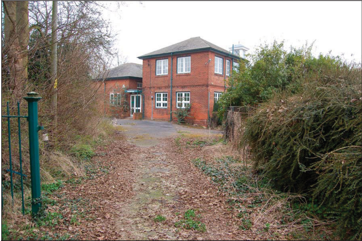
Plate 1 View of school from Rosemary Lane entrance (south-east)
