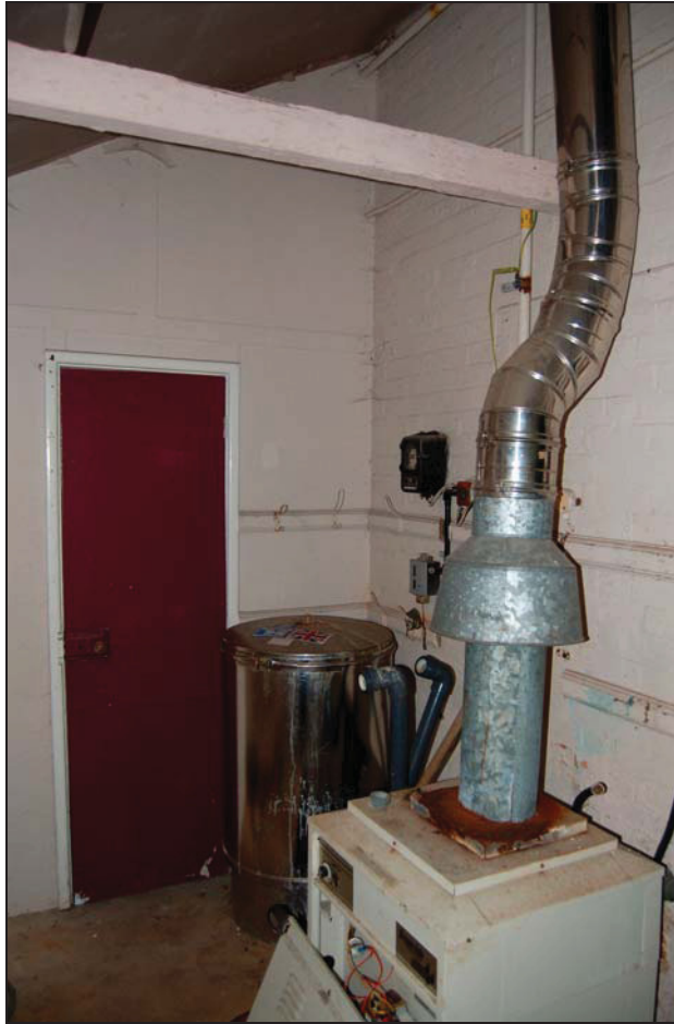
Plate 17 Interior of boiler room viewed to east
