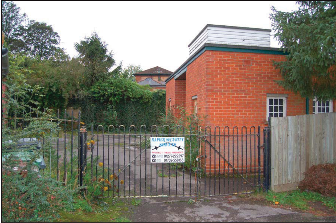
Plate 9 Kitchen extension next to side entrance
