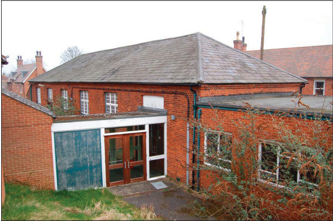
Plate 7 1844 School viewed to north-east with modern kitchen and link
