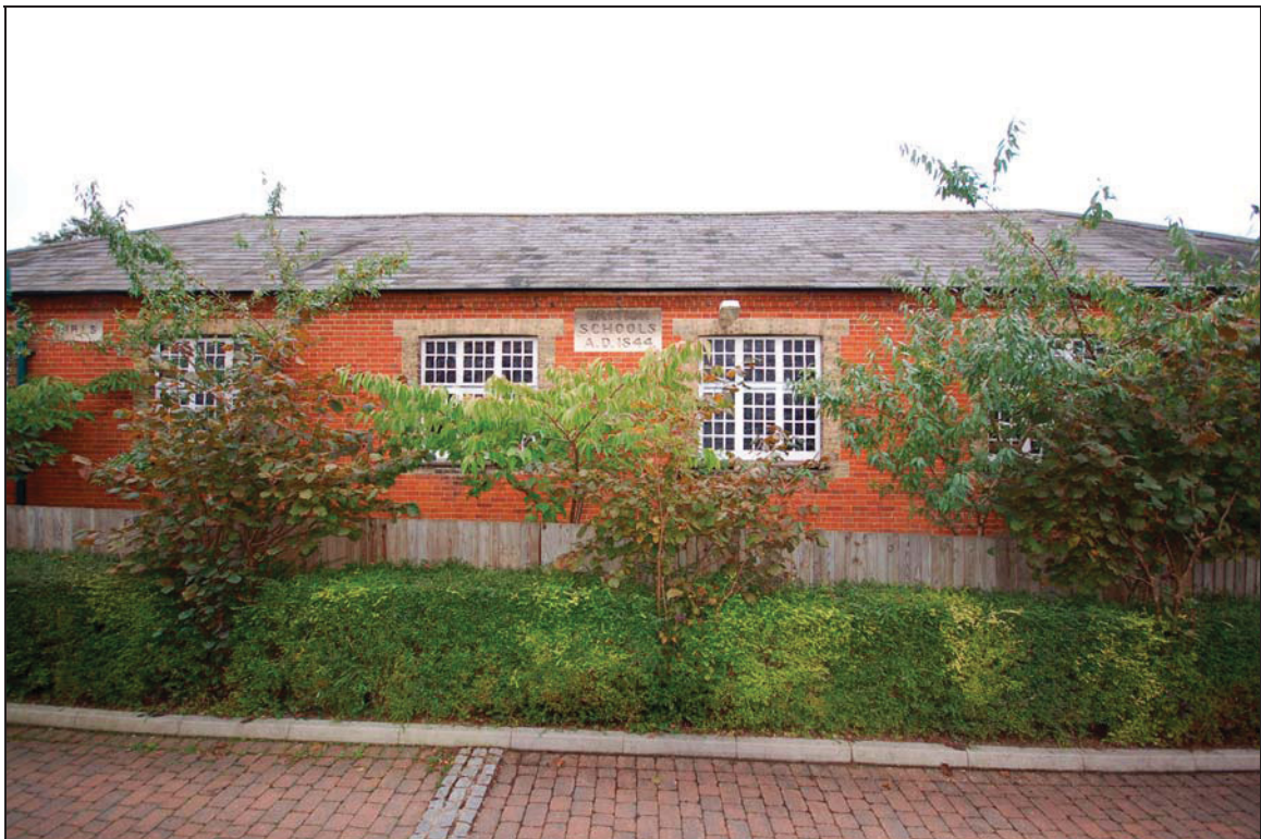
Plate 4 1844 School viewed to west
