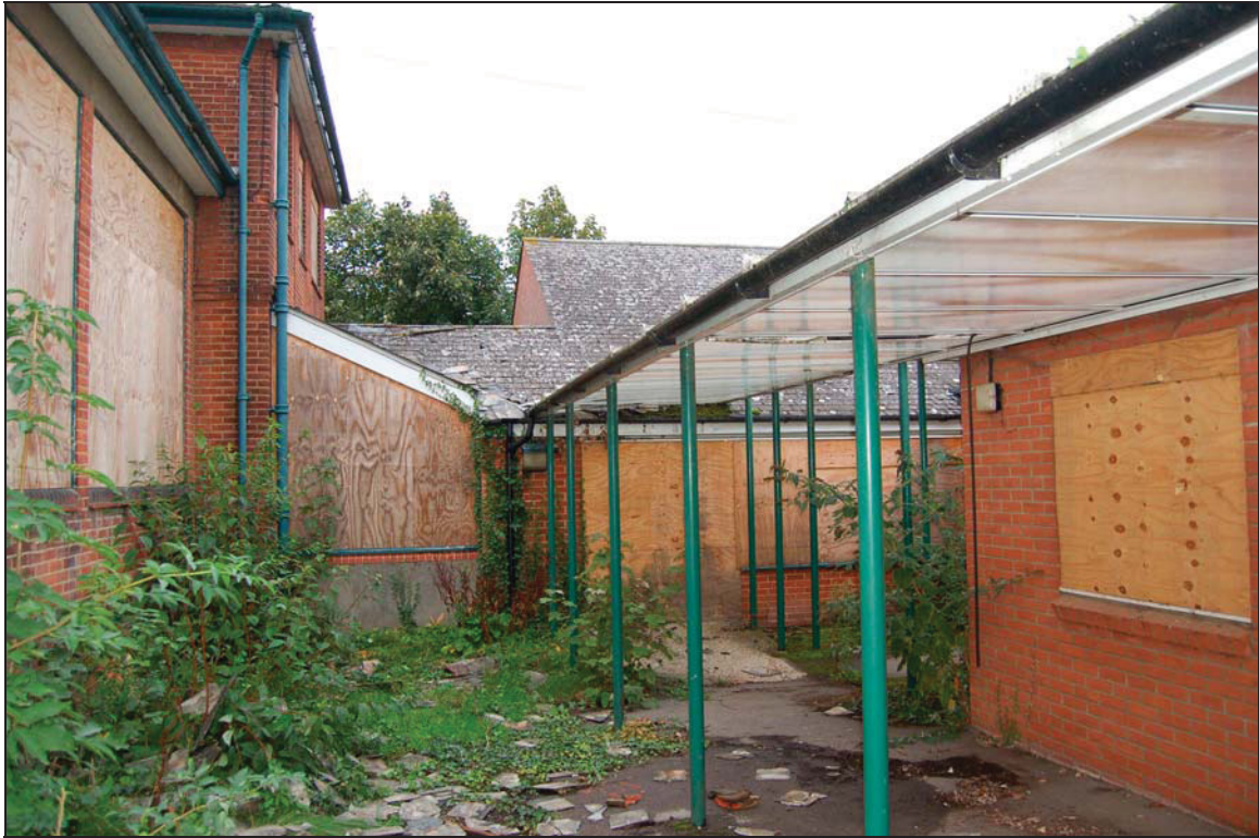
Plate 29 Covered area between 1958 school and modern additions
