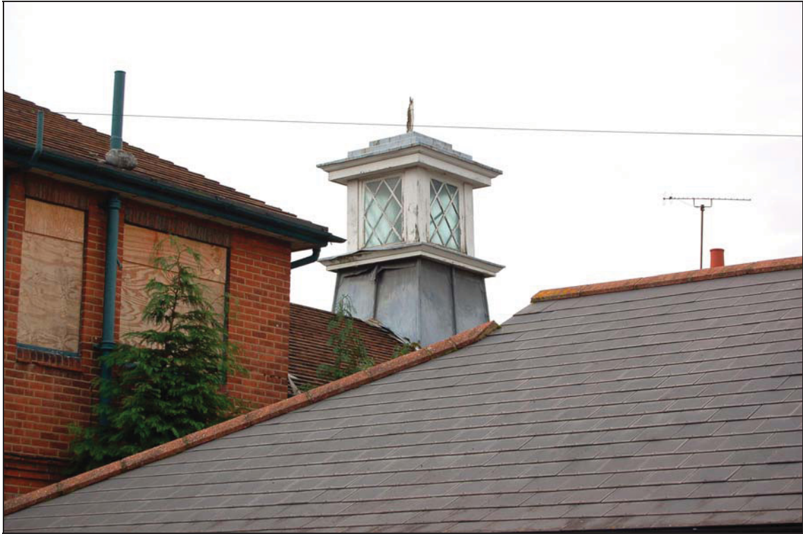
Plate 23 Roof lantern viewed to north-west
