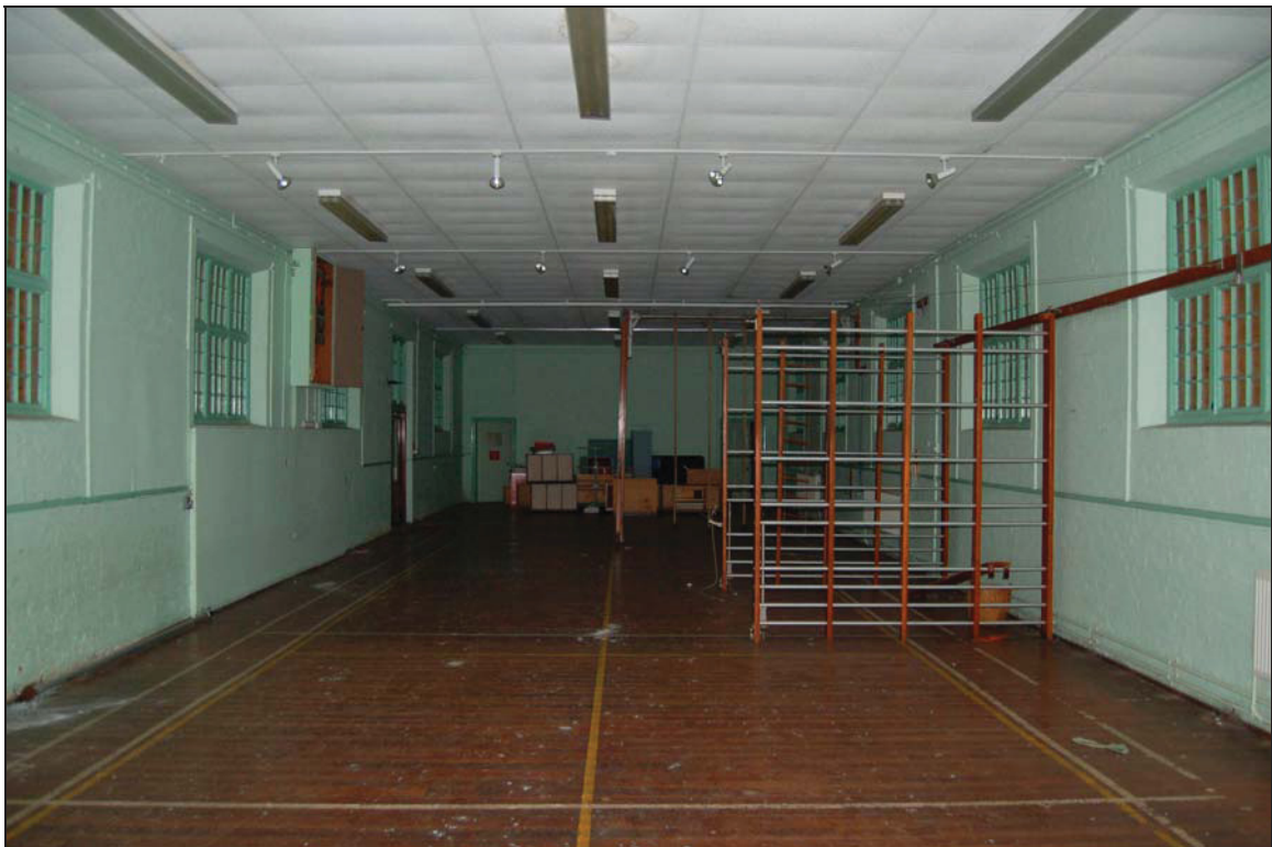
Plate 10 Interior of gym viewed to north
