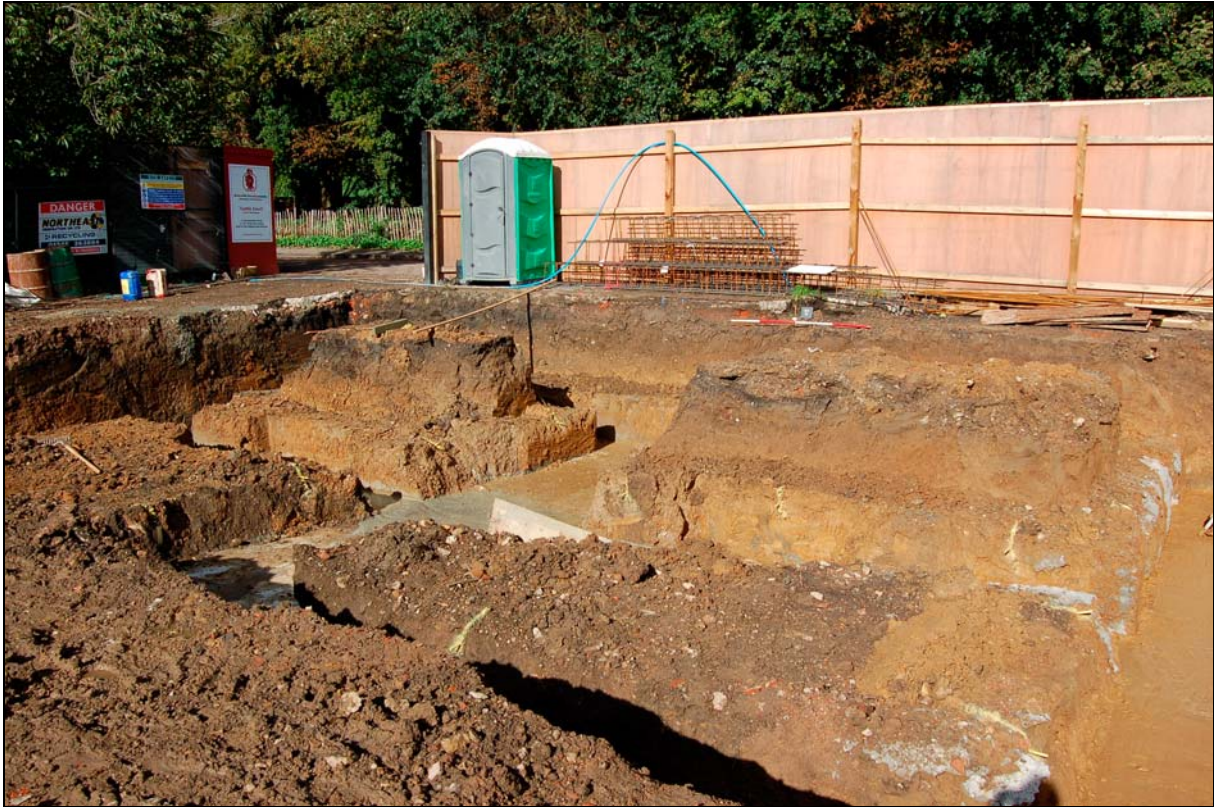
Plate 1 Monitored area viewed to north, showing sections 1 & 2
