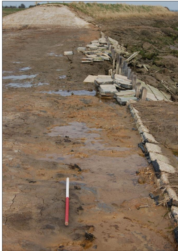
Plate 10. Detail of decayed stakes (1m scale)
