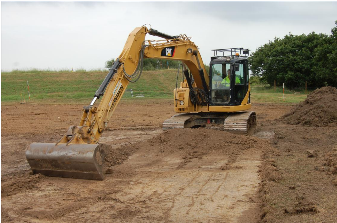
Plate 8. Topsoil stripping for Rigdons closure bank
