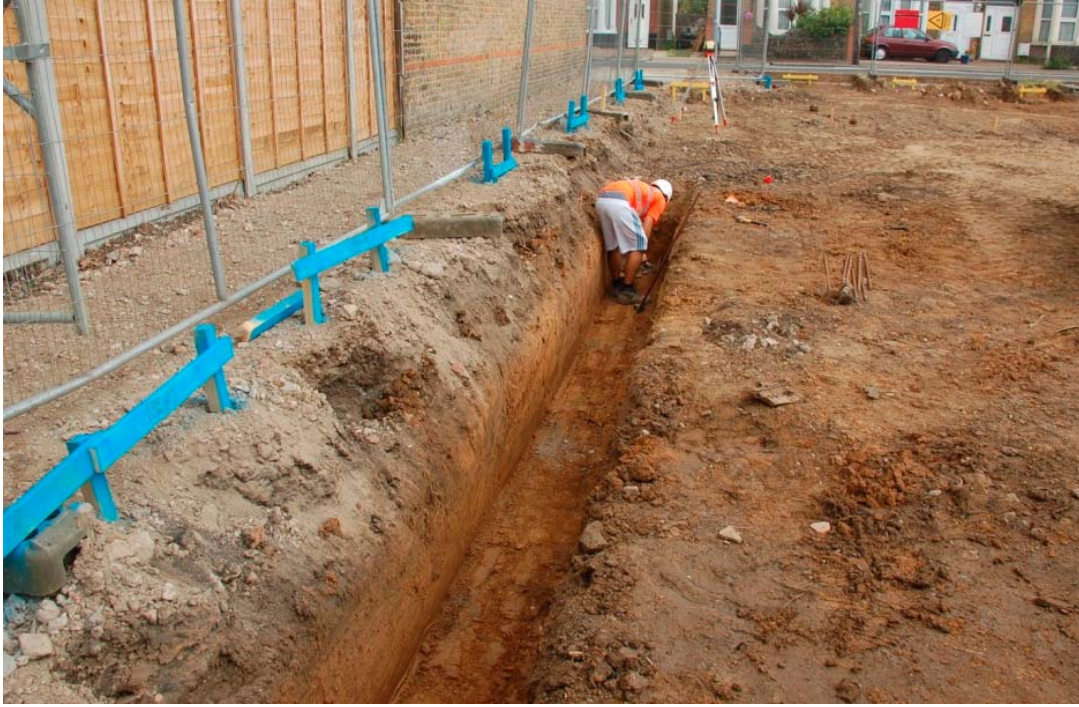
Plate 1. Foundation trench for new church looking east
