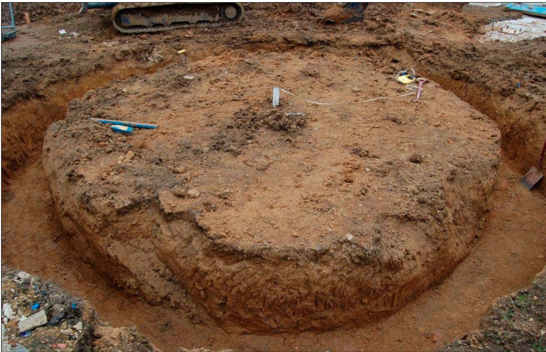
Plate 2. Circular foundation trench looking north-west
