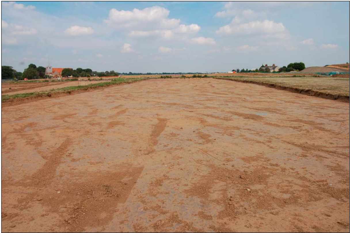
Plate 5. Runway extension topsoil strip, looking north-east
