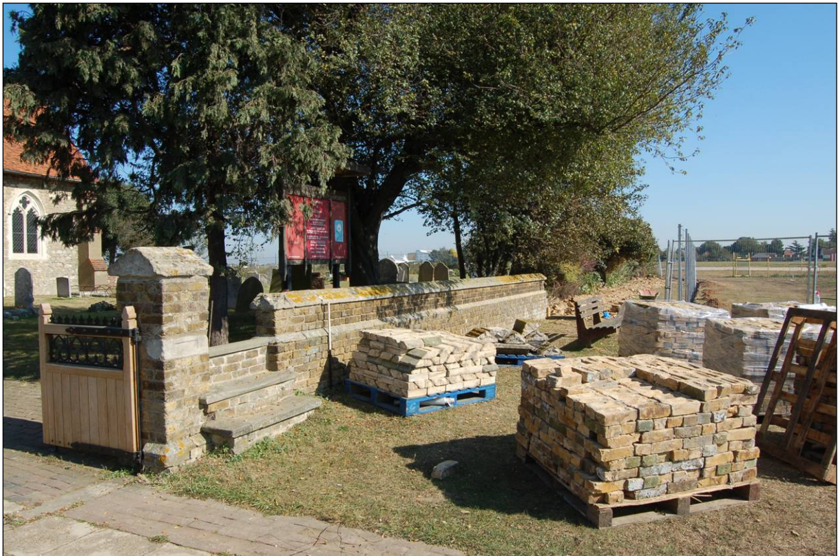
Plate 12. Churchyard wall, during removal works
