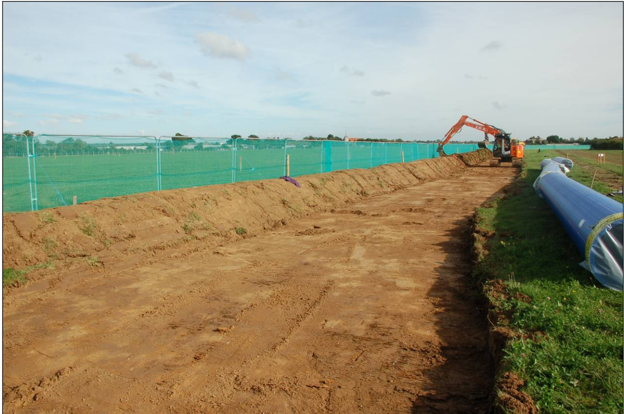
Plate 1. Easement strip for mains services diversion works, looking east
