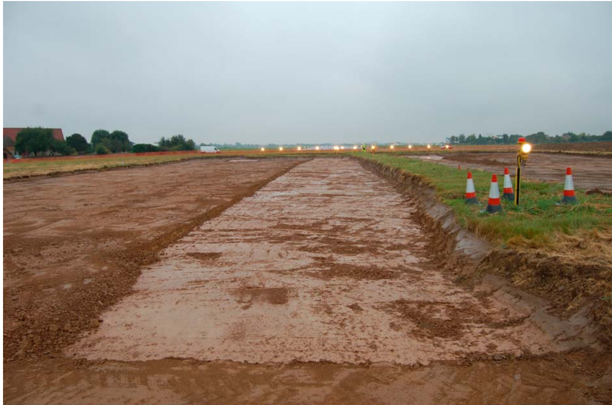
Plate 8. Deeper strip of Runway extension footprint
