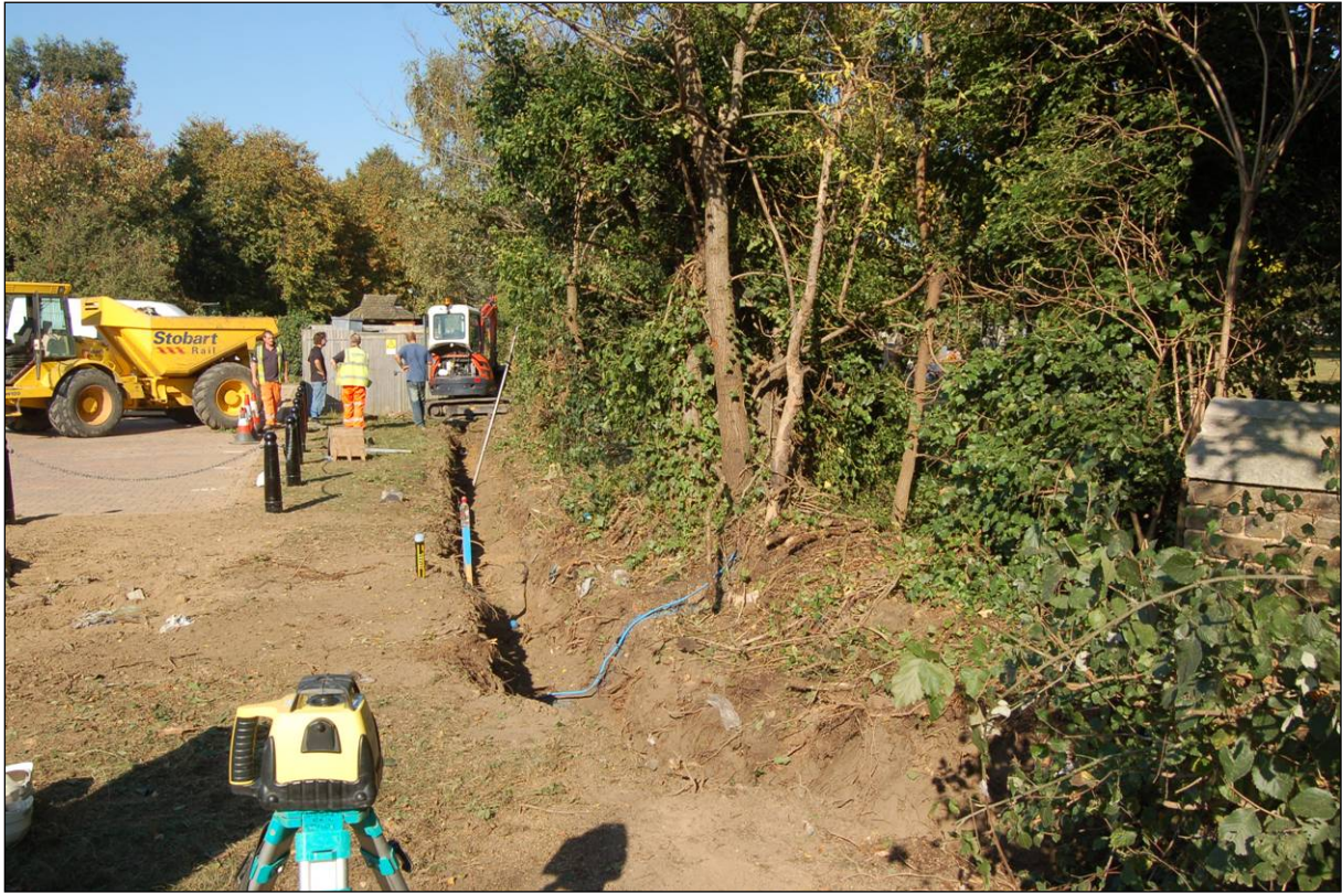
Plate 13. Foundation trench for new wall on west side of churchyard
