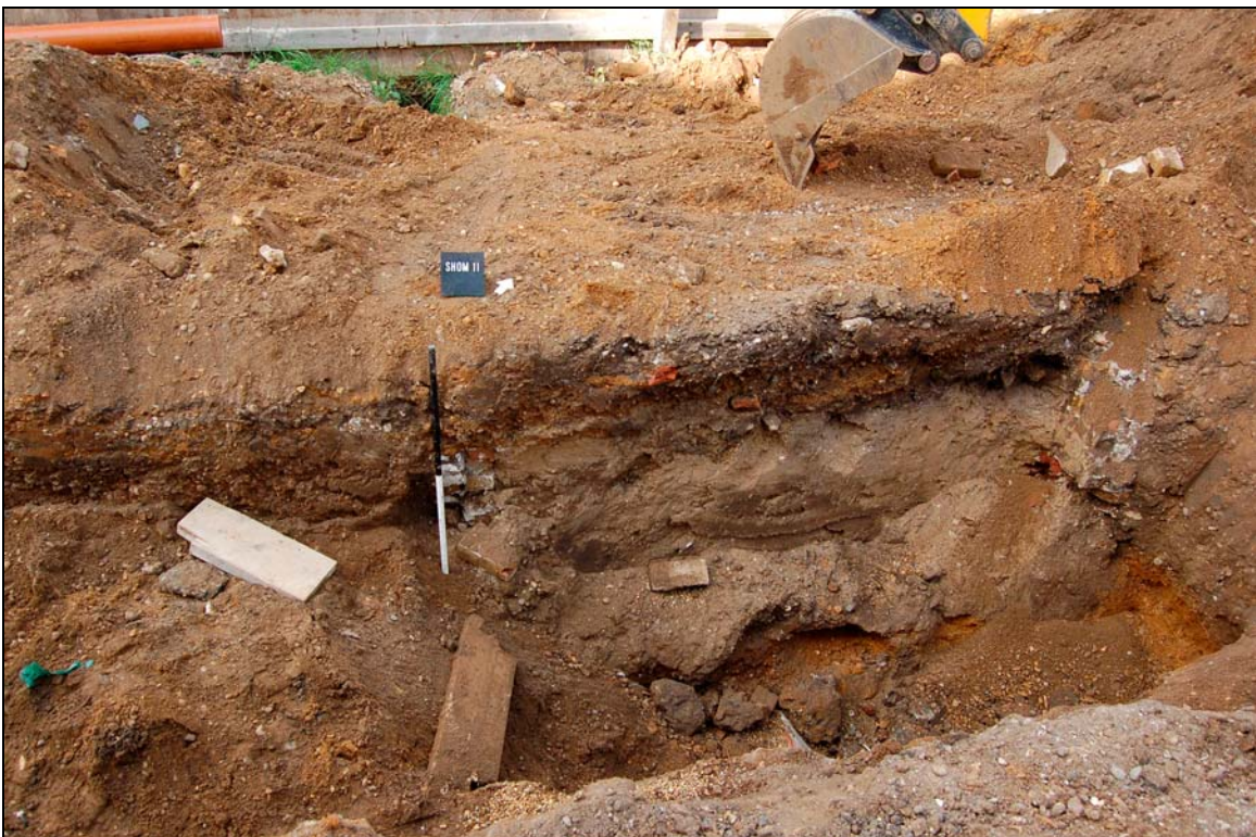
Plate 4. Large 'bunker' viewed at south-west end of storm drain trench
