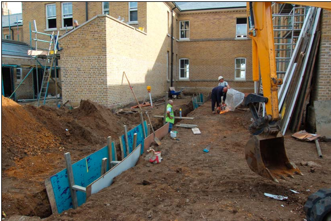
Plate 6. Boundary wall trench between plots 7 and 8
