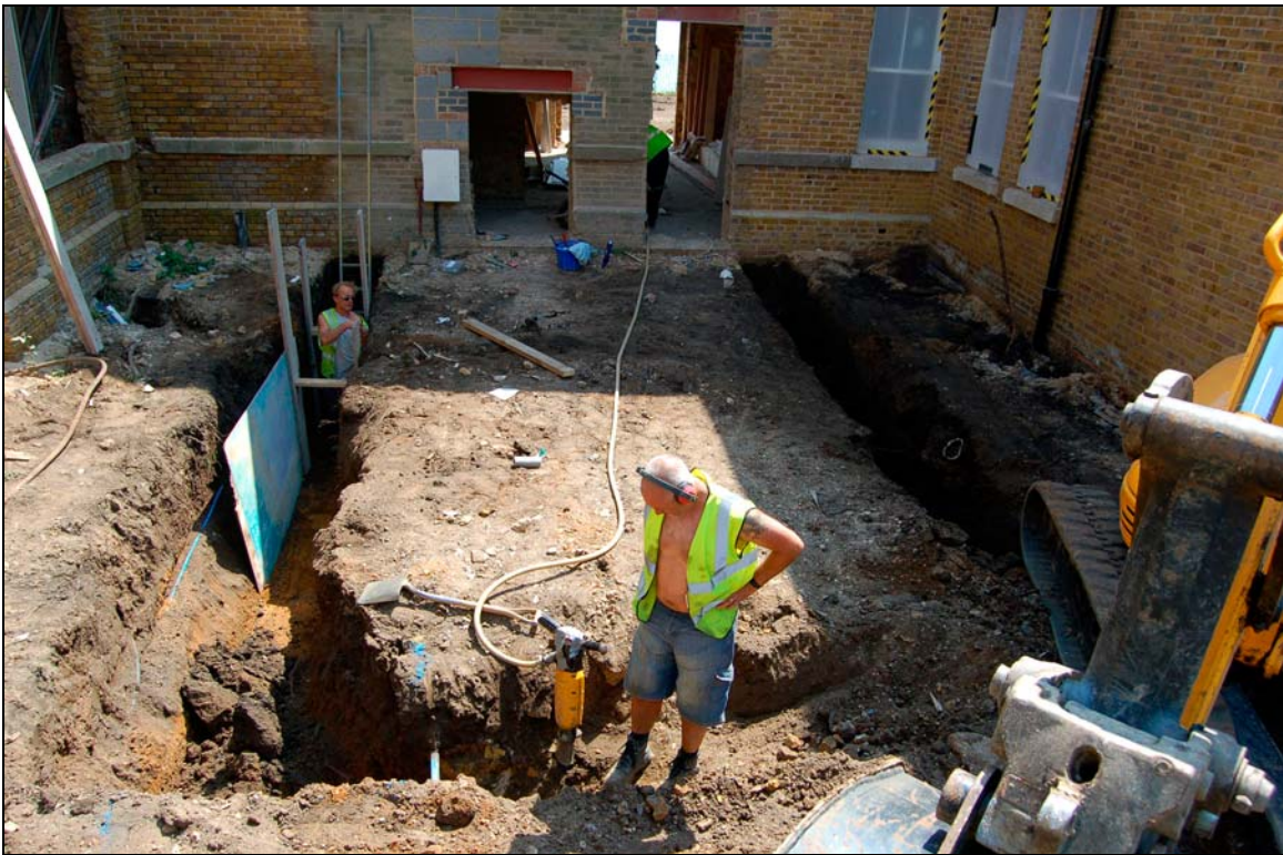
Plate 2. Excavation of plot 10 extension, viewed to south-east
