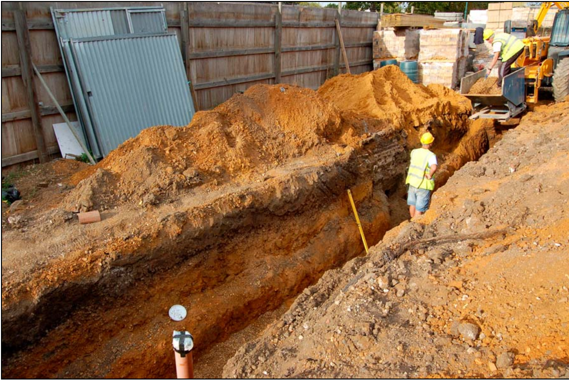
Plate 3. Excavation of storm drain trench, viewed to north-east
