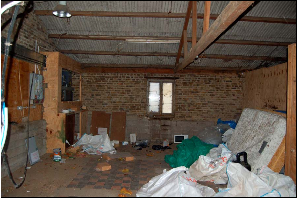
Plate 7 Interior of building 2
