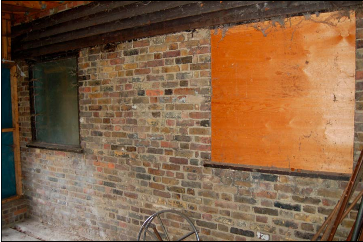
Plate 9 Detail of brickwork of building 3
