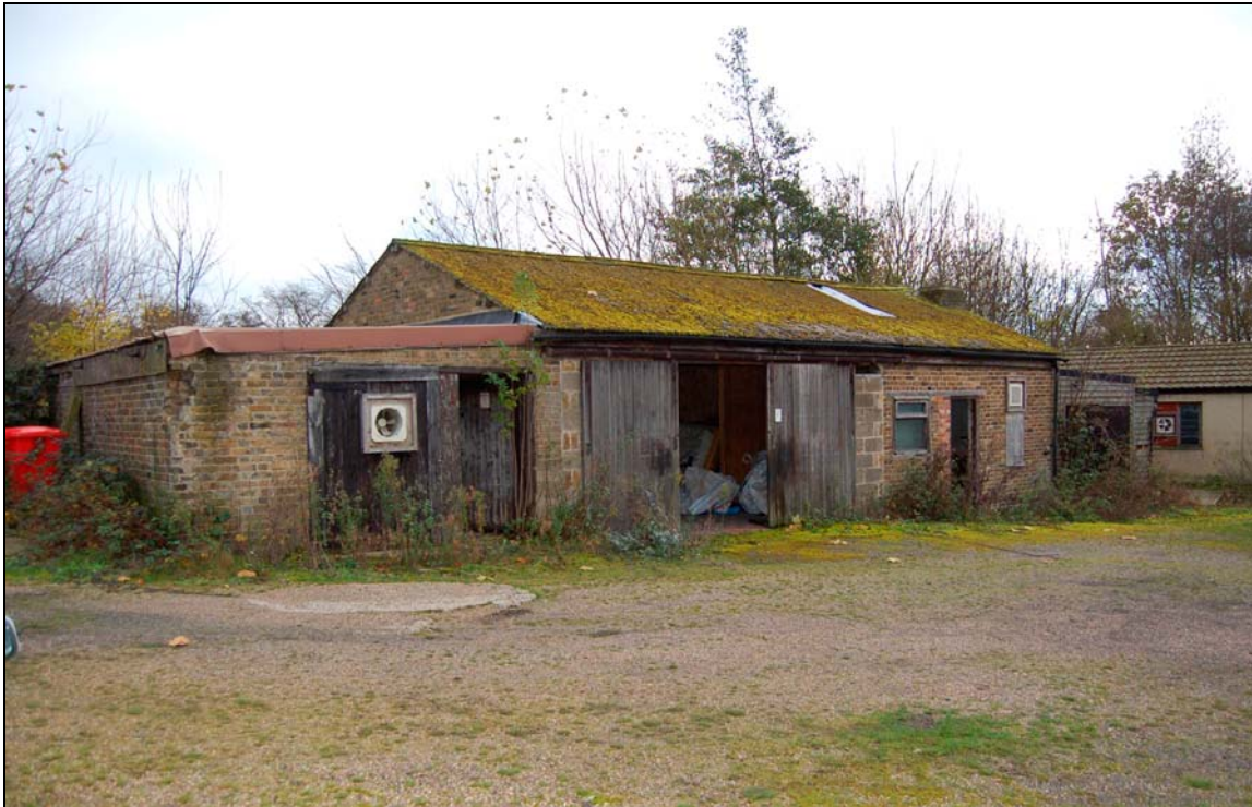
Plate 6 Building 2 viewed to east
