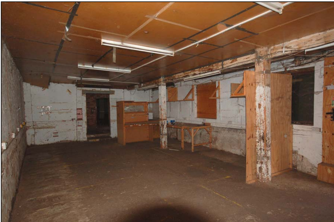
Plate 10 Interior of building 3 viewed to north
