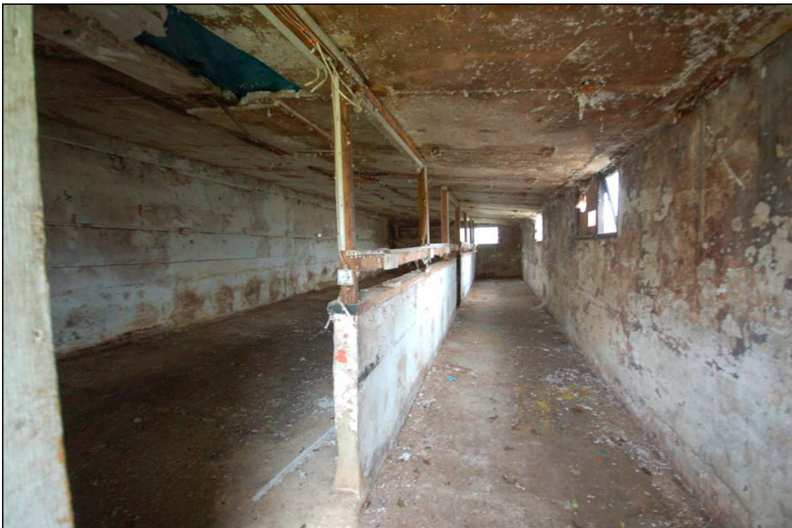
Plate 14 Interior of dairy lean-to viewed to east
