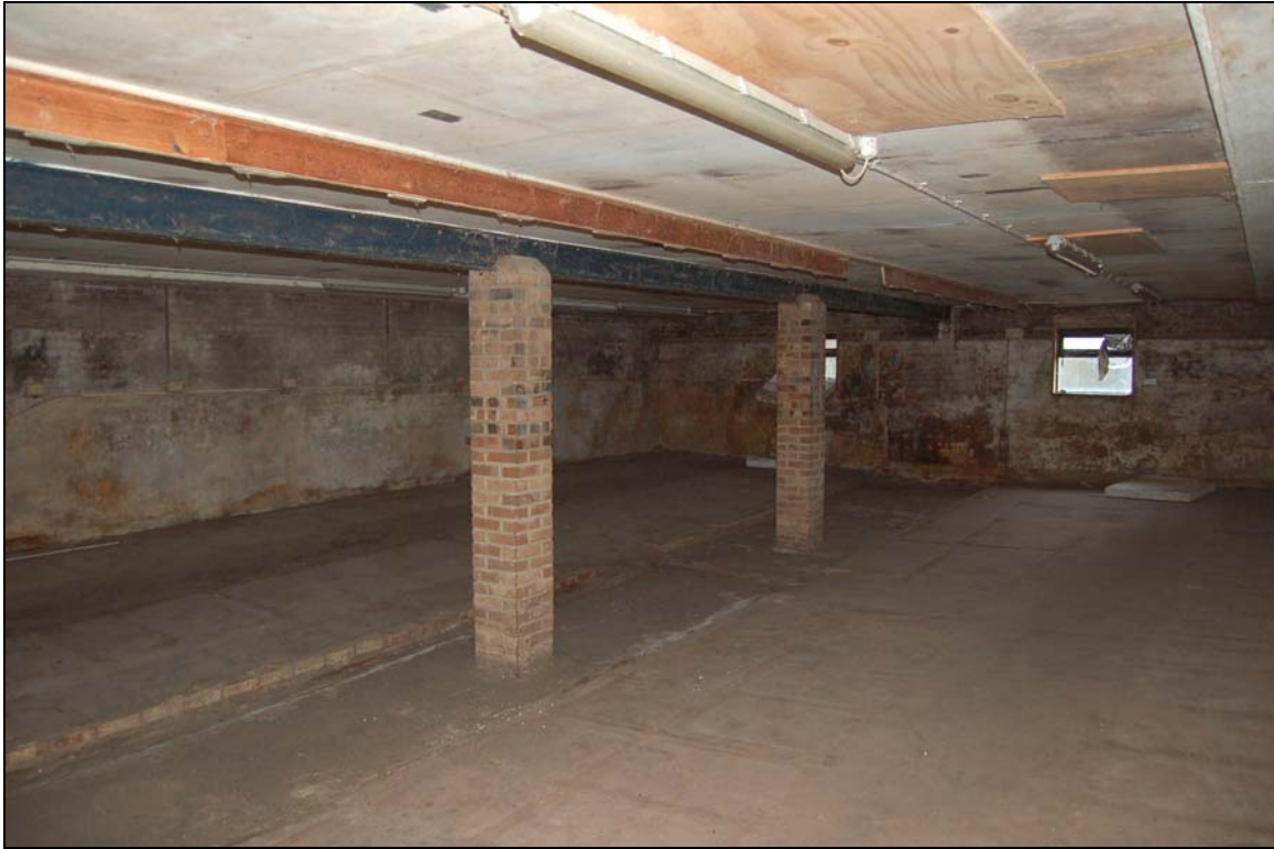
Plate 13 Interior of dairy viewed to north-east
