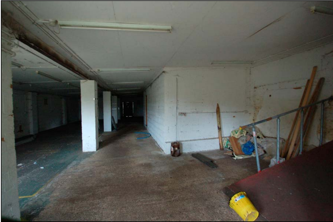
Plate 15 Interior of modern warehouse viewed to north
