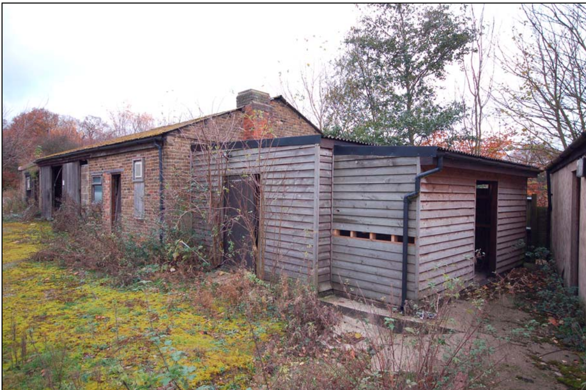
Plate 16 Typical modern shed, attached to building 2
