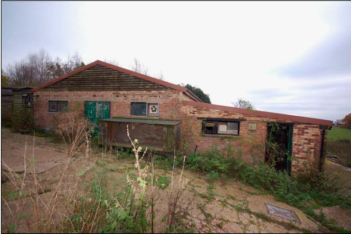
Plate 11 Dairy building 4 viewed to east
