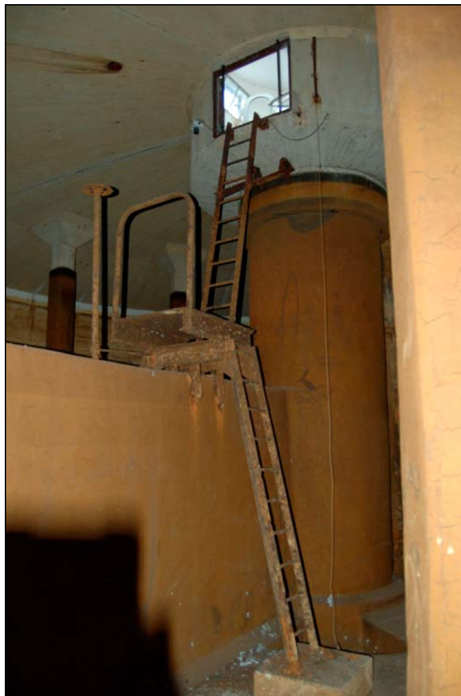
Plate 12 View of doorway into tank and platform
