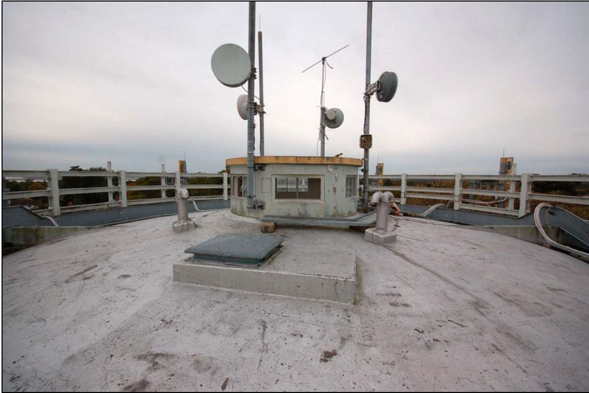
Plate 3 Roof of water tower
