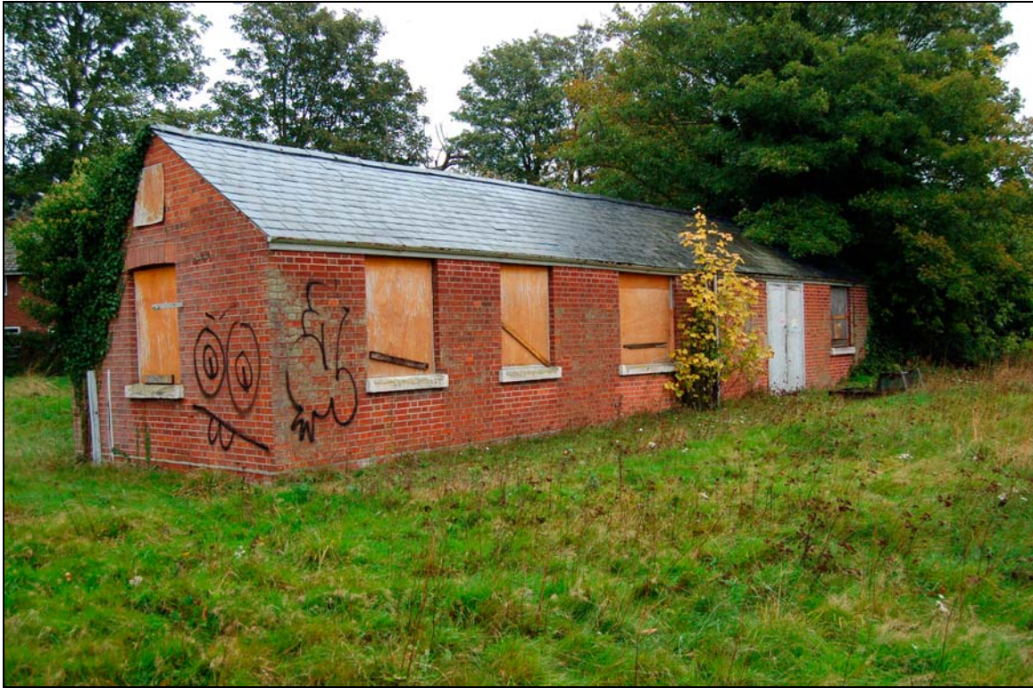
Plate 15 Pump house viewed to north-east
