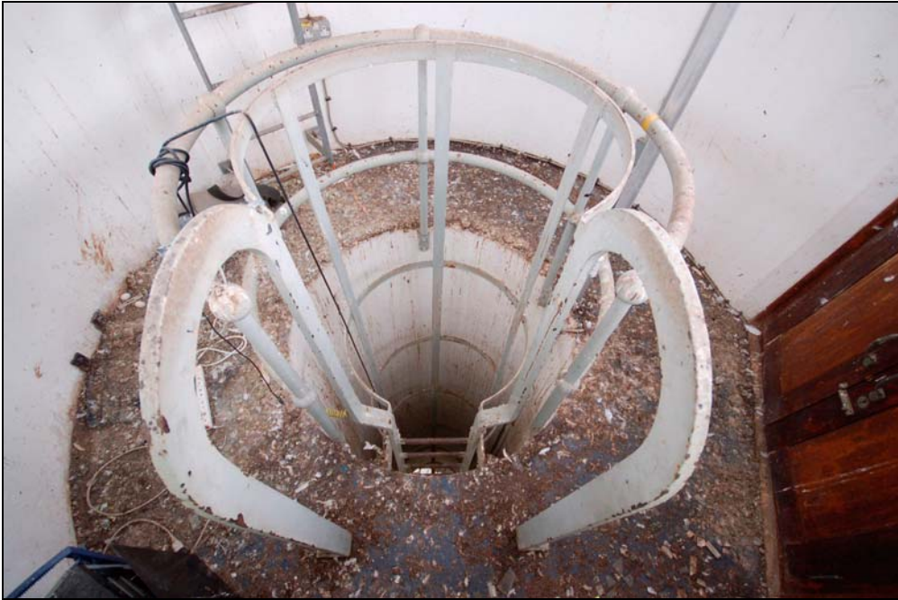
Plate 11 View down access shaft from turret room
