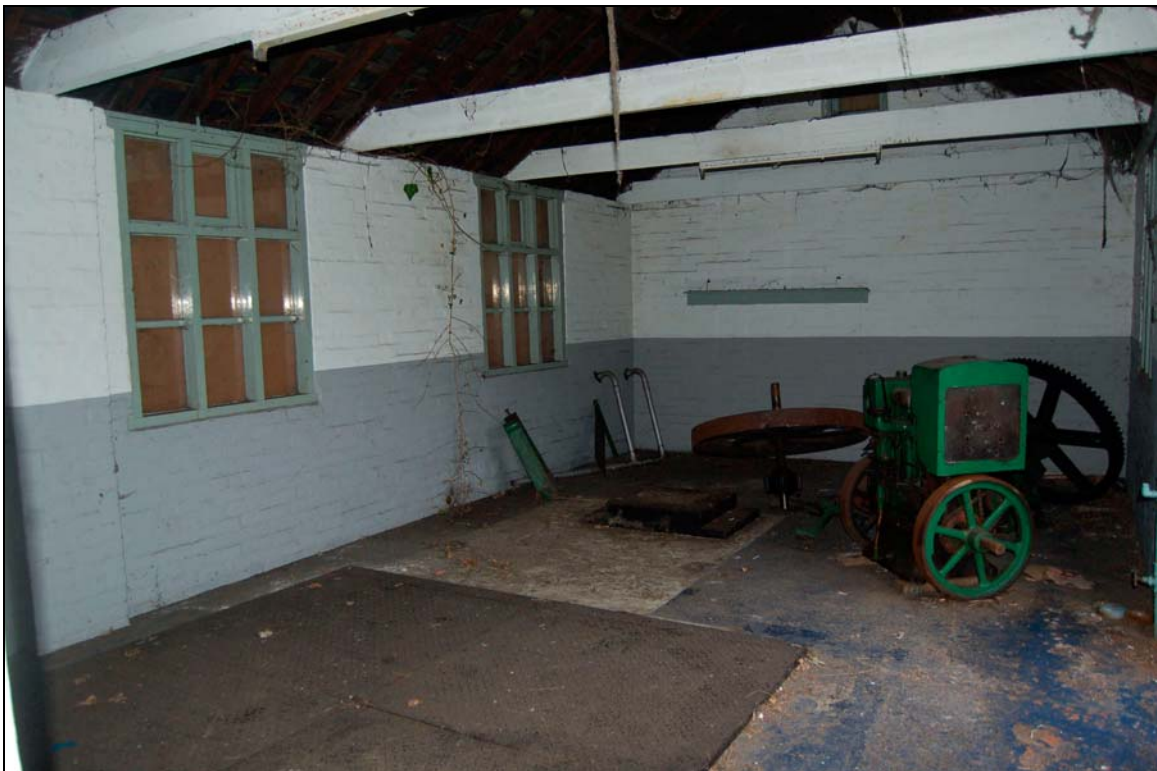
Plate 16 Interior of eastern well room, viewed to north-east
