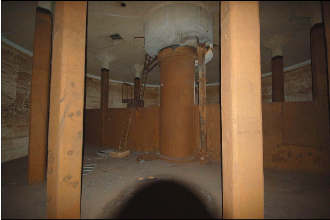
Plate 13 General interior of tank
