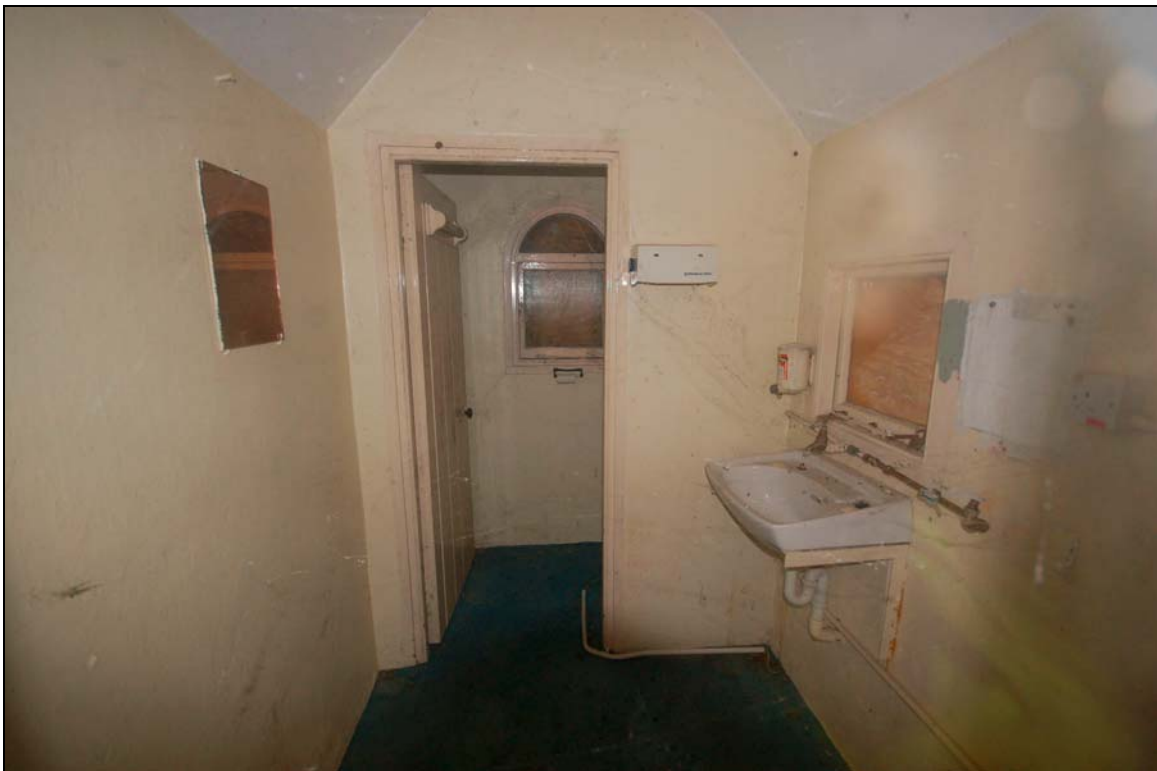
Plate 18 Interior of washroom/toilet
