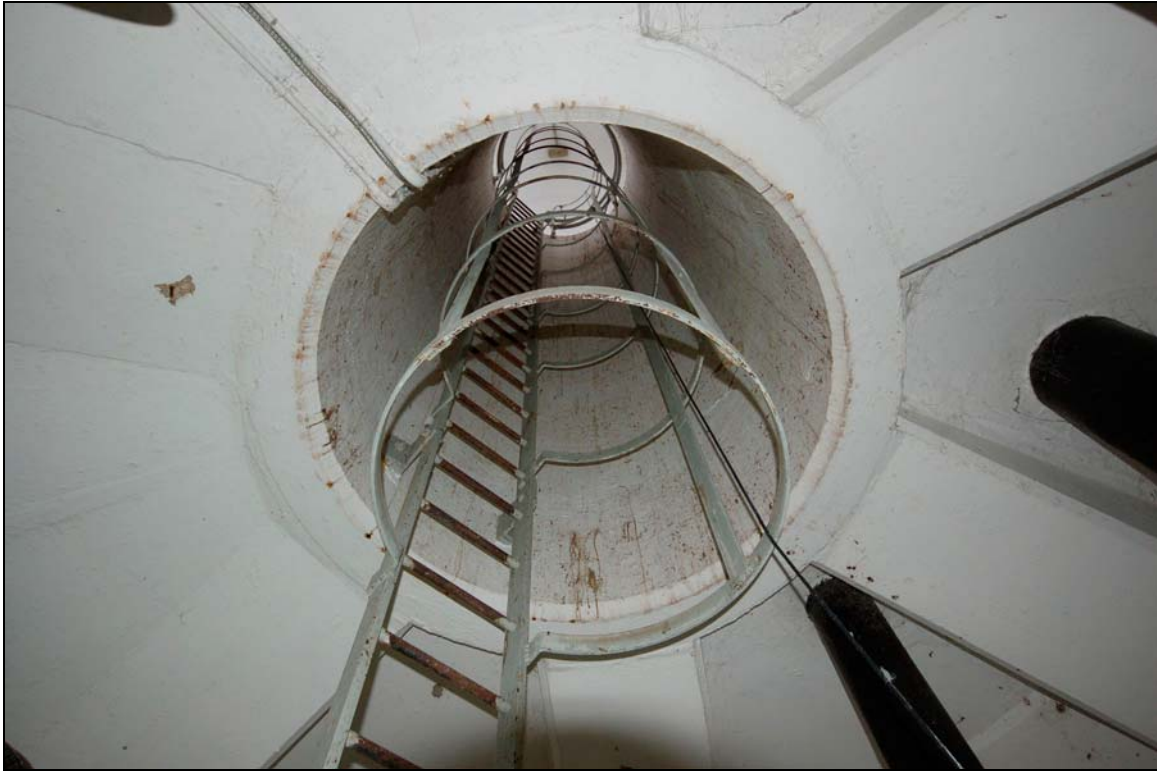
Plate 9 Access shaft through tank from level 2
