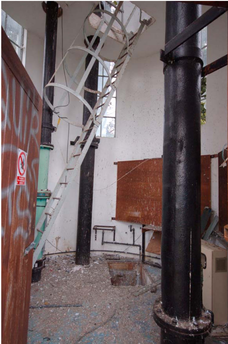
Plate 5 Engineer's room viewed to north
