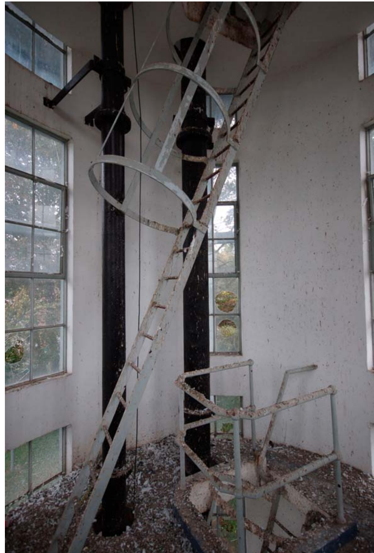
Plate 6 Level 1 viewed to north
