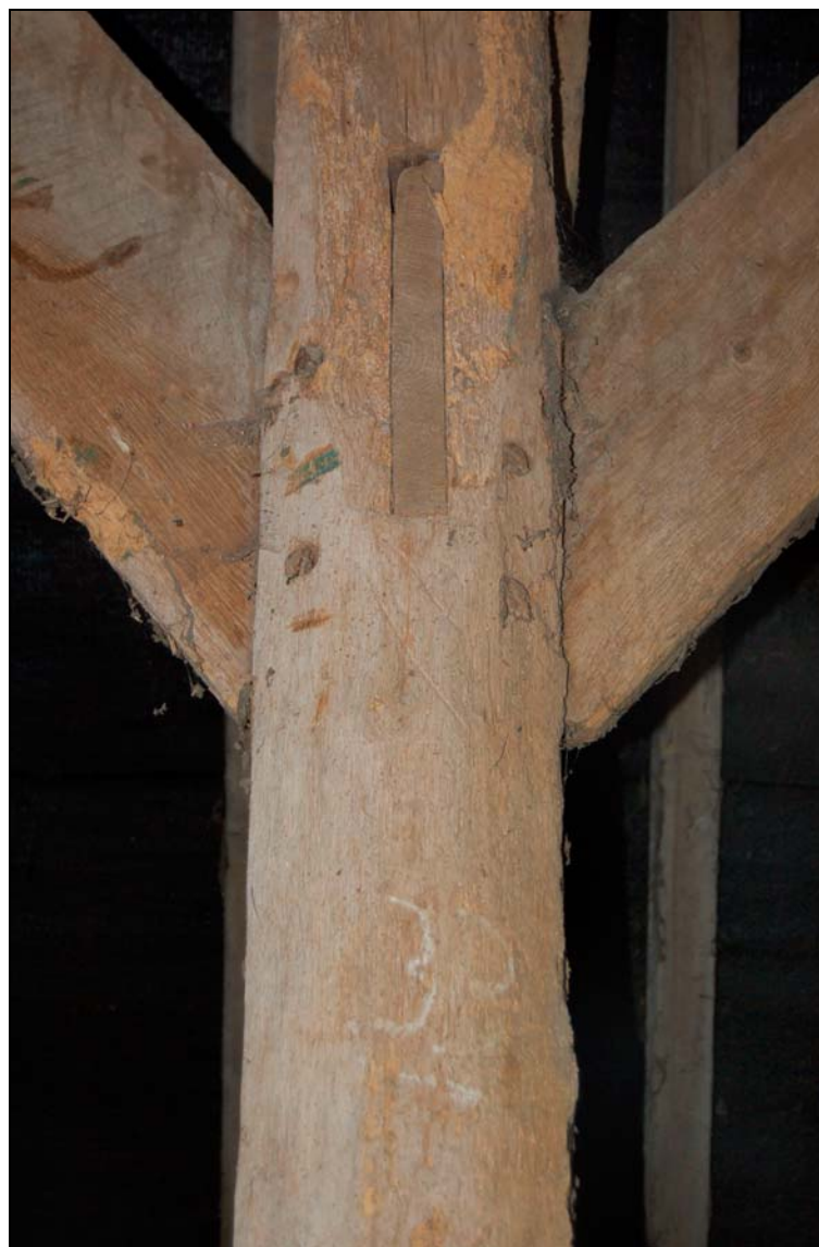
Plate 14 Scored carpenter's mark on T5 aisle post
