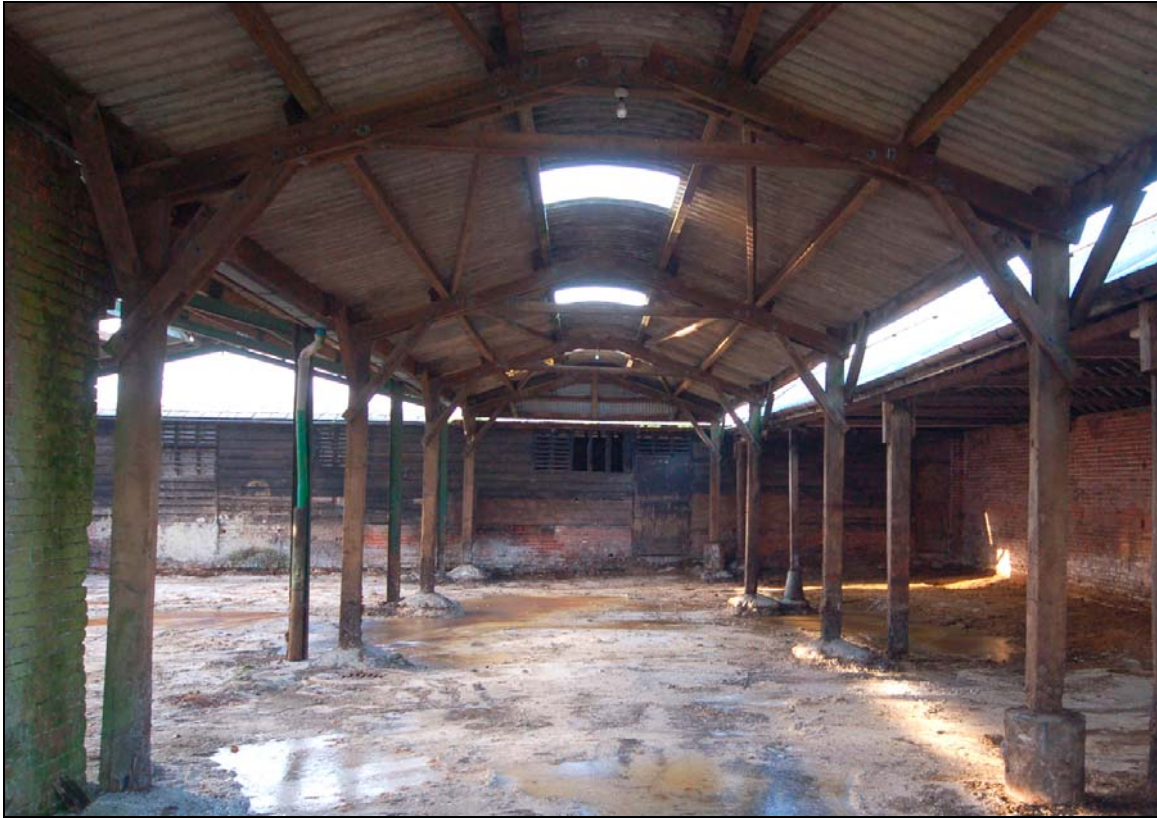
Plate 21 Stable viewed to west through covered yard
