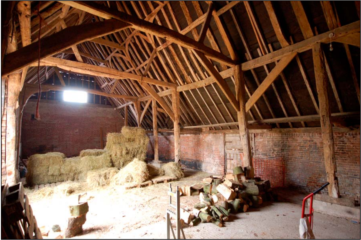
Plate 5 Interior of barn viewed to south
