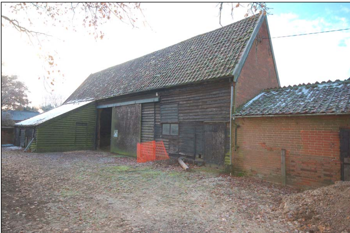
Plate 2 Barn, lean-to and cow house viewed to south
