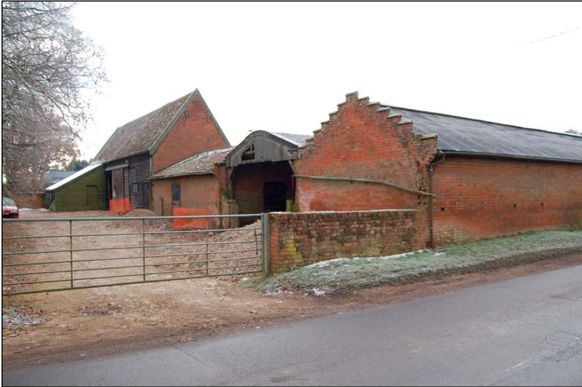
Plate 3 Farm group viewed to south from Church Road
