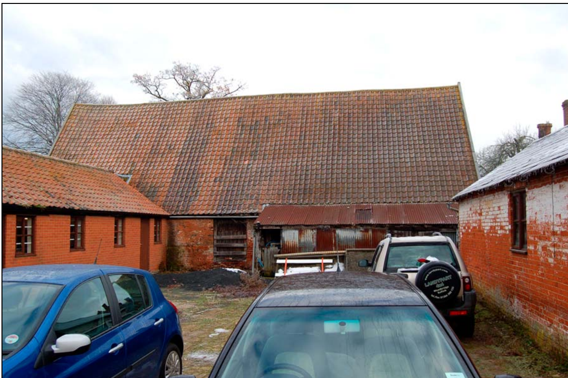
Plate 4 Rear of barn and former bullock yard viewed to east
