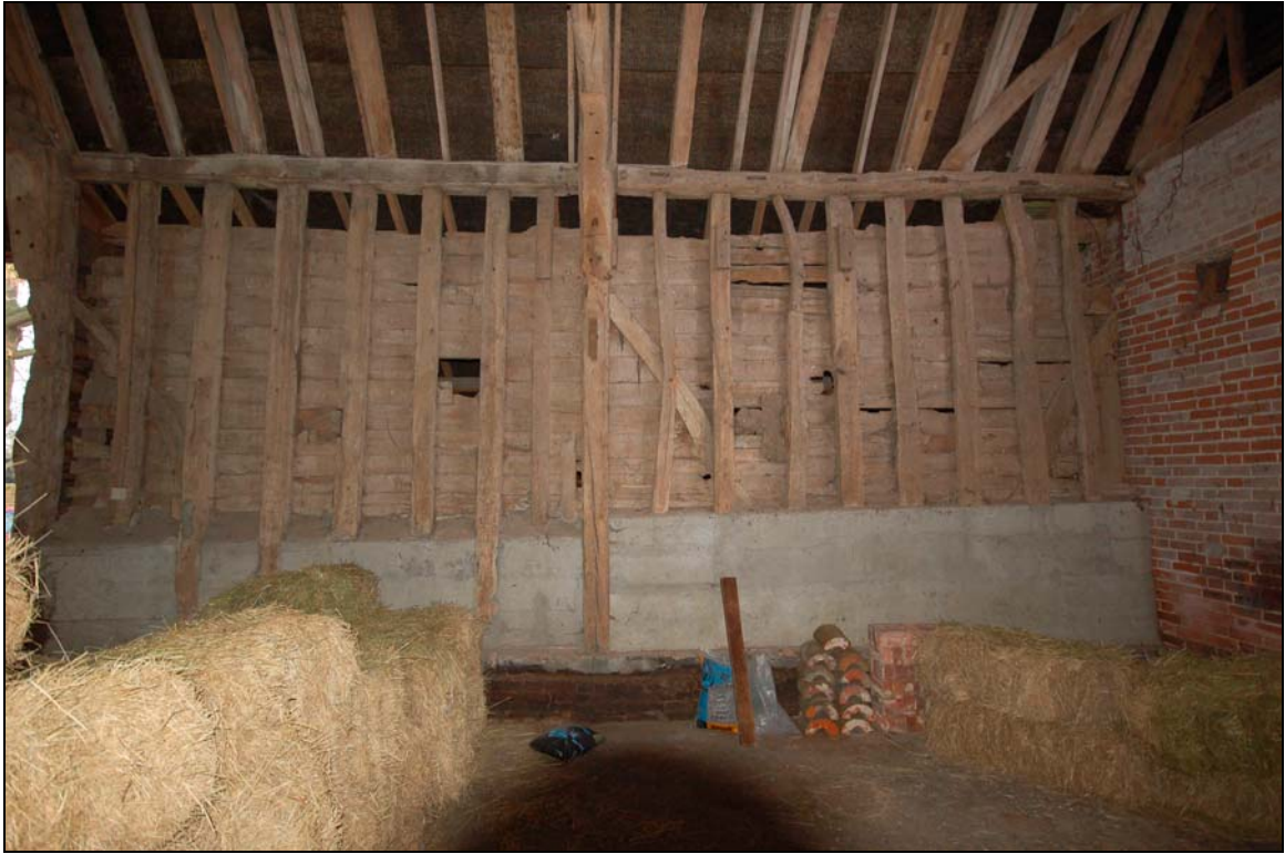
Plate 9 Wall-framing (southern bays)
