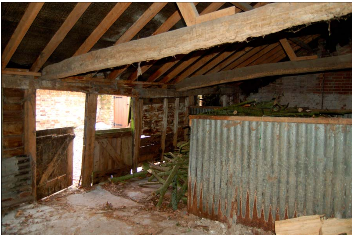
Plate 16 Lean-to interior viewed to east
