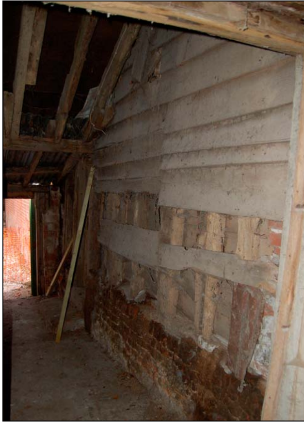
Plate 11 West wall of north bay (hay loft)
