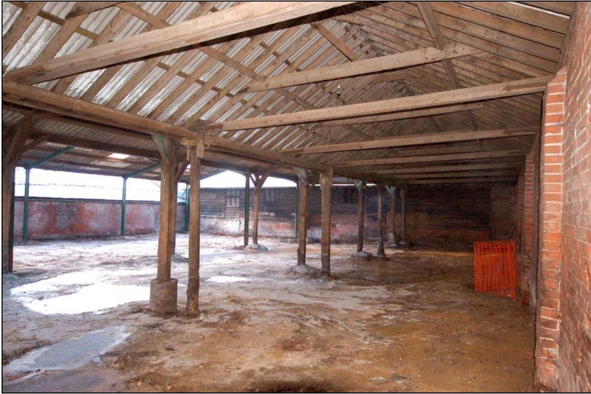
Plate 19 Interior of shelter shed viewed to west
