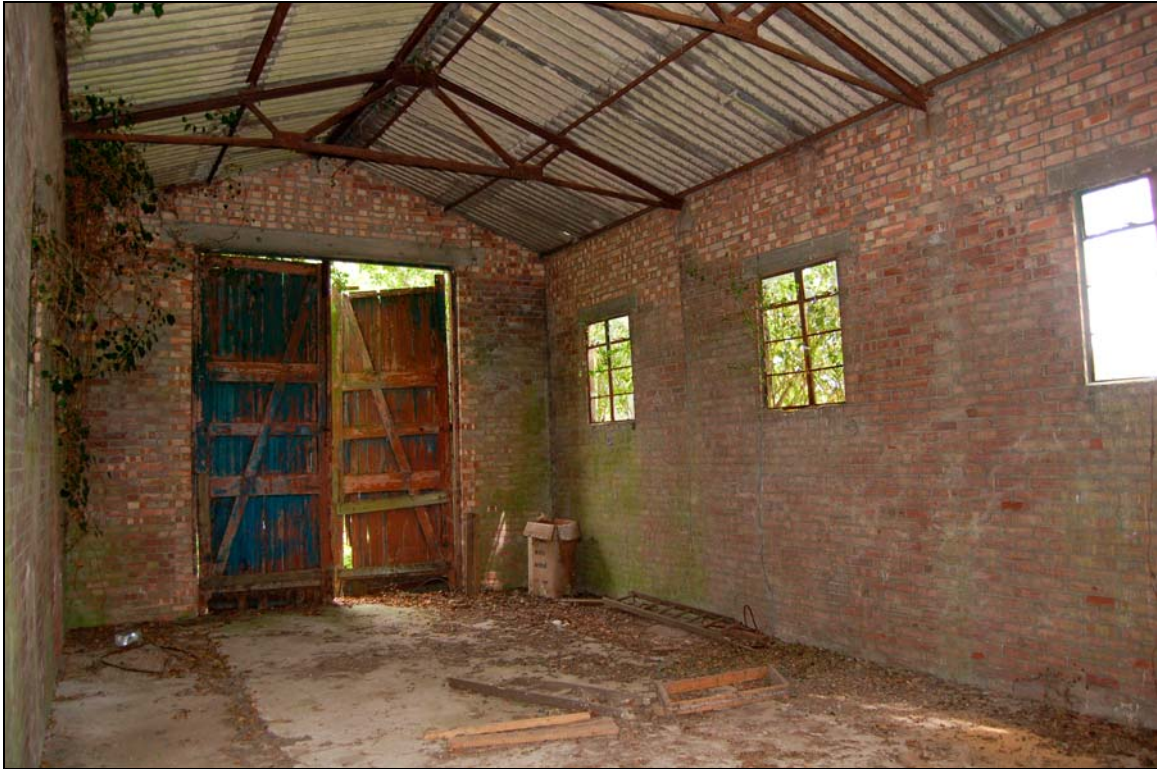
Plate 17 Interior of Floodlight Trailer and Tractor Shed 3
