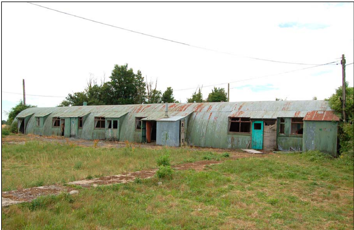
Plate 26 Maintenance Unit Block 9 viewed to south
