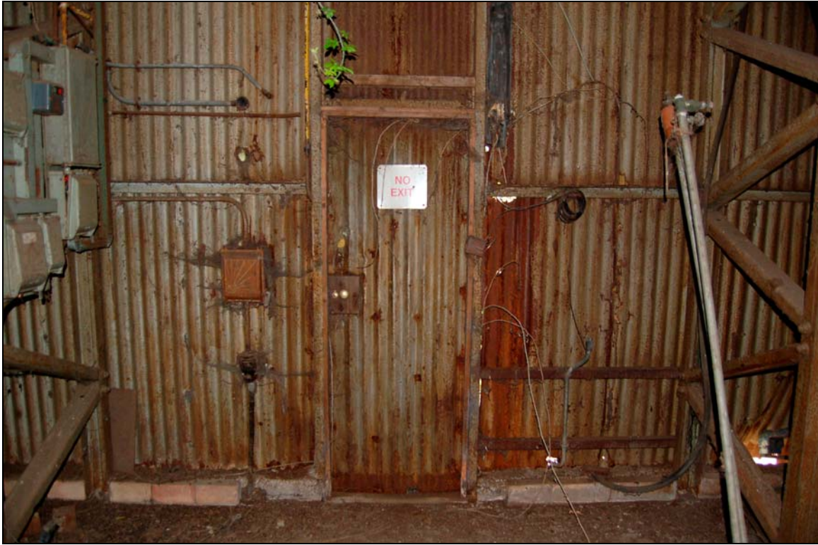
Plate 13 Personnel door on south-east wall
