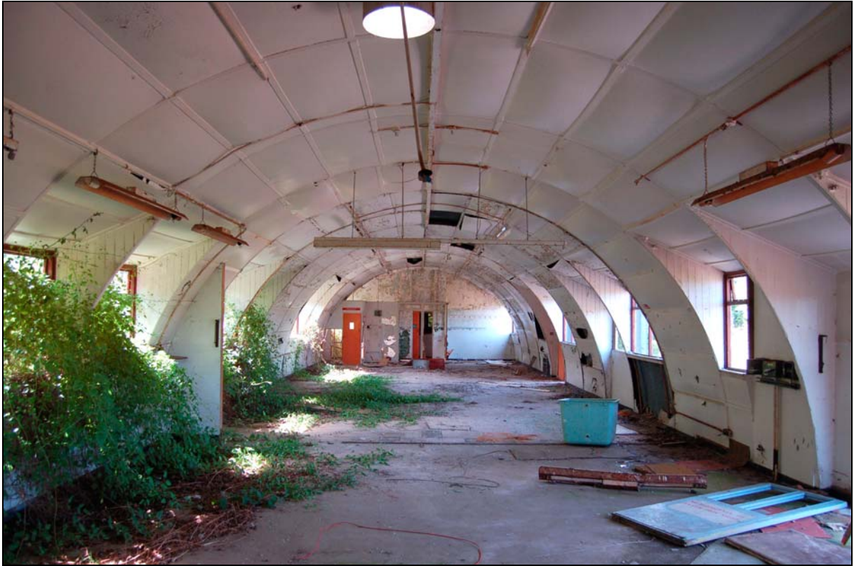
Plate 27 Interior of Maintenance Unit Block viewed to north-west
