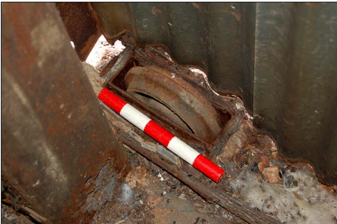
Plate 4 Roller-track door mechanism
