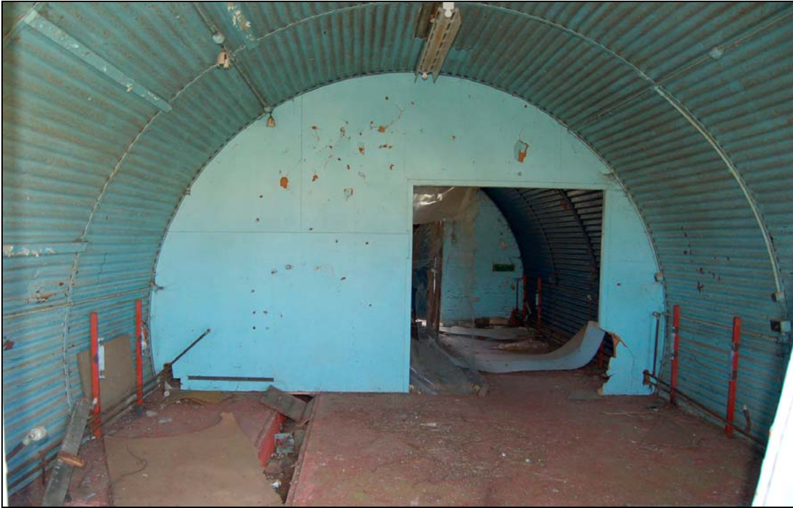
Plate 29 Interior of General Purpose Hut viewed to south-west
