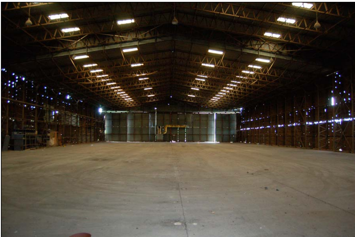
Plate 6 Interior of hanger 1 viewed to south-west
