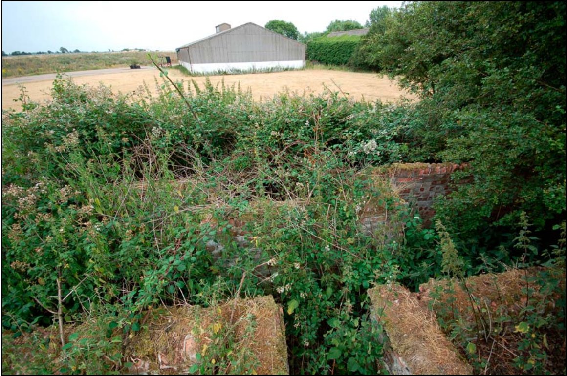
Plate 21 Blast shelter 5 viewed to north
