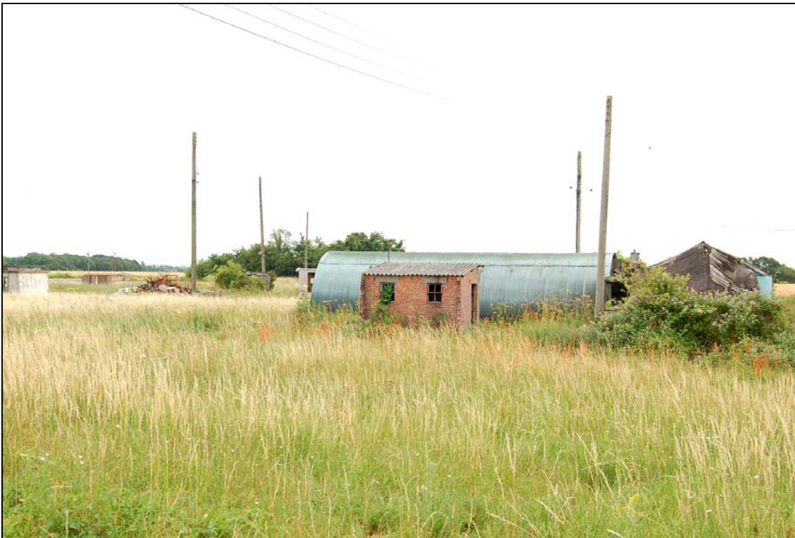
Plate 30 Latrines/sub-station 11 viewed to south-west in front of General Purpose Hut
