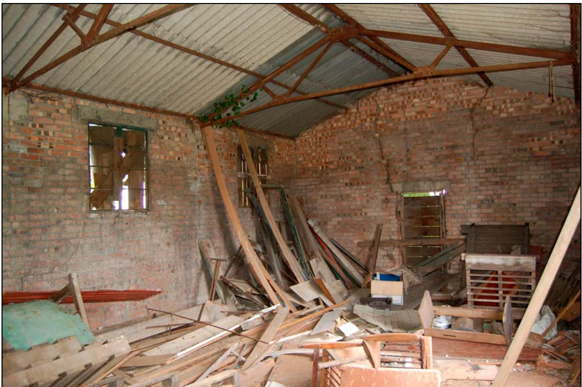
Plate 16 Interior of NFE Store viewed to west
