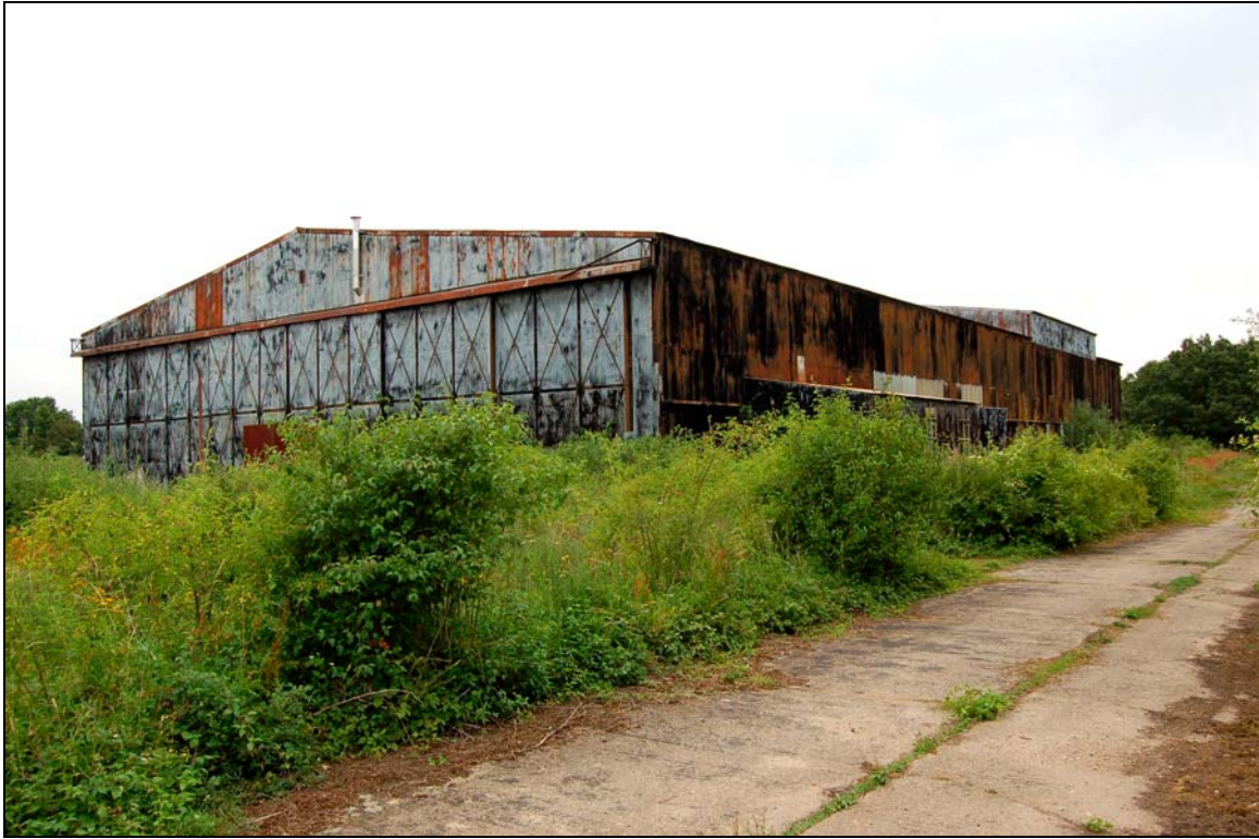
Plate 3 Hanger 1 viewed to north
