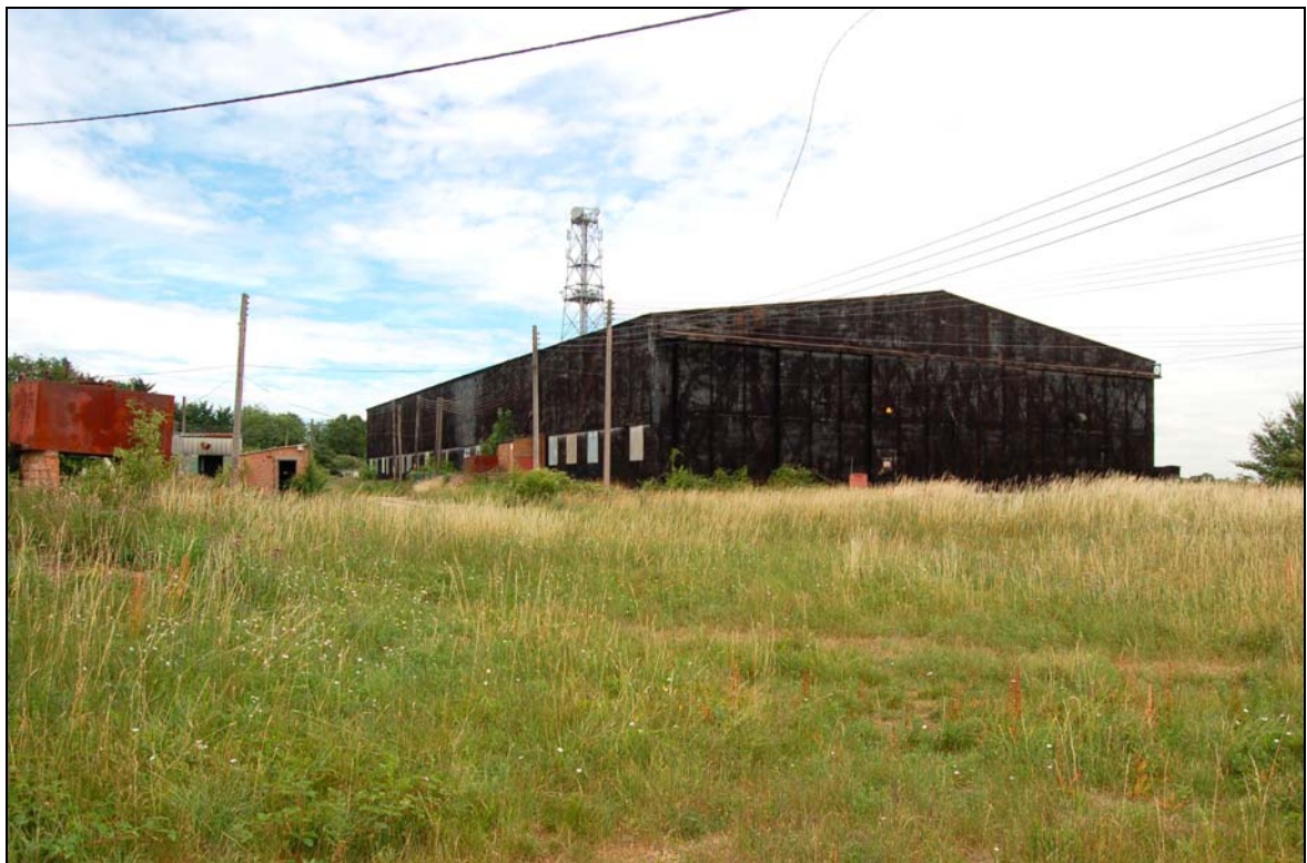
Plate 22 Hanger 7 viewed to north
