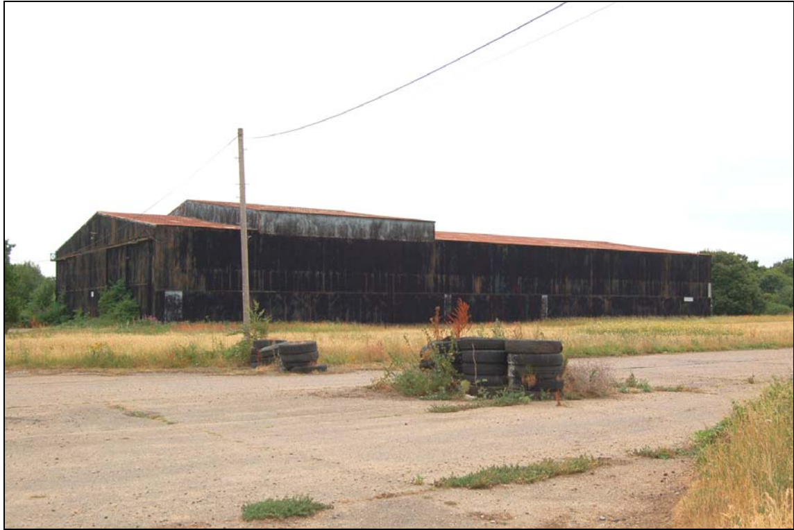
Plate 1 Hanger 1 viewed to south
