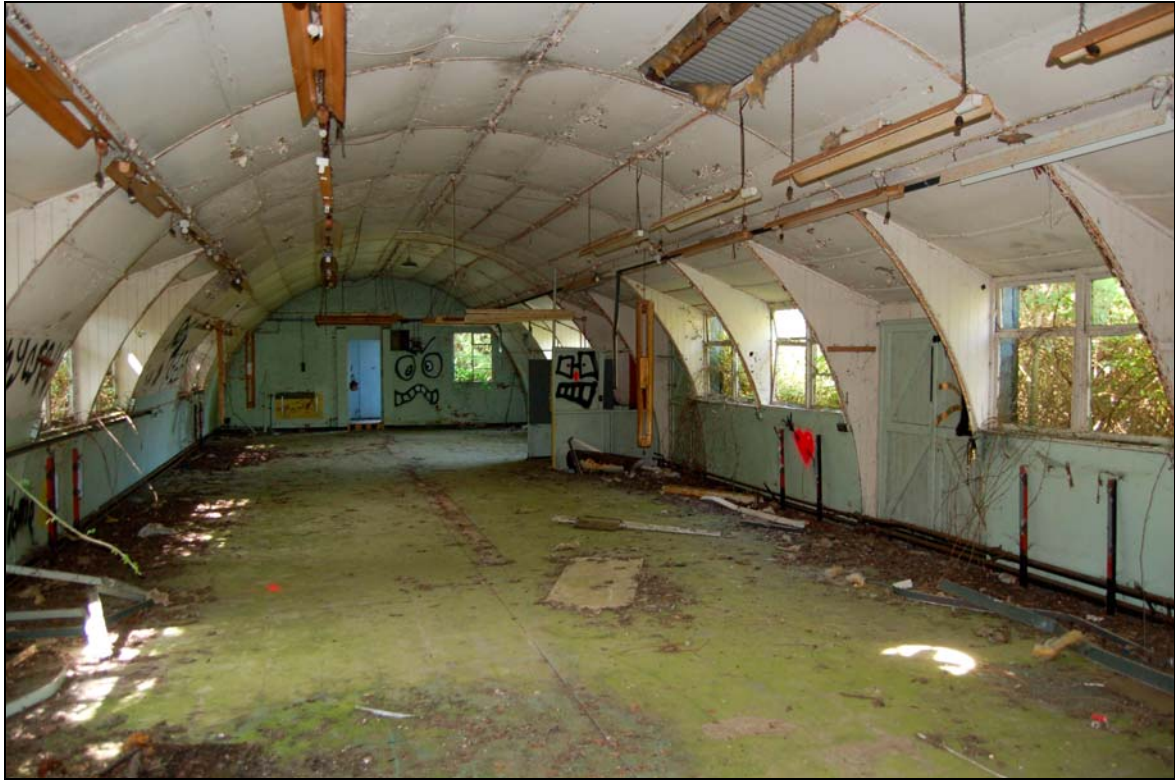
Plate 25 Interior of Armoury and Maintenance Unit viewed to north-west
