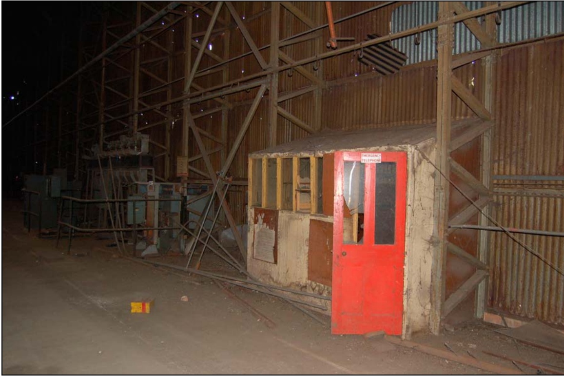
Plate 11 Emergency telephone booth
