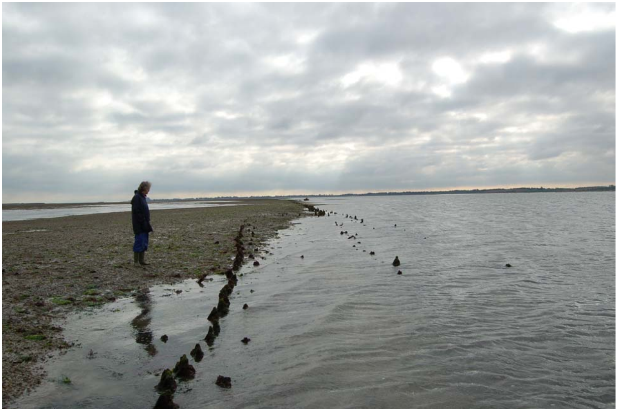
Plate 4 Main alignment at Collins Creek in 2007, looking west
