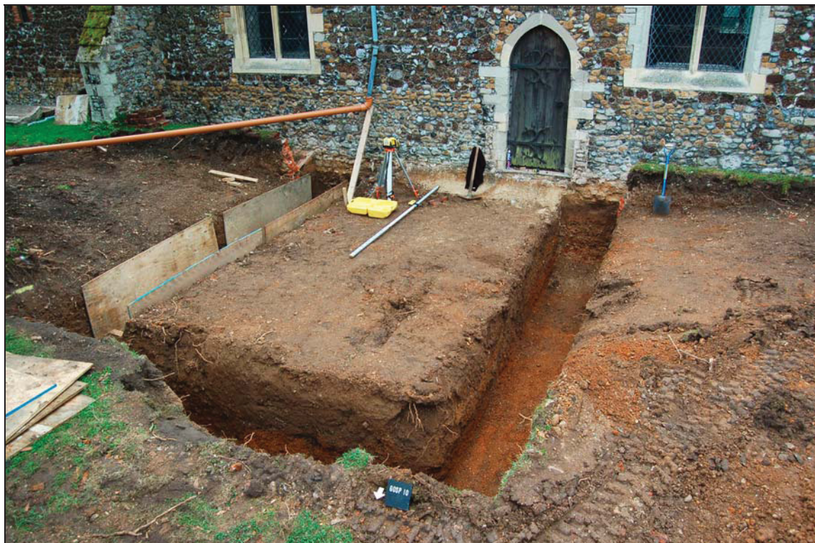
Plate 1 Foundation trench for north extension viewed to south
