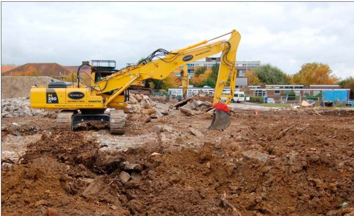
Plate 4: Monitoring of foundation removal (looking south)
