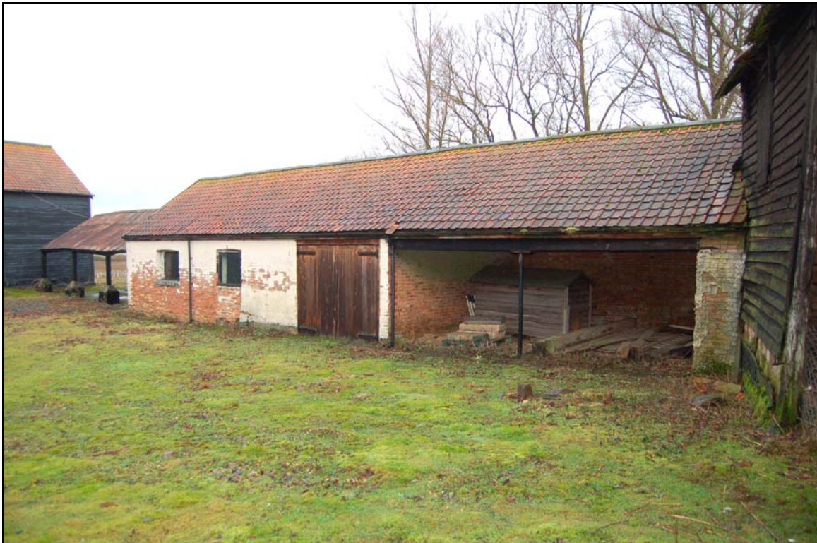
Plate 13 North range (buildings 2 and 3) viewed to north-west
