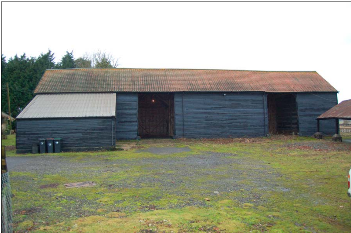
Plate 2 North-west elevation, facing the yard
