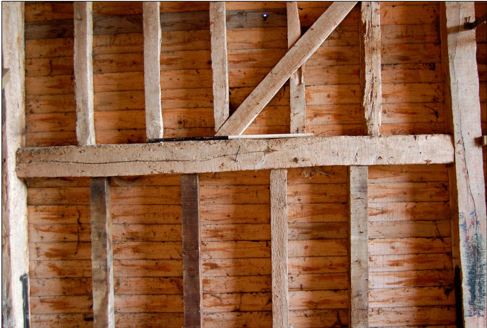
Plate 11 Carpenters marks in porch (1-6 from right to left)
