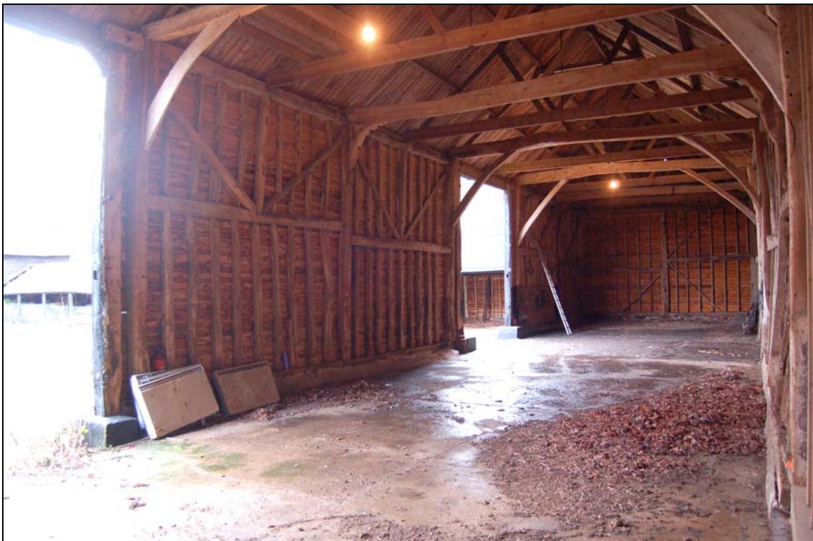
Plate 10 Wall-framing on south-east wall, viewed to south
