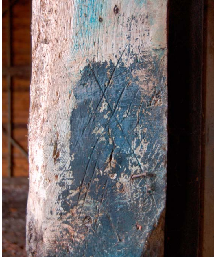
Plate 12 Carpenters mark on T3 midstrey/porch post
