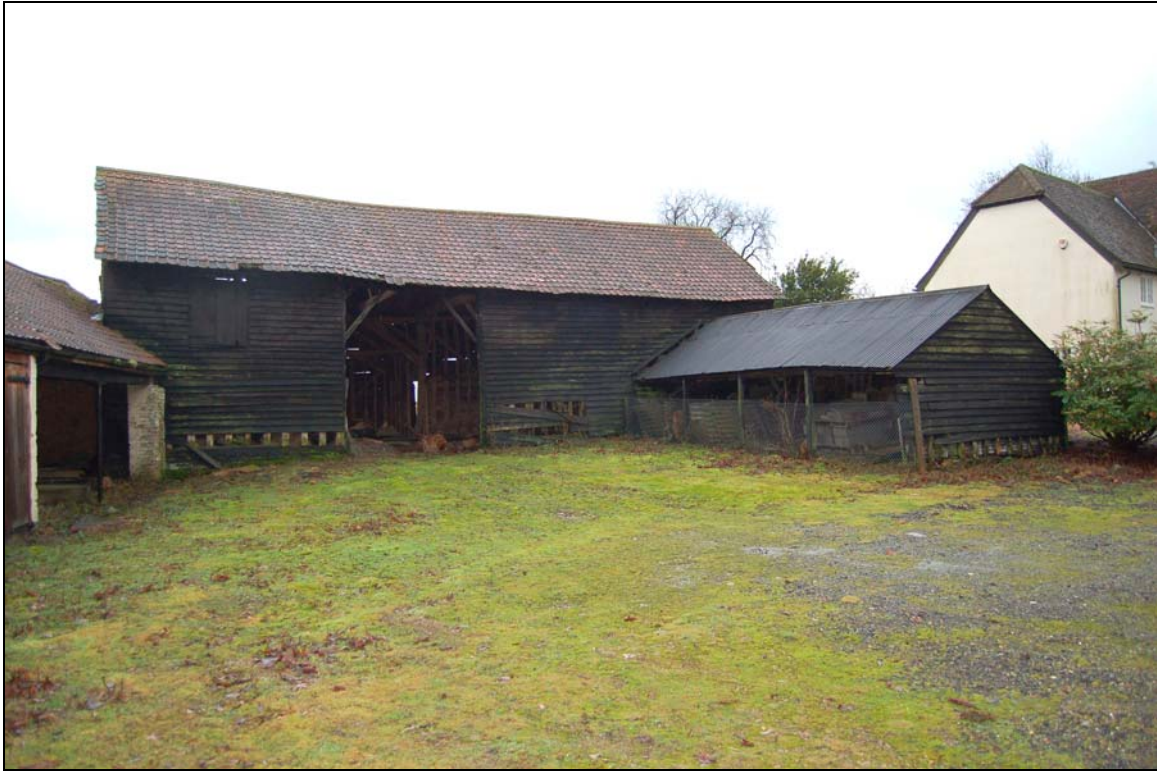
Plate 14 Barn 4 and shed 5 viewed to south
