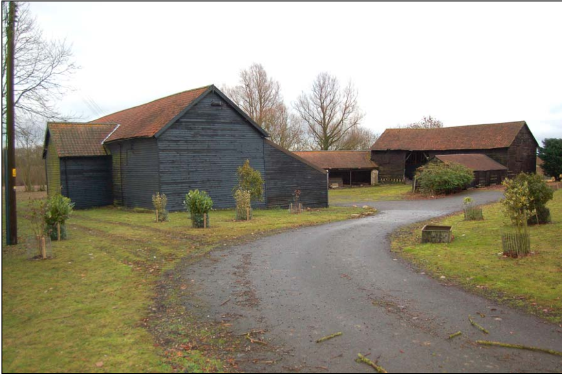
Plate 1 Barn 1 and other farm buildings viewed to north-east
