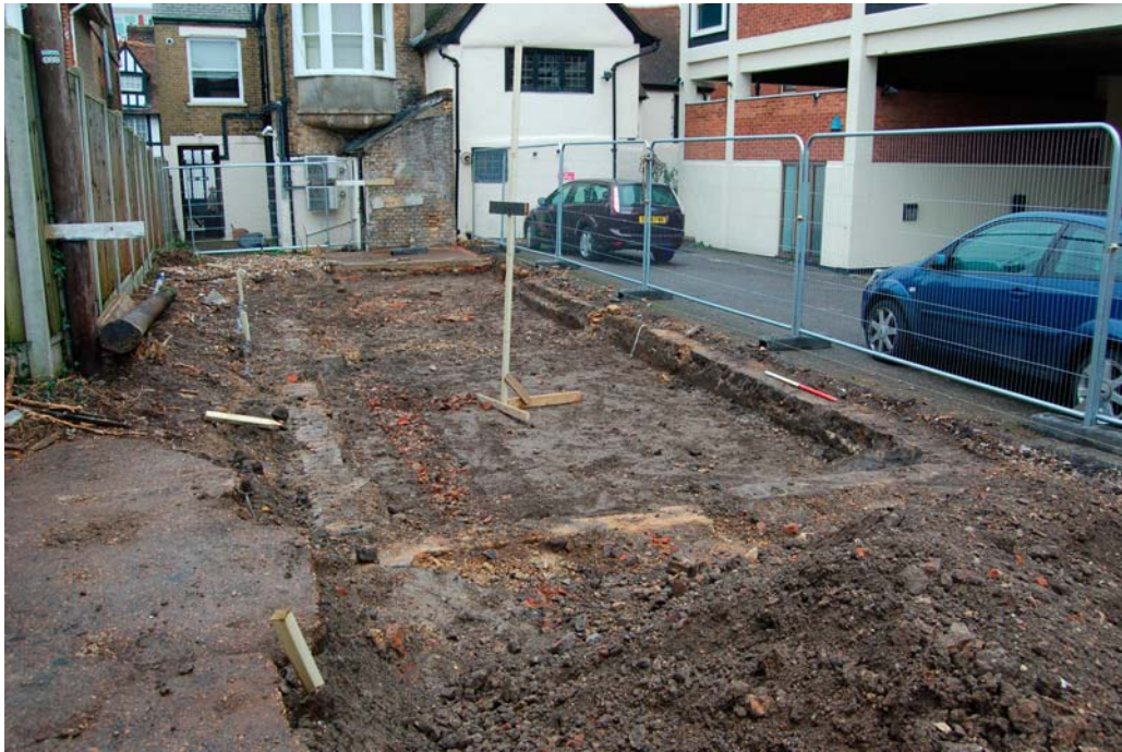
Plate 3. Modern walls 1 and 2 and drain 3 looking north. 1m scale.
