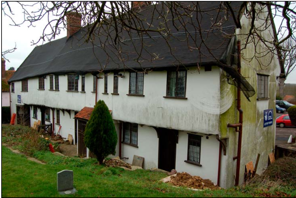
Plate 1 Guildhall during excavation works, viewed to west
