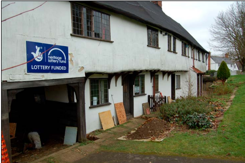
Plate 2 Guildhall during excavation works, viewed to north
