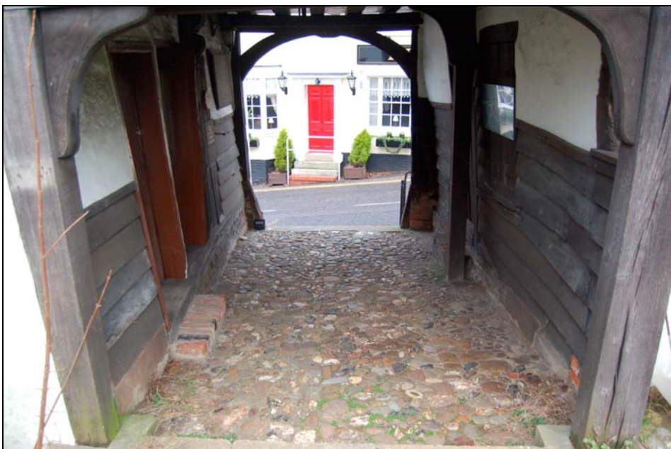
Plate 12 Passage viewed to north-west
