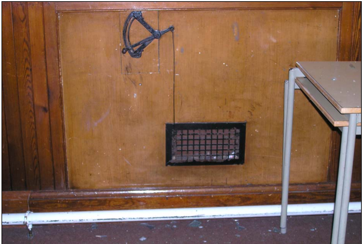
Plate 23 Air vent and control mechanism in Storeroom 1 (2006)
