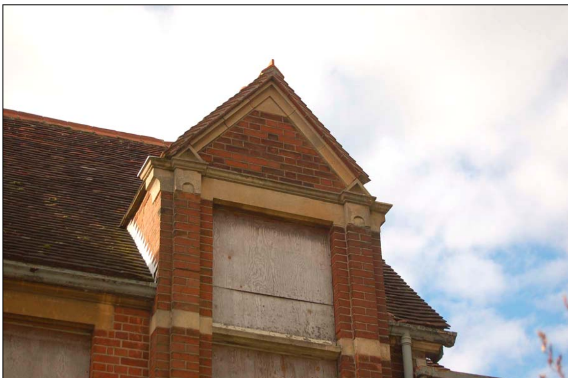
Plate 10 Codestone detailing to gambrel-roofed projections on east side
