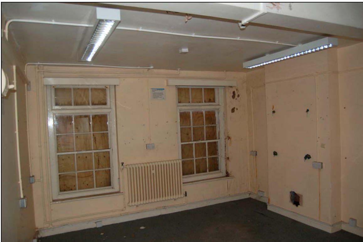
Plate 50 Ground floor room in original infirmary (4)
