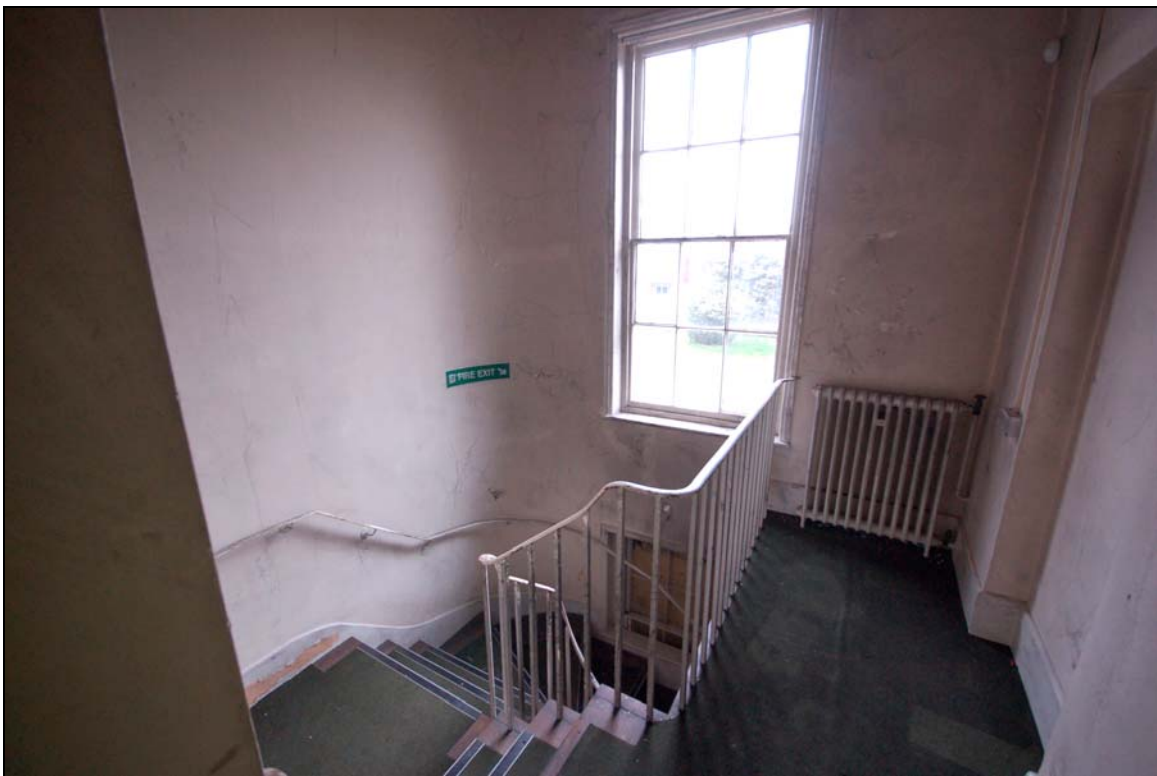
Plate 10 Top landing and former boardroom entrance
