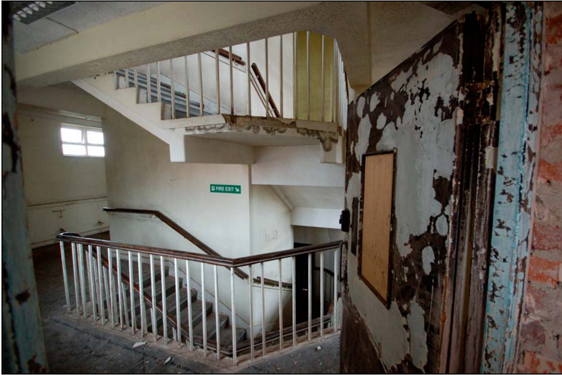
Plate 17 Hub staircase and lift from first floor (block D)
