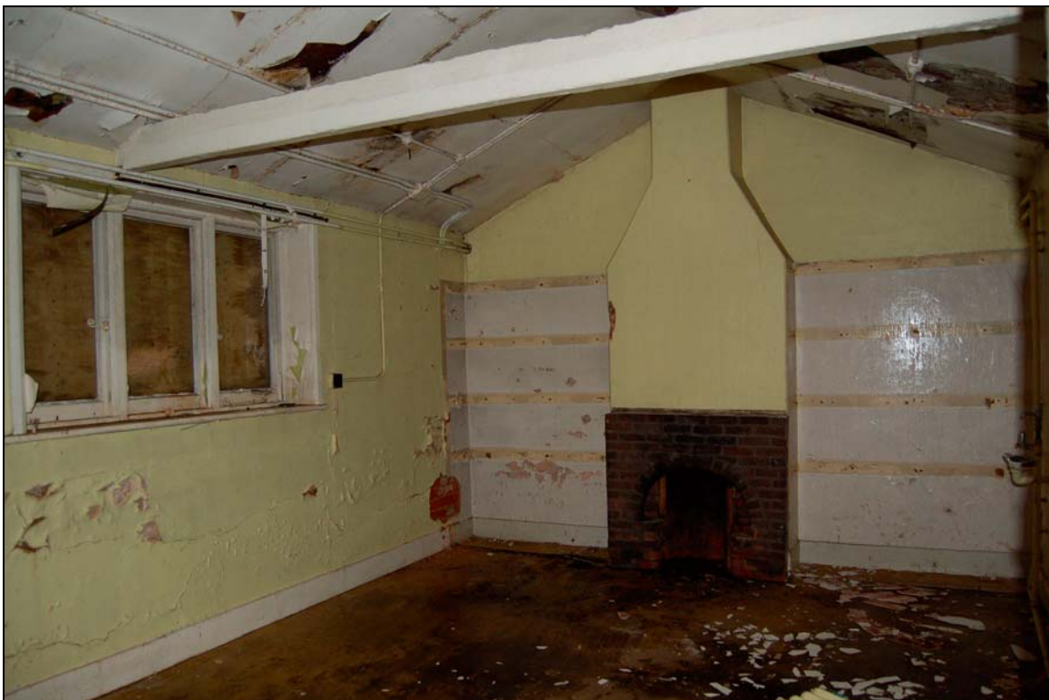
Plate 42 Interior of outbuilding 3a viewed to north-east
