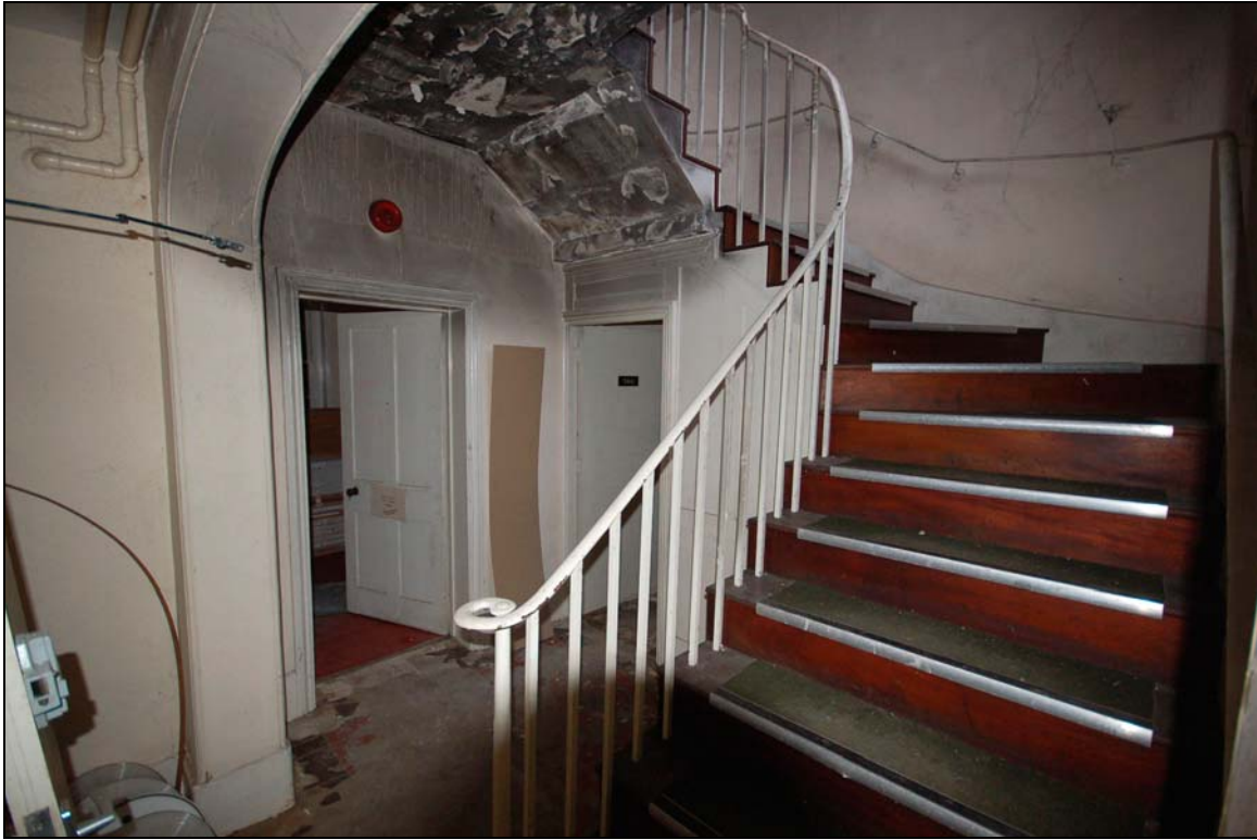
Plate 9 Stairs viewed to south-west
