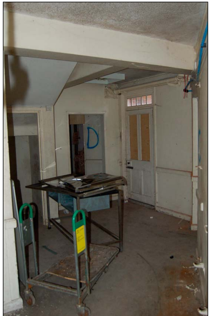
Plate 16 Interior of hub, viewed to doorway into north yard
