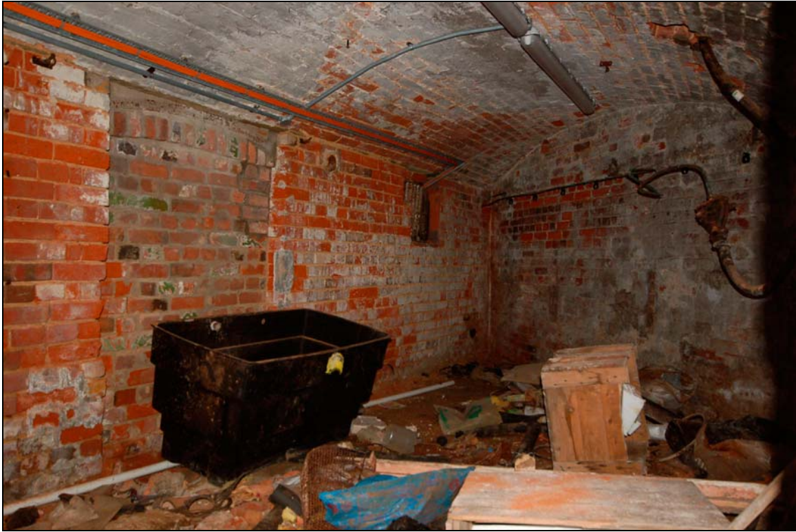
Plate 19 Basement underneath hub
