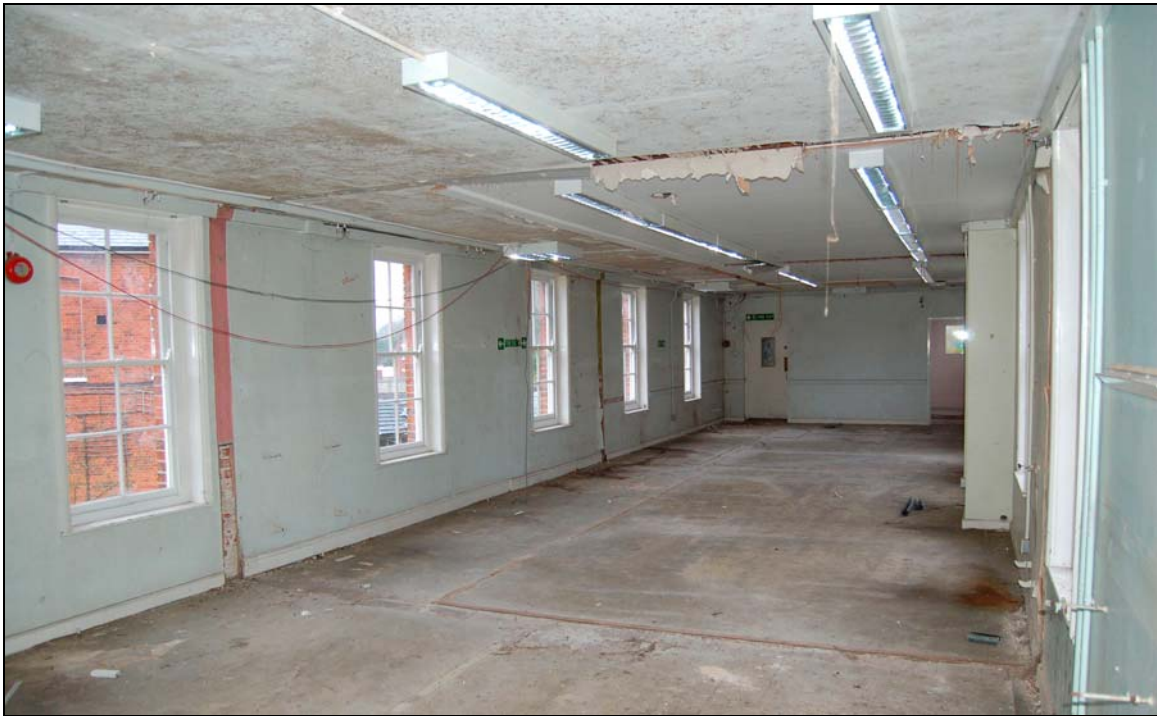
Plate 30 First floor of block C viewed to north-east
