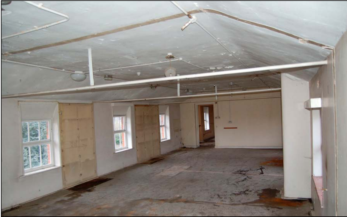
Plate 31 Block C, second floor viewed to north
