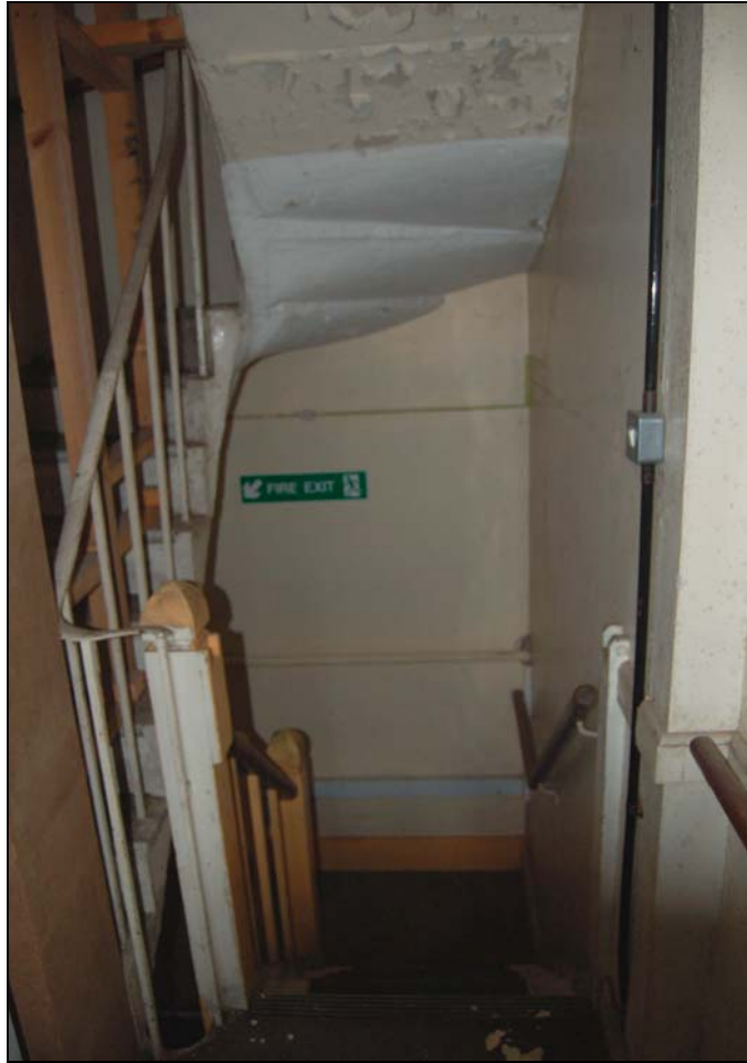
Plate 33 Change from wooden to cast iron stair on first floor landing
