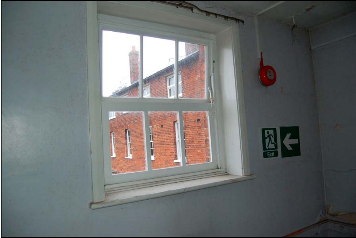
Plate 35 Original window viewed internally
