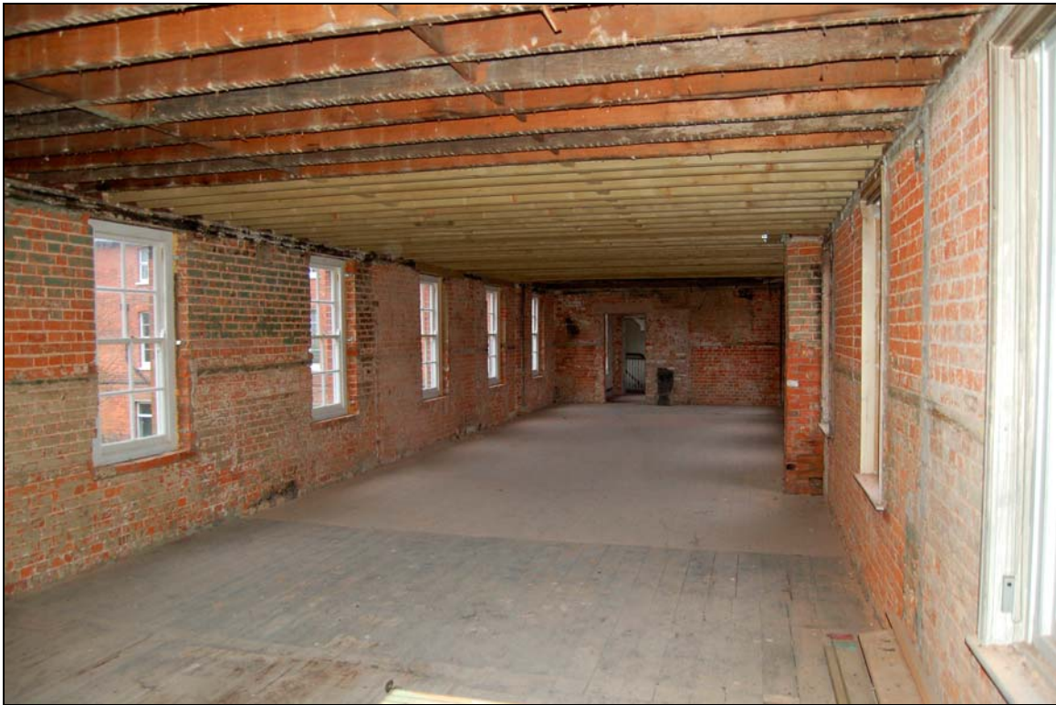
Plate 36 Stripped-out first floor of block D, viewed to south-east
