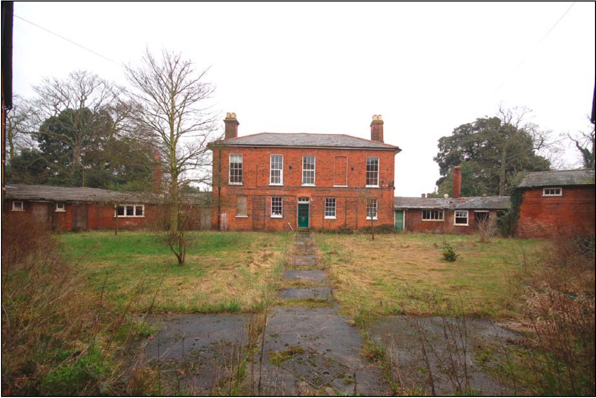
Plate 5 Rear elevation of Master's House and north yard
