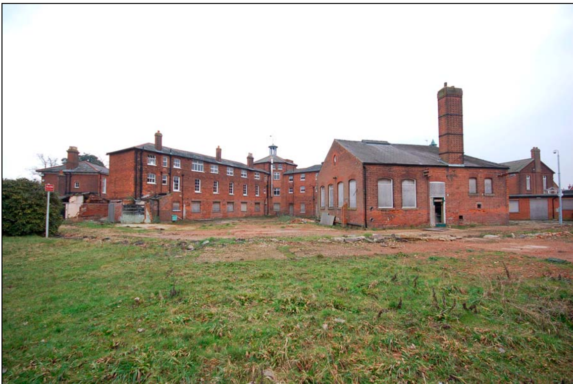
Plate 24 West yard and laundry building viewed to east
