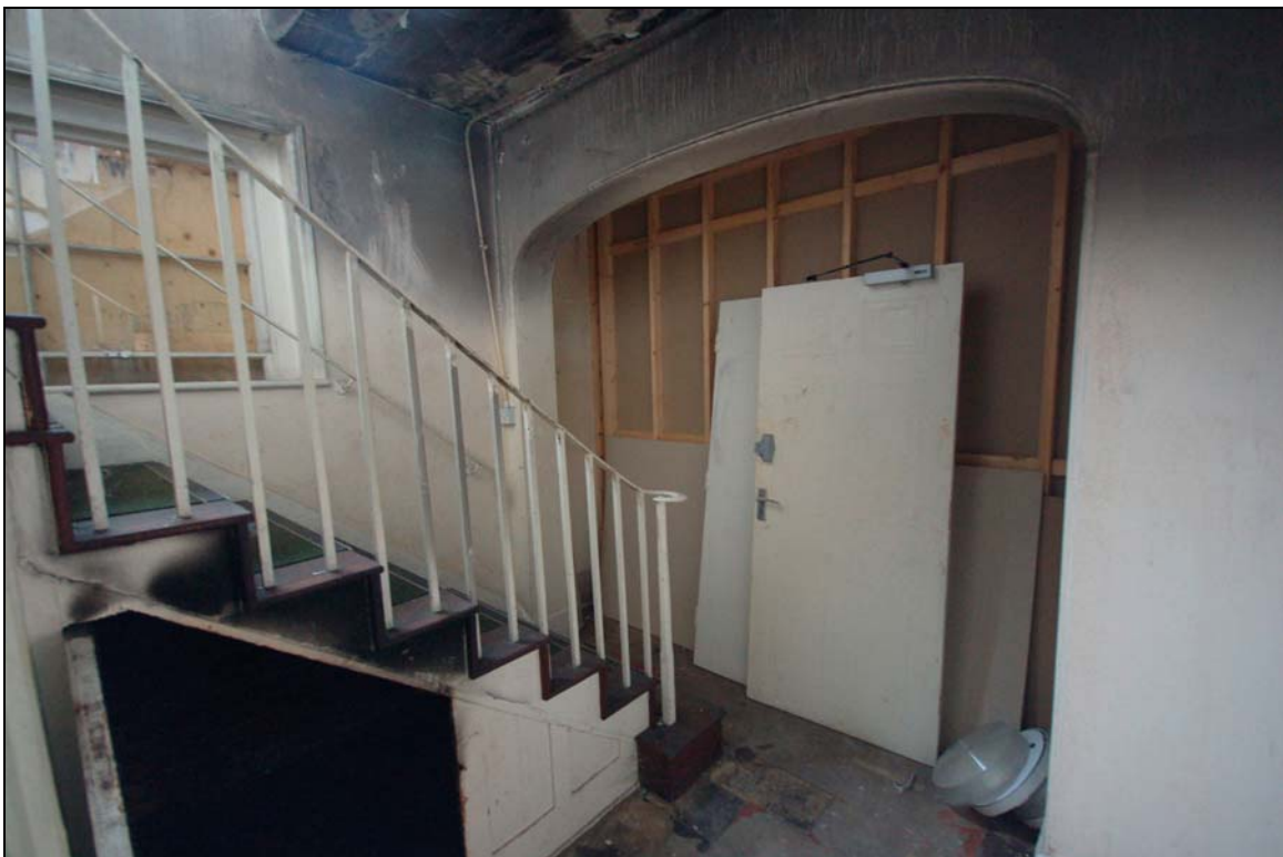
Plate 8 Stairs in Master's House and arch from entrance lobby
