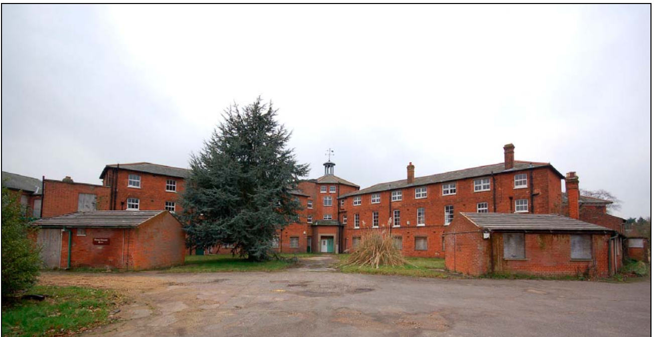
Plate 14 East yard and outbuilding range
