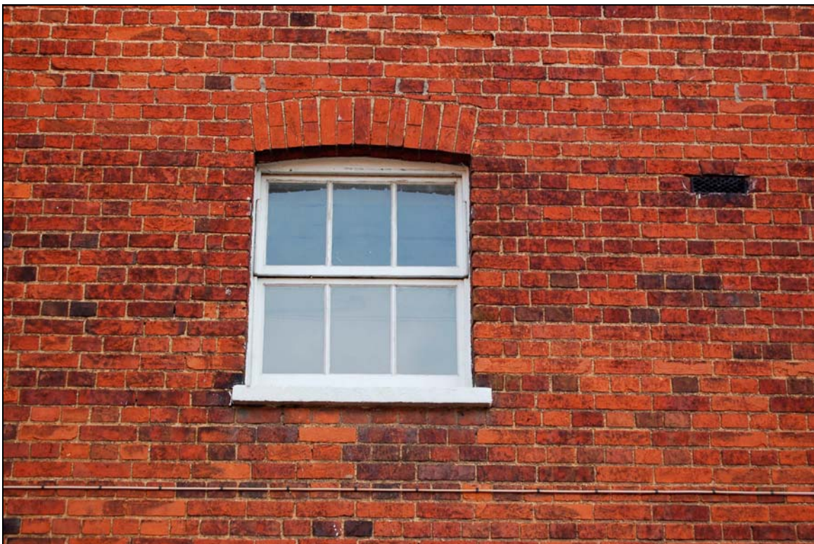
Plate 26 Detail of original tilting window
