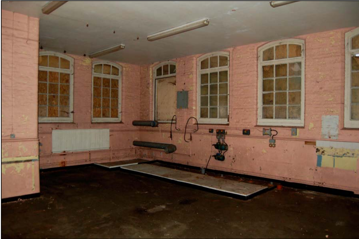
Plate 61 Interior of washroom viewed to north-west
