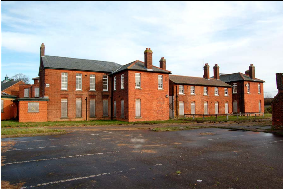
Plate 47 Rose House viewed to north-east
