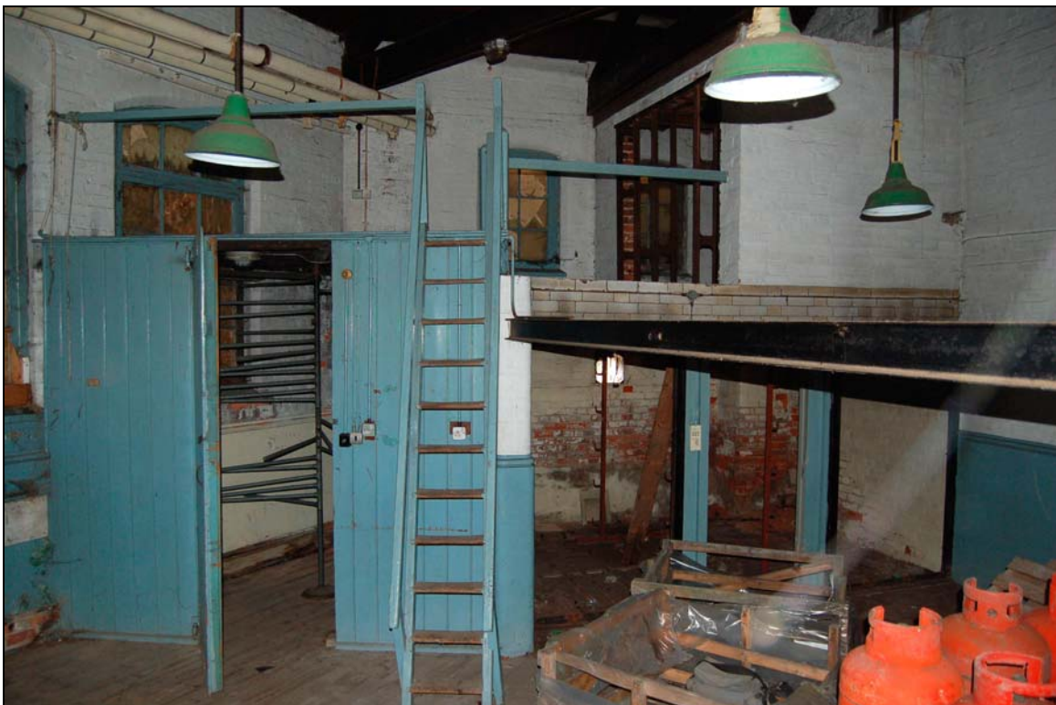
Plate 62 Interior of laundry viewed to west
