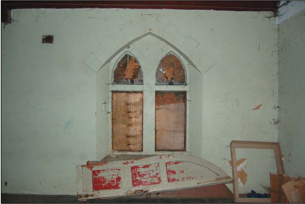
Plate 59 Detail of chapel window and original doors
