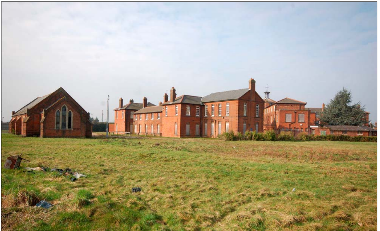
Plate 2 Chapel, infirmary and workhouse viewed to north-west
