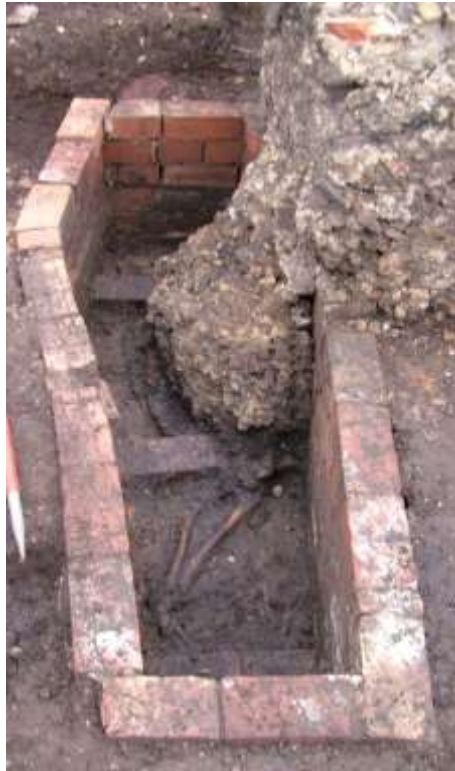
Fig.6: Sk36: Modern damage.
