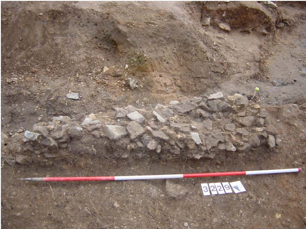
Figure 109: Phase 8.2, fragment of clay-bonded stone wall footing G1005, possibly forming the southern wall of a structure, perhaps St. Michael's church, in Plot Seven
