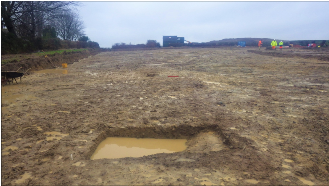
Plate 5: Excavation Area 2, general view, looking west
