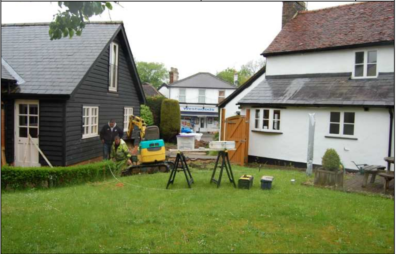
Plate 1: View of site, looking north west
