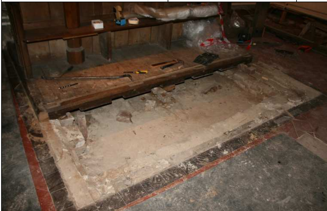
Plate 1: Removal of the pews, looking north-west
