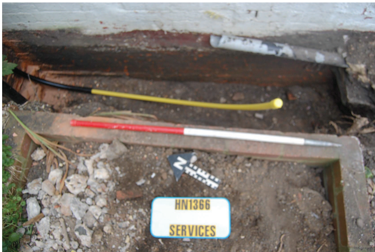
Plate 25 - Gas trench and drain, looking NE
