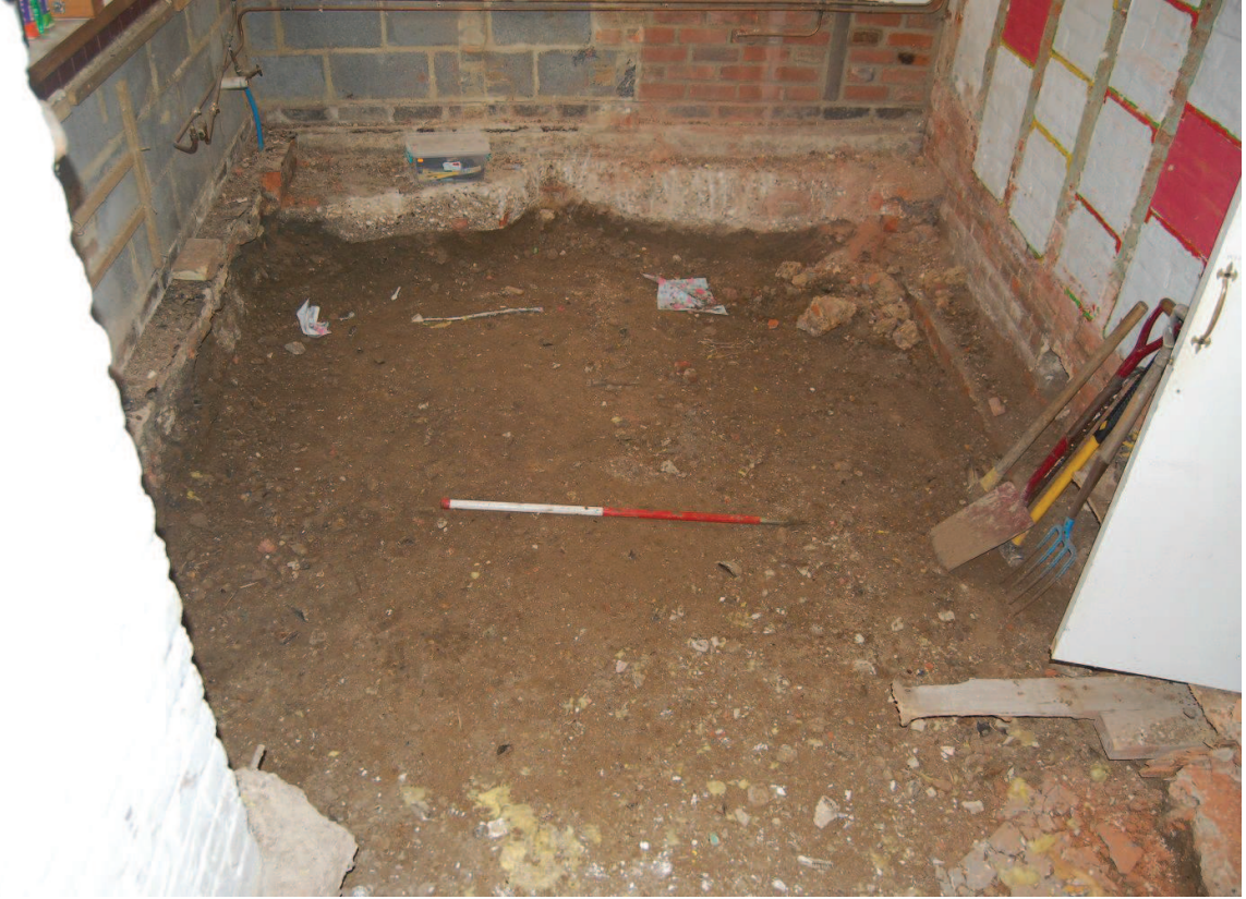
Plate 26 - Kitchen ground reduction, looking E
