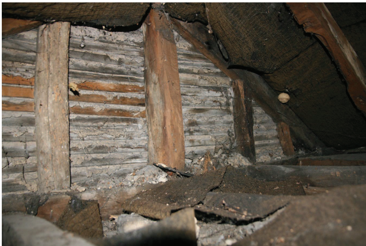
Plate 23 - Roof space, showing exposed timber-framing, looking W
