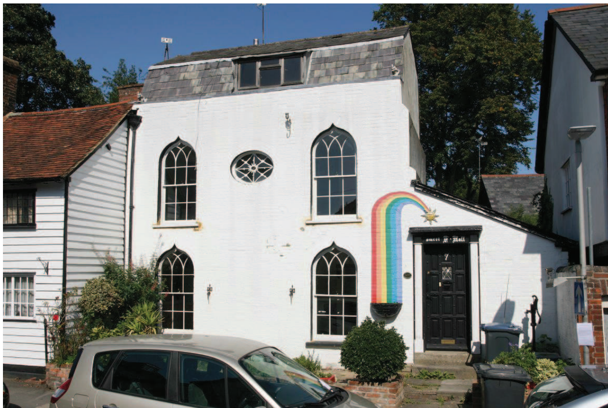
Plate 01 - South and east exterior elevation, looking N
