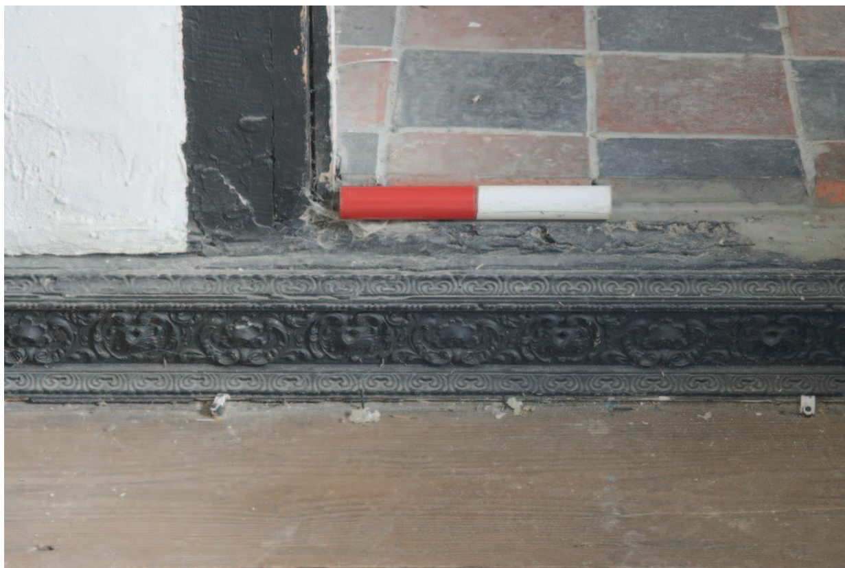
Plate 05b - Skirting in east elevation, looking E
