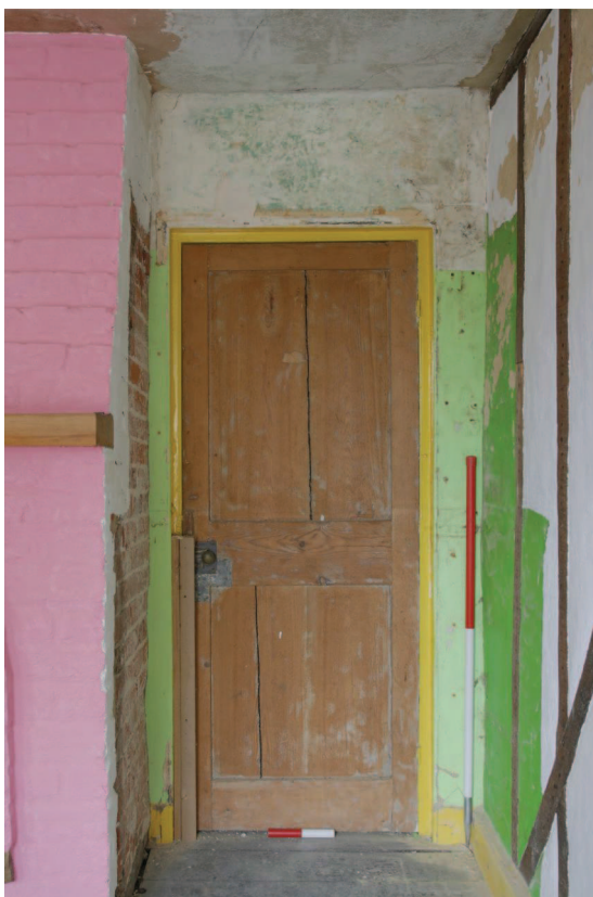
Plate 19 - Bedroom 1, N elevation, eastern doorway, looking N
