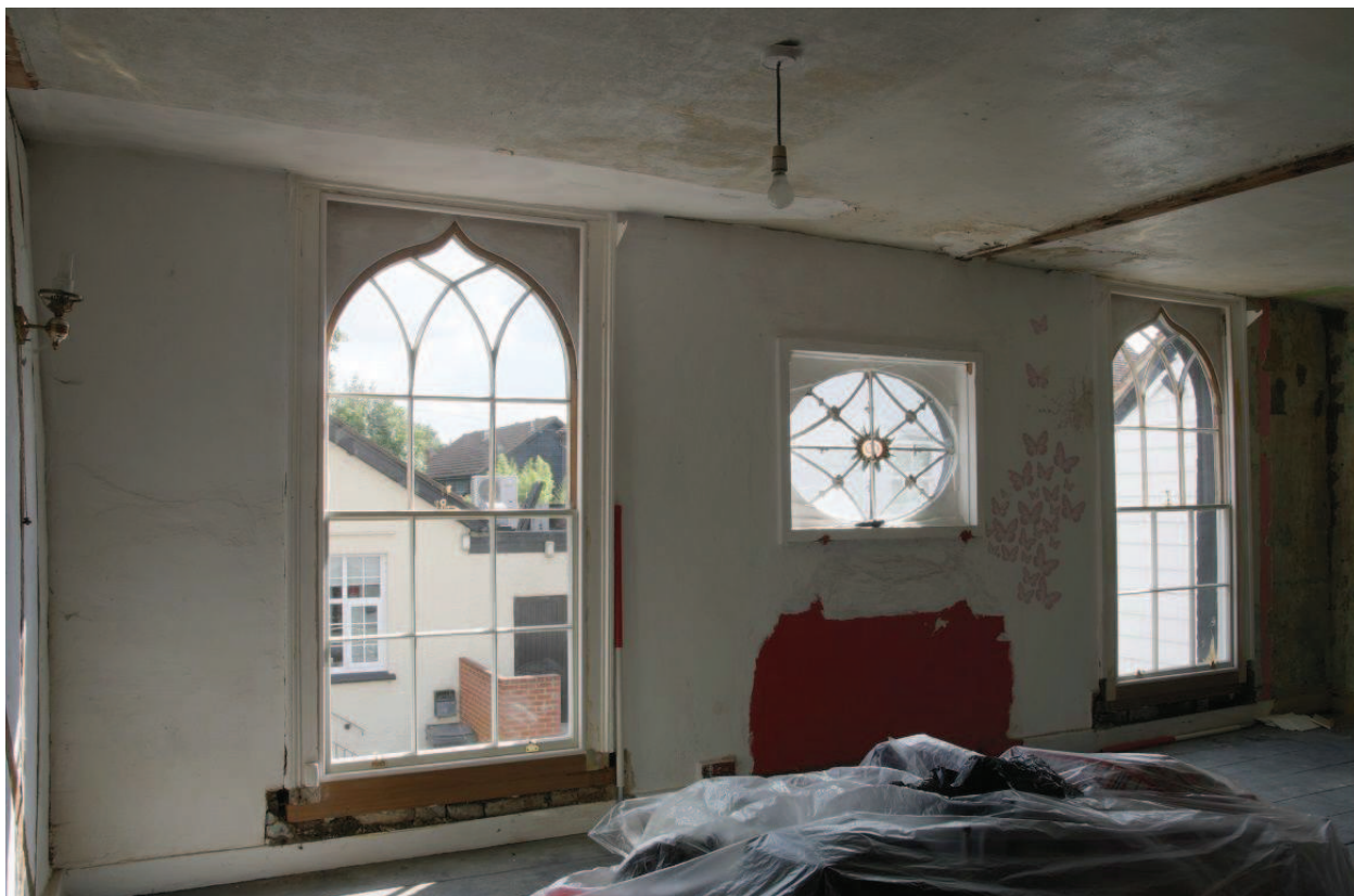
Plate 14 - Bedroom 1, south elevation, looking SW
