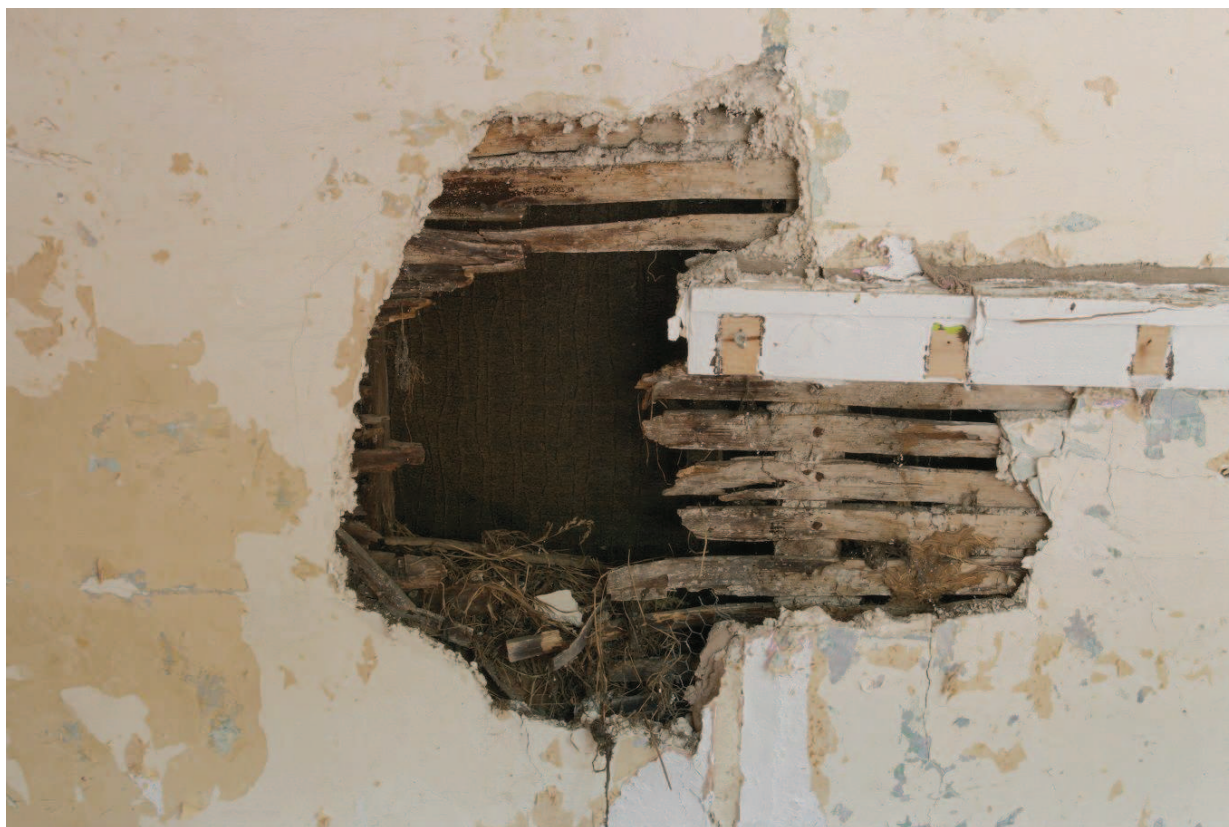
Plate 21 - Bedroom 2, N elevation, exposed laths & stow insulation, looking N
