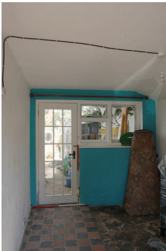
Plate 03 - Dining room, north elevation, looking N
