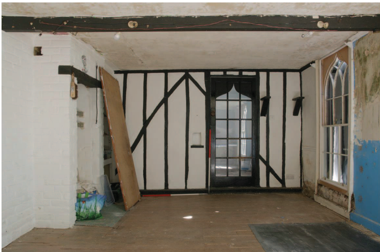
Plate 04 - Living Room, east elevation, looking E
