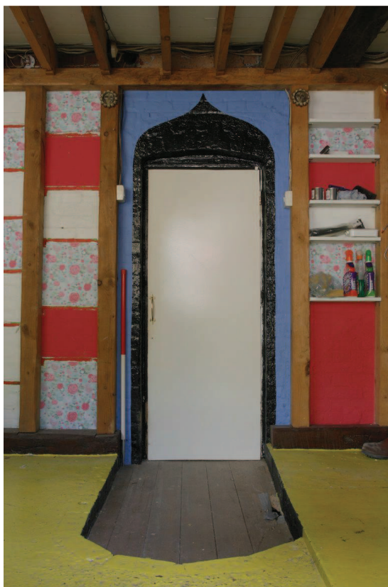
Plate 13 - Kitchen, doorway in S elevation, looking S
