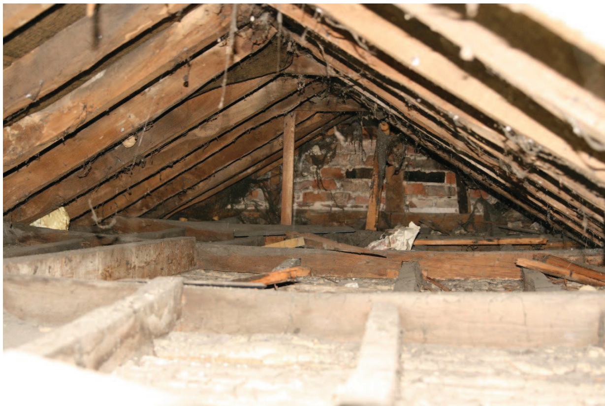
Plate 24 - Roof space, showing exposed brickwork, looking E
