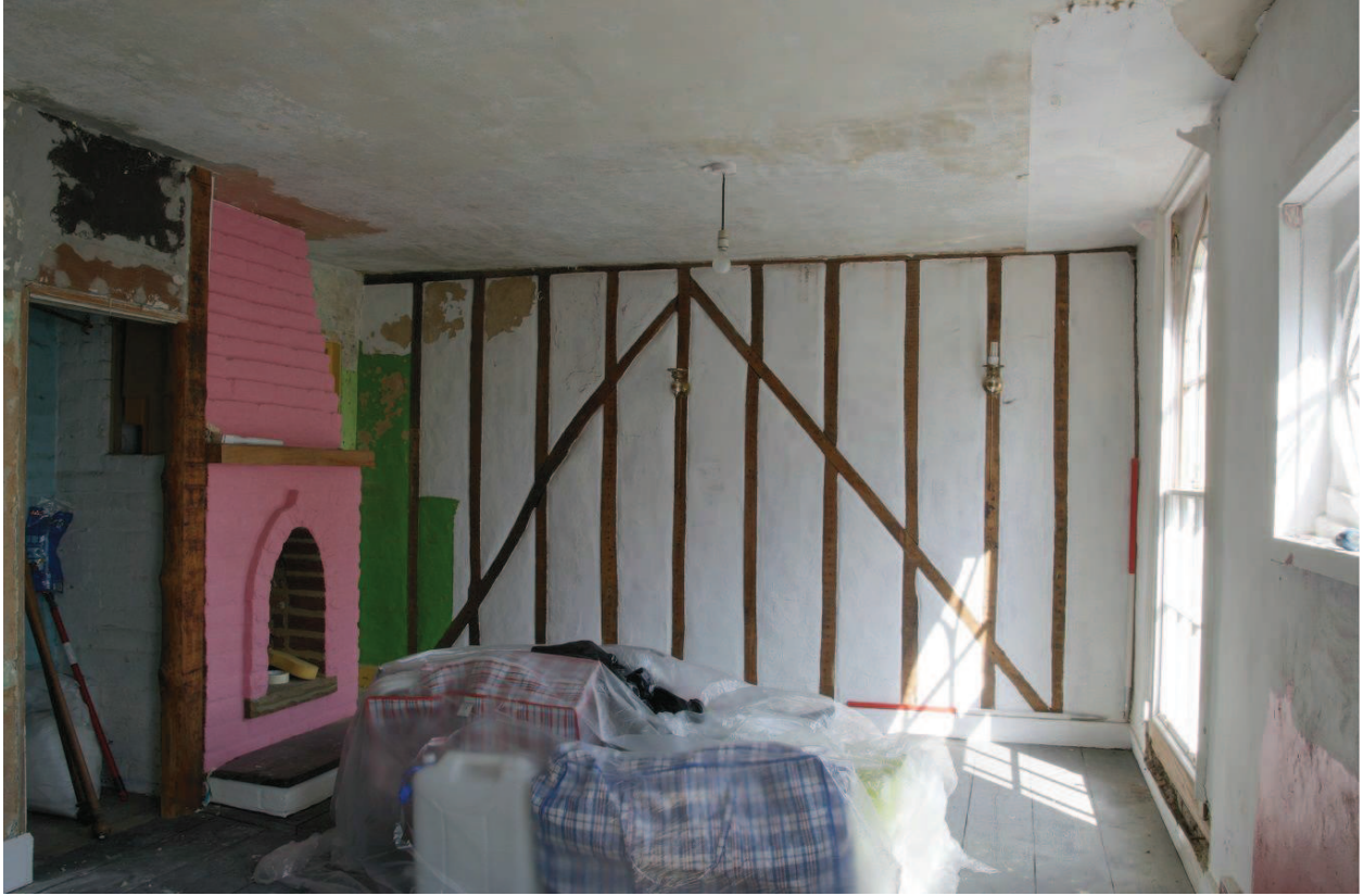
Plate 16 - Bedroom 1, east elevation, looking NE
