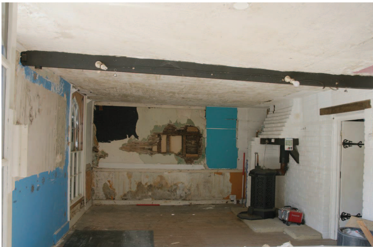
Plate 07 - Living room, west elevation, looking W
