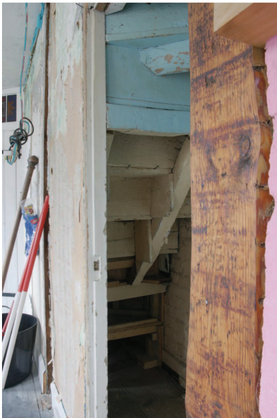
Plate 18 - Bedroom 1, N elevation, cupboard under the stairs, looking W
