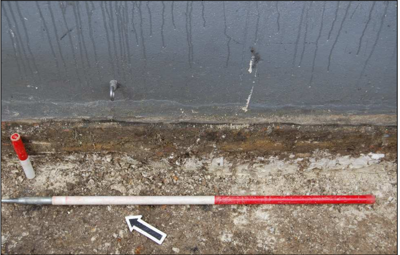
Plate 3: Exposed brickwork resting on natural chalk, looking northeast.
