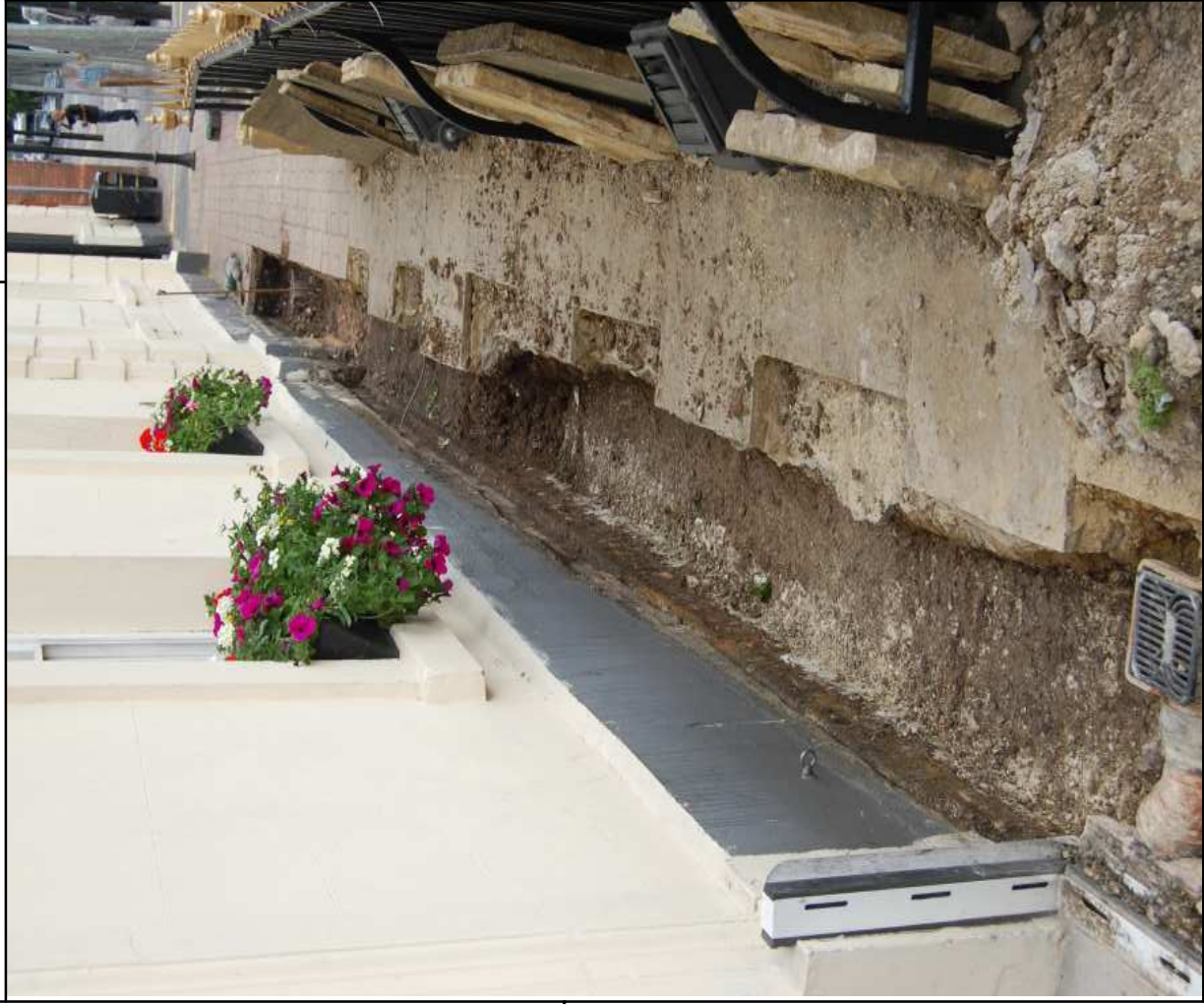
Plate 1: View of French drain, looking southeast.
