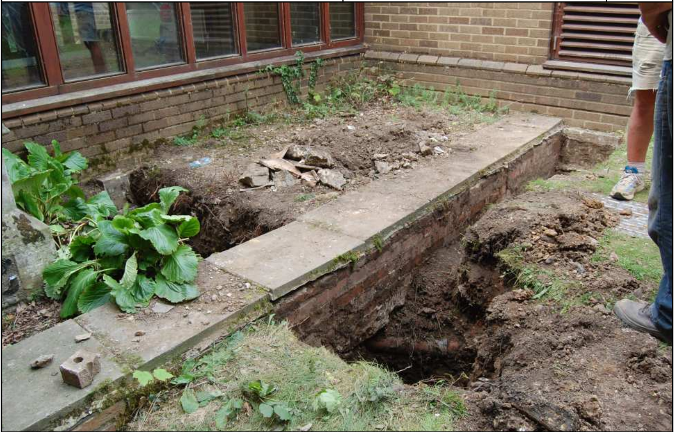
Plate 1: Extension footing, looking northwest.
