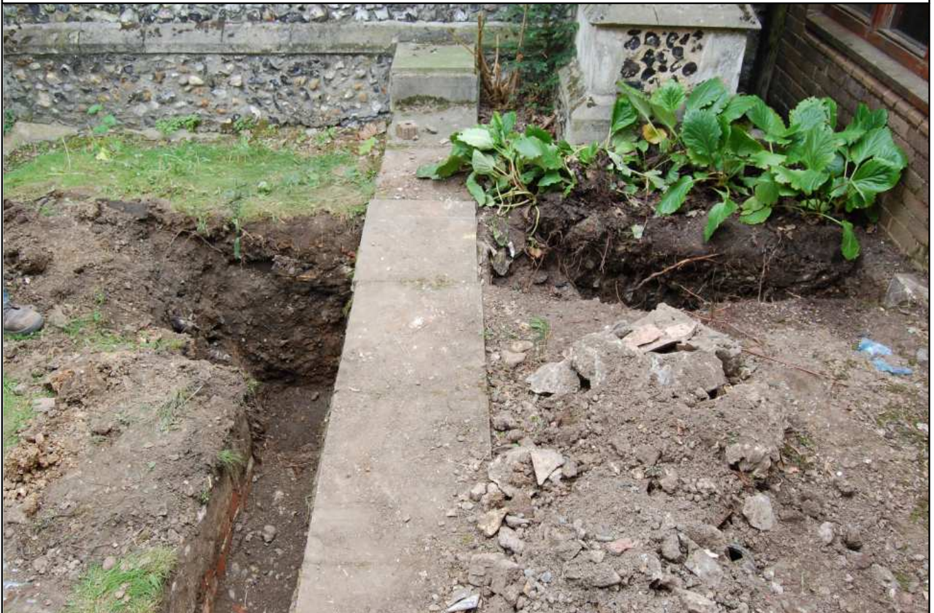
Plate 2: Extension footing, looking south.
