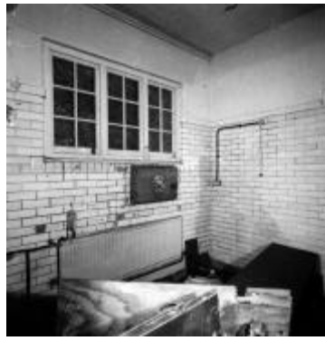
2 Scullery facing south-east
