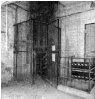
4 Water Tower: south-west corner
