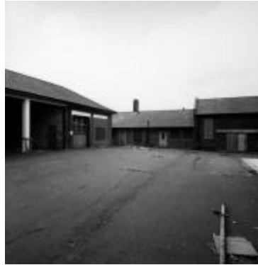
2 North-west corner of the courtyard
