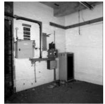
6 Water Tower: north-west corner of the BT machine room
