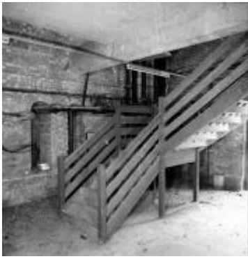
1 Water Tower: stair
