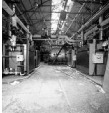
2 Boiler House: general shot facing south
