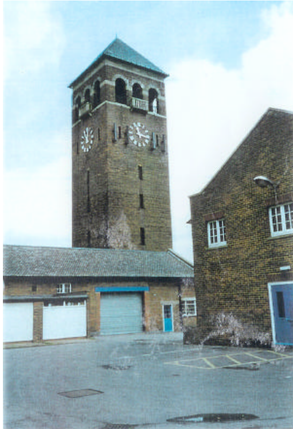
South elevation of the Old Bakery showing an extension, now demolished
