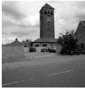
8 Water Tower: west elevation
