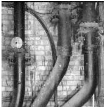
10 Water Tower: pipework detail
