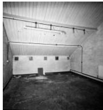
5 First Floor Office facing south
