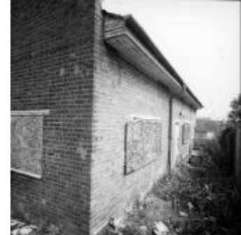
9 Works Office facing north-east
