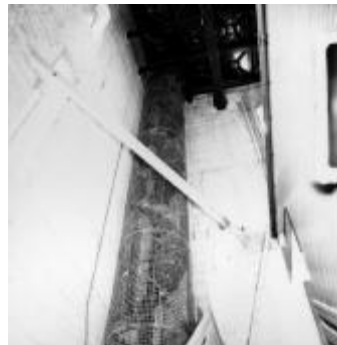
11 Water Tower: upper level of spiral stairs
