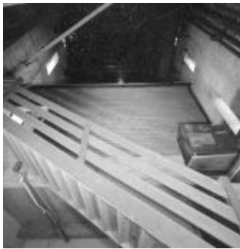
4 Water Tower: tanks & mezzanine from the south
