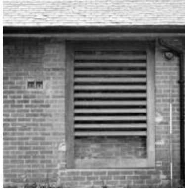
2 Engineer's Block: south elevation louvered window detail
