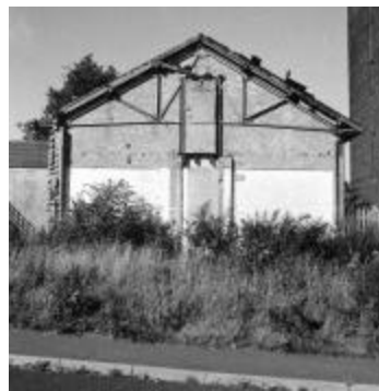
5 Works Office: east elevation
