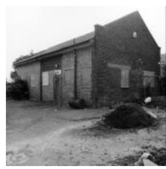
12 Works Office from the north-west
