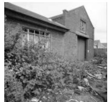
12 West Range: door to the Old Bakery
