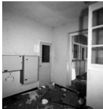
11 Reception facing west
