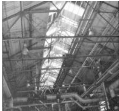
1 Boiler House: roof truss
