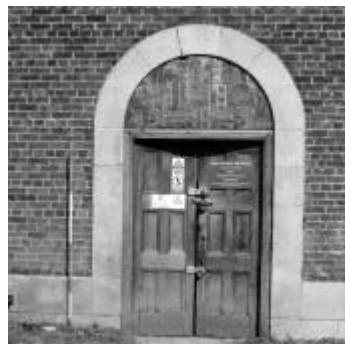
11 Water Tower: door detail
