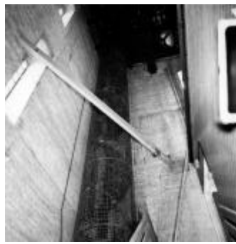
8 Water Tower: spiral staircase from the east
