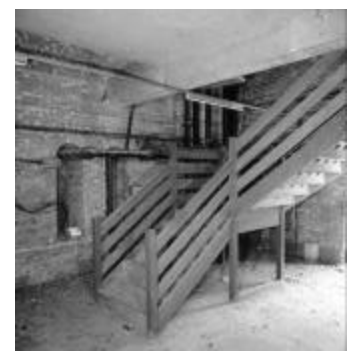
12 Water Tower: stair
