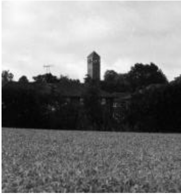
1 Water Tower from the brideway
