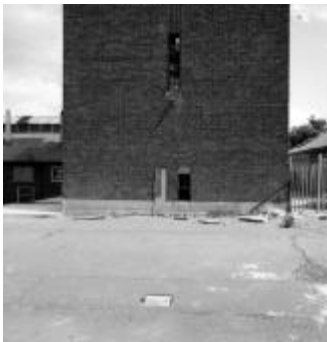
4 Water Tower: base of the west elevation
