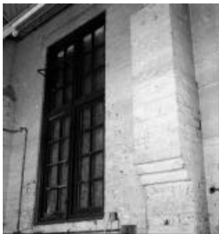
10 Engineer's Block: workshop window & buttress detail
