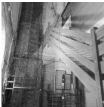
10 Water Tower: spiral staircase & stair to mezzanine
