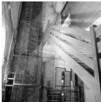
11 Water Tower: spiral staircase & stair to mezzanine
