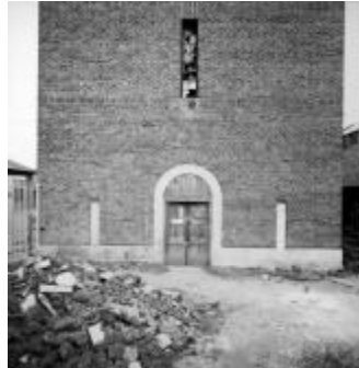
8 Water Tower: south elevation
