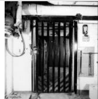
9 Boiler House: gate to switch room
