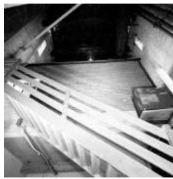
5 Water Tower: tanks & mezzanine from the south
