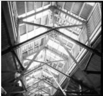
7 Boiler House: roof truss from gantry
