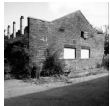
9 Boiler House: south elevation
