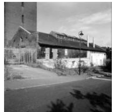
6 Boiler House: south & east elevation
