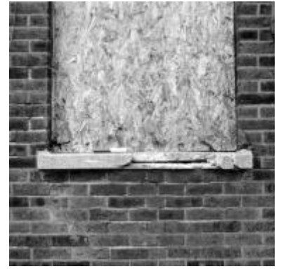
3 Engineer's Block: south elevation window detail
