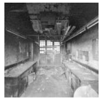
12 West Range: workshop interior facing east
