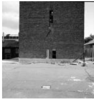
5 Water Tower: base of the west elevation
