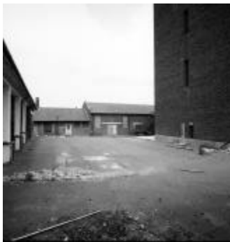
4 Courtyard from the south-west
