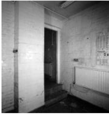
2 Engineer's Block: store facing north-west
