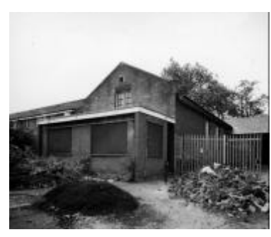
12 Reception & Old Bakery from the north-east
