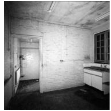
3 Engineer's Block: kitchen facing west
