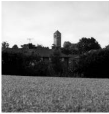
2 Water Tower from the brideway
