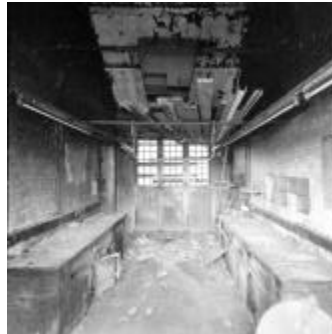
11 West Range: workshop interior facing east
