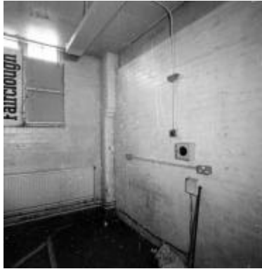
1 Engineer's Block: office facing north-east
