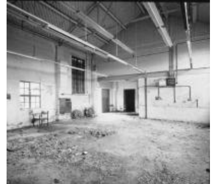
12 Workshop: general shot facing north-east
