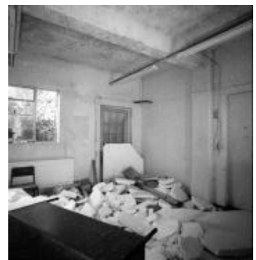
3 Partitioned Office facing south-west
