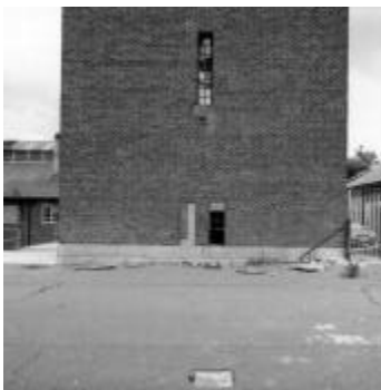
10 Water Tower: base of the west elevation
