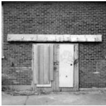
4 Engineer's Block: south elevation door detail
