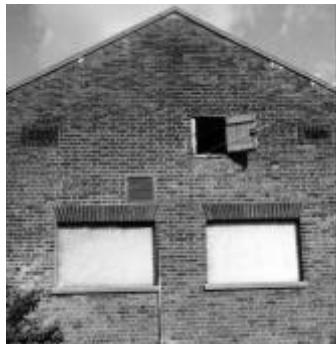
10 Boiler House: south elevation
