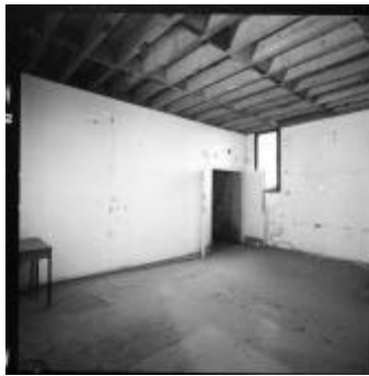
7 Water Tower: mezzanine room
