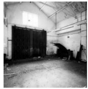
9 Old Bakery facing north-west
