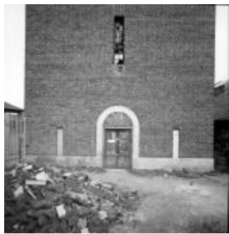
7 Water Tower: south elevation
