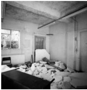
2 Partitioned Office facing south-west
