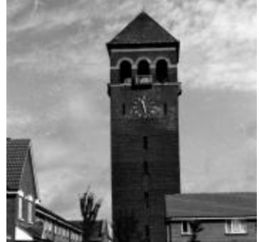
12 Water Tower: south elevation
