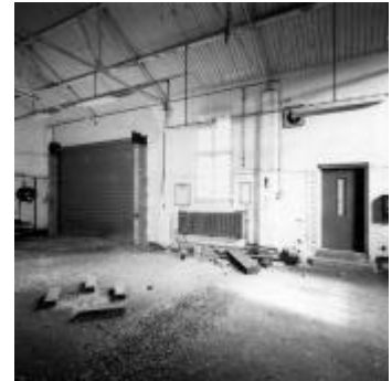
6 Old Bakery facing south-east
