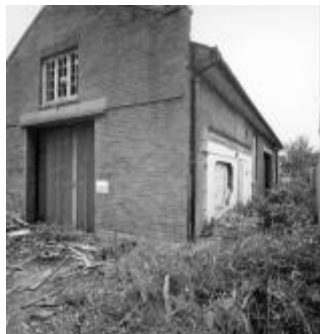
10 South-west corner of the complex
