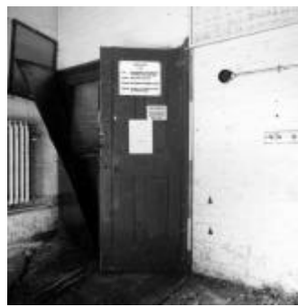
11 Engineer's Block: door to office
