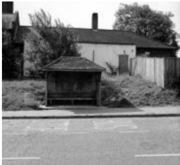
7 Electricity Sub-station: north elevation
