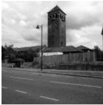
7 Water Tower from the north-west
