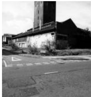
5 Boiler House from the north-east
