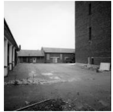
3 Courtyard from the south-west
