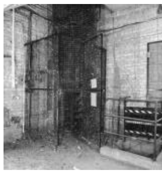
5 Water Tower: south-west corner
