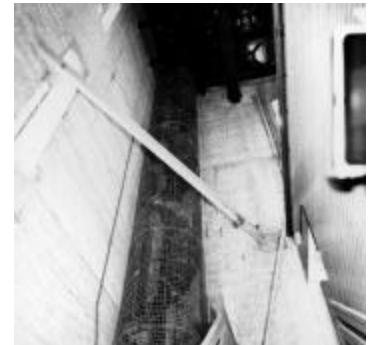
12 Water Tower: upper level of spiral stairs
