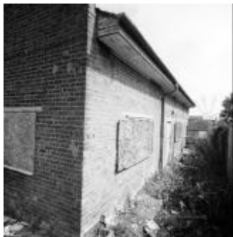
10 Works Office facing north-east
