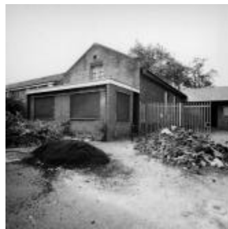
11 Reception & Old Bakery from the north-east
