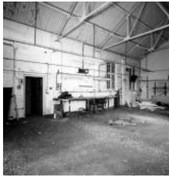
5 Old Bakery facing north-east
