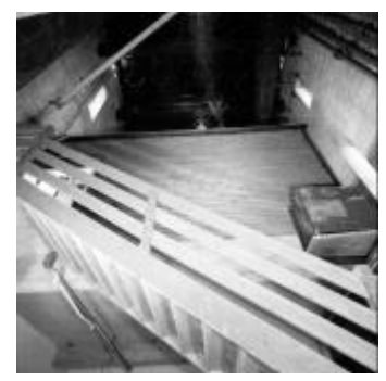
6 Water Tower: tanks & mezzanine from the south
