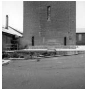
2 Water Tower: base of the north elevation
