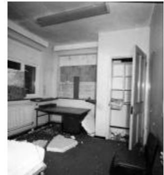
12 Rear office facing south-west
