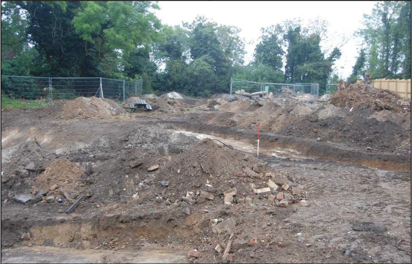
Plate 1: General view of the site, looking north.
