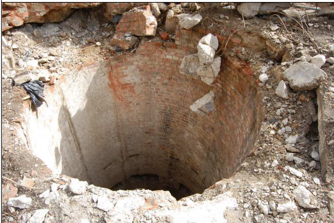
Plate 14: Pump shaft, looking south.
