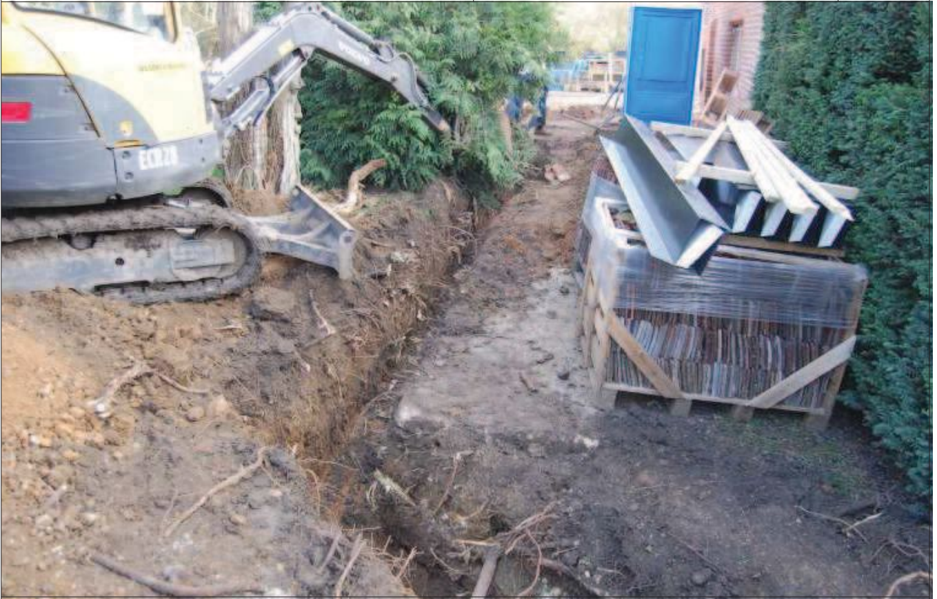
Plate 11: Drainage 1 trench looking southwest
