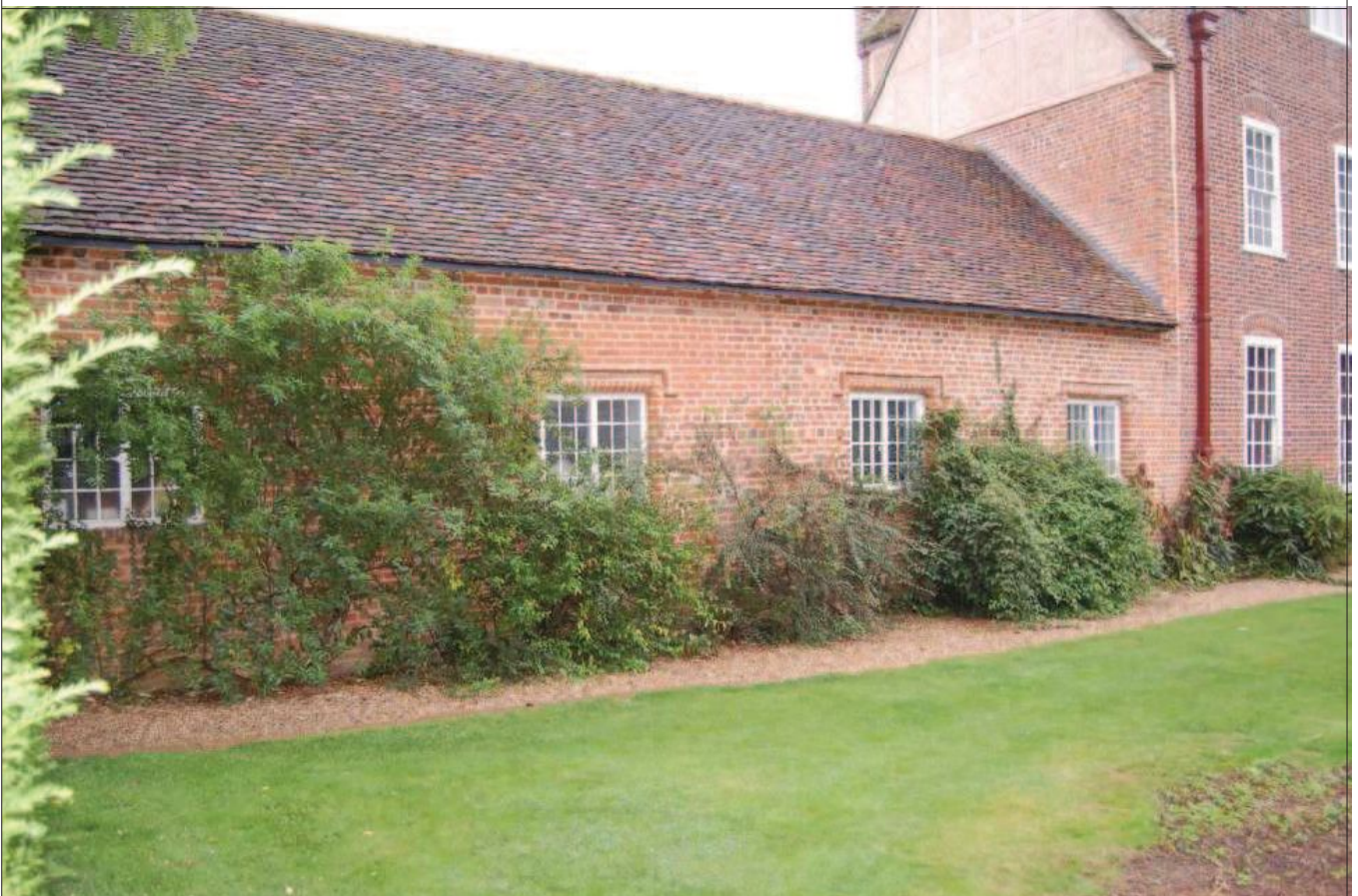
Plate 2: West wing prior to groundworks, looking southeast
