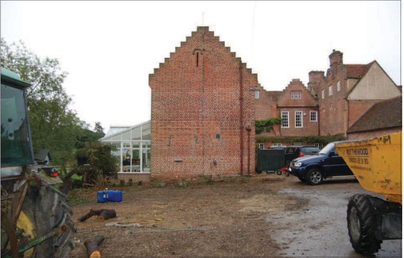
Plate 1: East wing prior to groundworks, looking south
