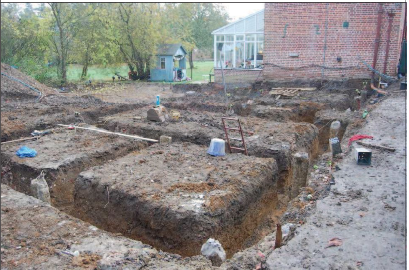
Plate 6: Eastern extension ground beam trenches, looking southeast
