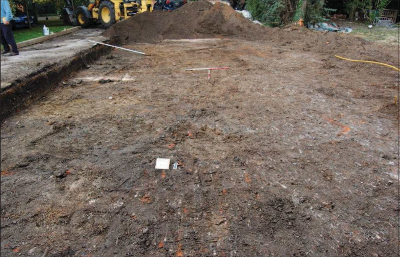
Plate 3: Eastern extension after initial strip, looking north
