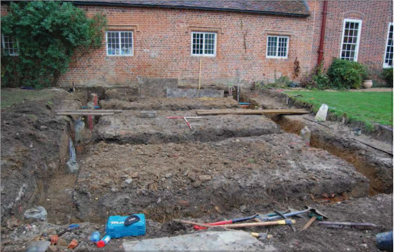
Plate 5: Ground beam trenches for Garden Room, looking east
