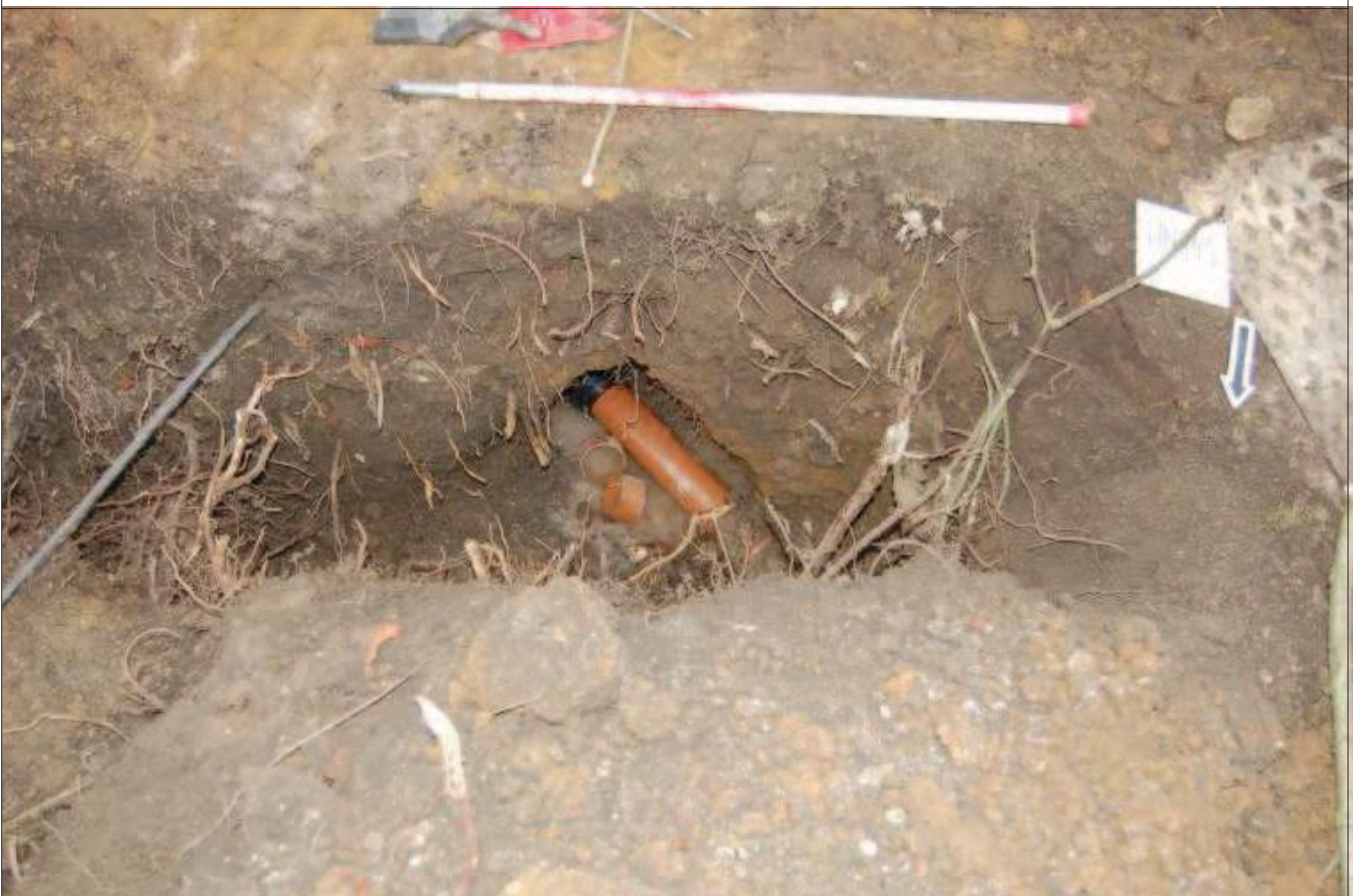
Plate 12: Drainage trench 2 looking south
