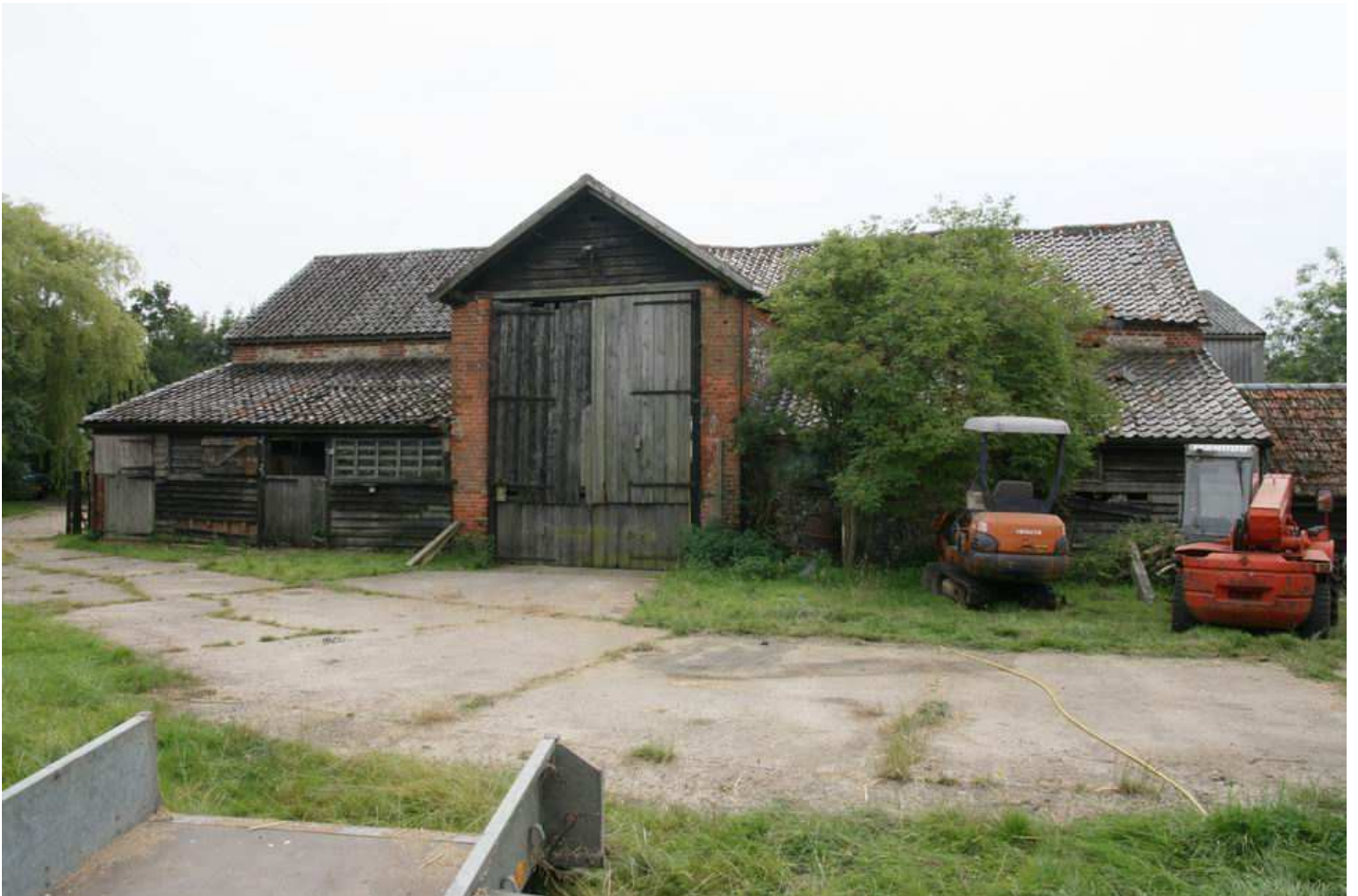
Plate 04 - Buildings 1 to 4, NW elevation
