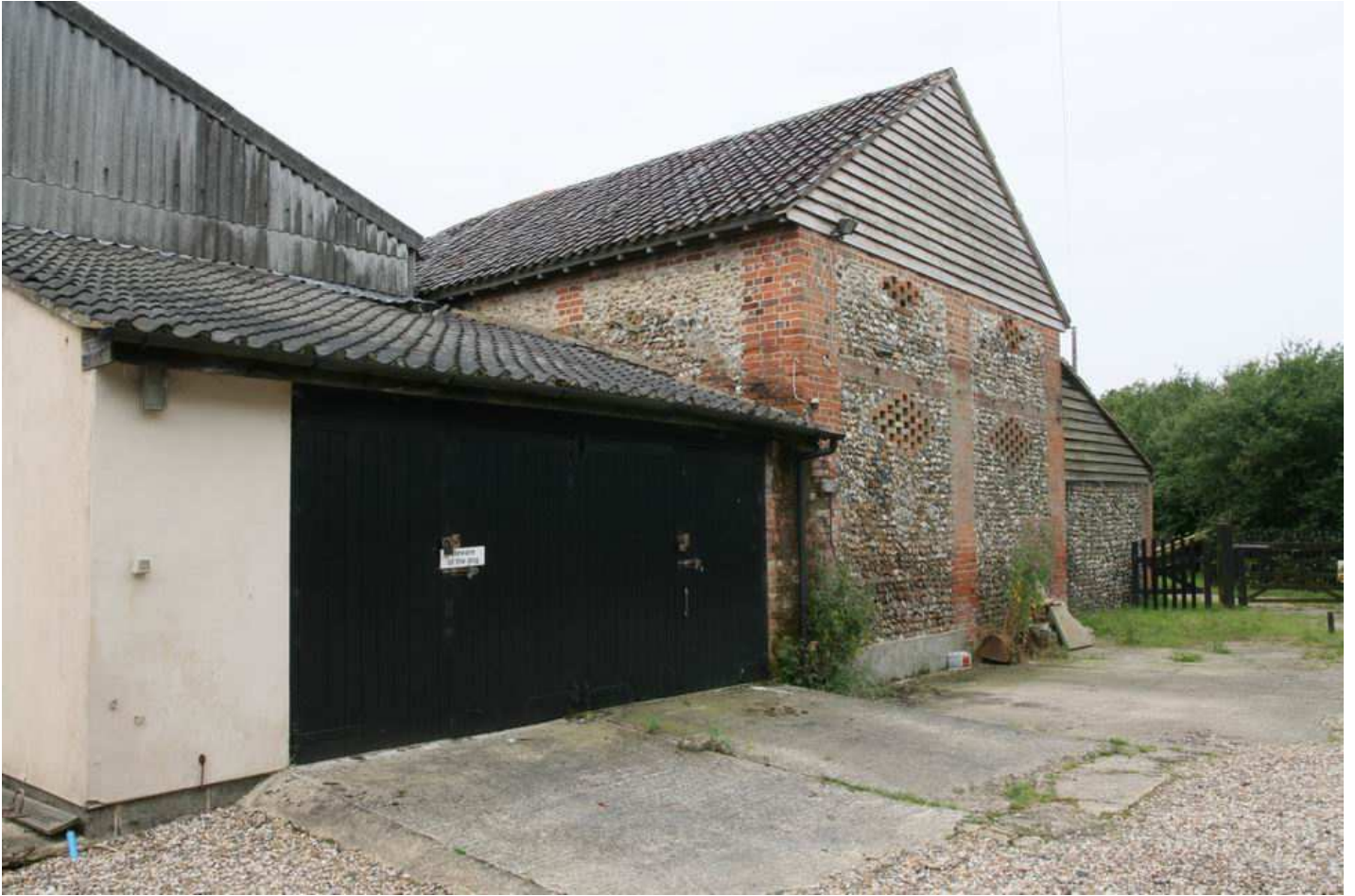
Plate 03 - Building 6, NE elevation
