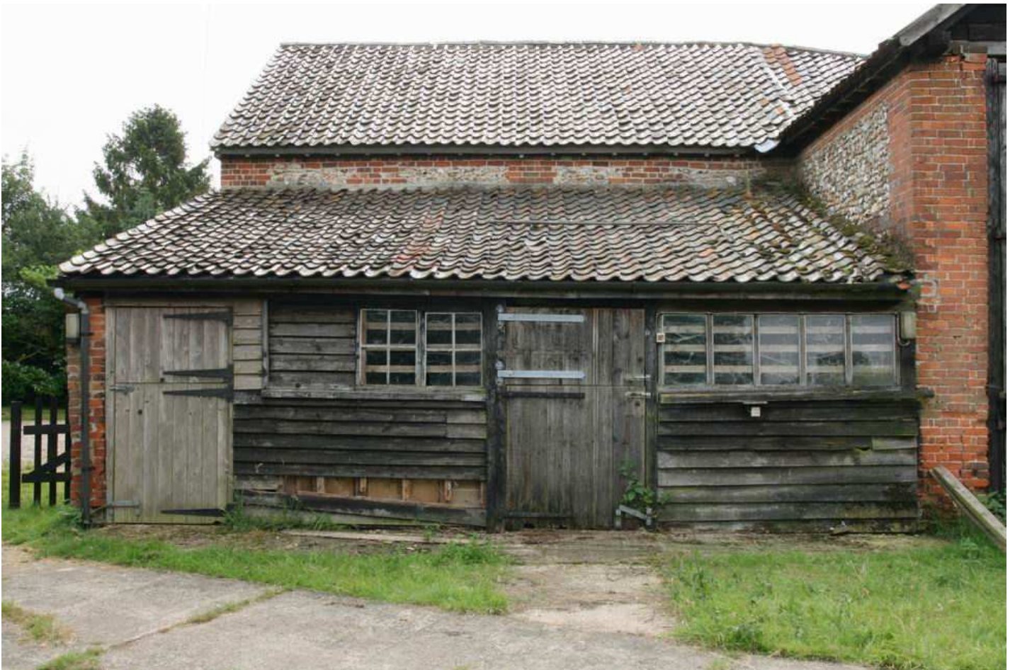
Plate 06 - Building 2, NW elevation
