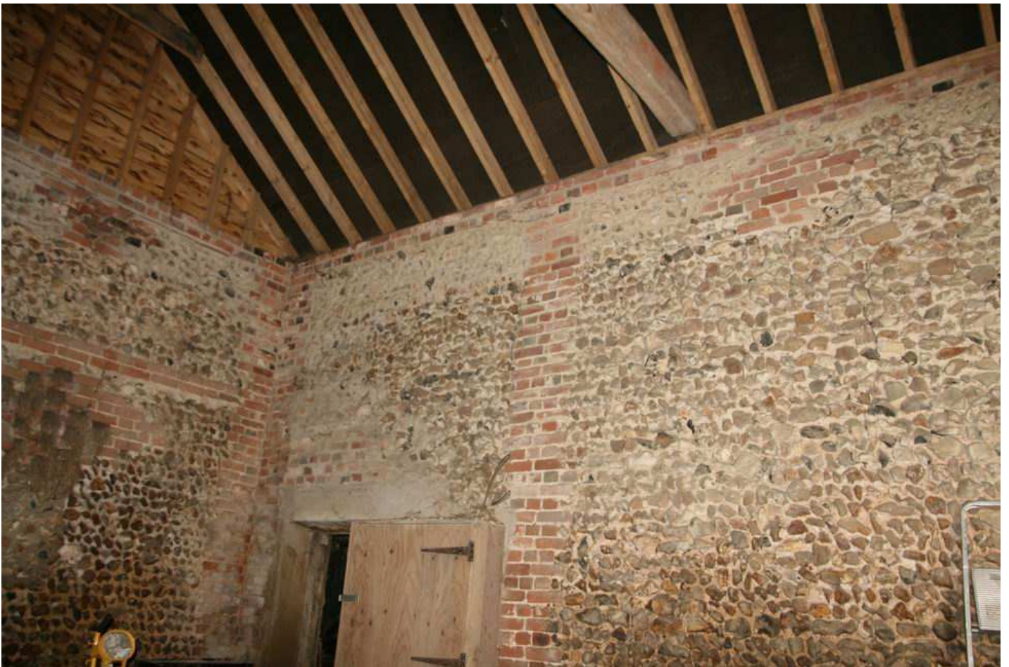
Plate 20 - Building 1, NE corner
