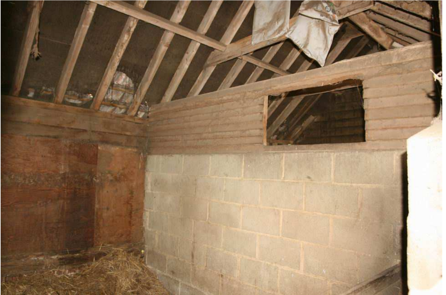
Plate 29 - Building 5, partition between Bays 3 & 4
