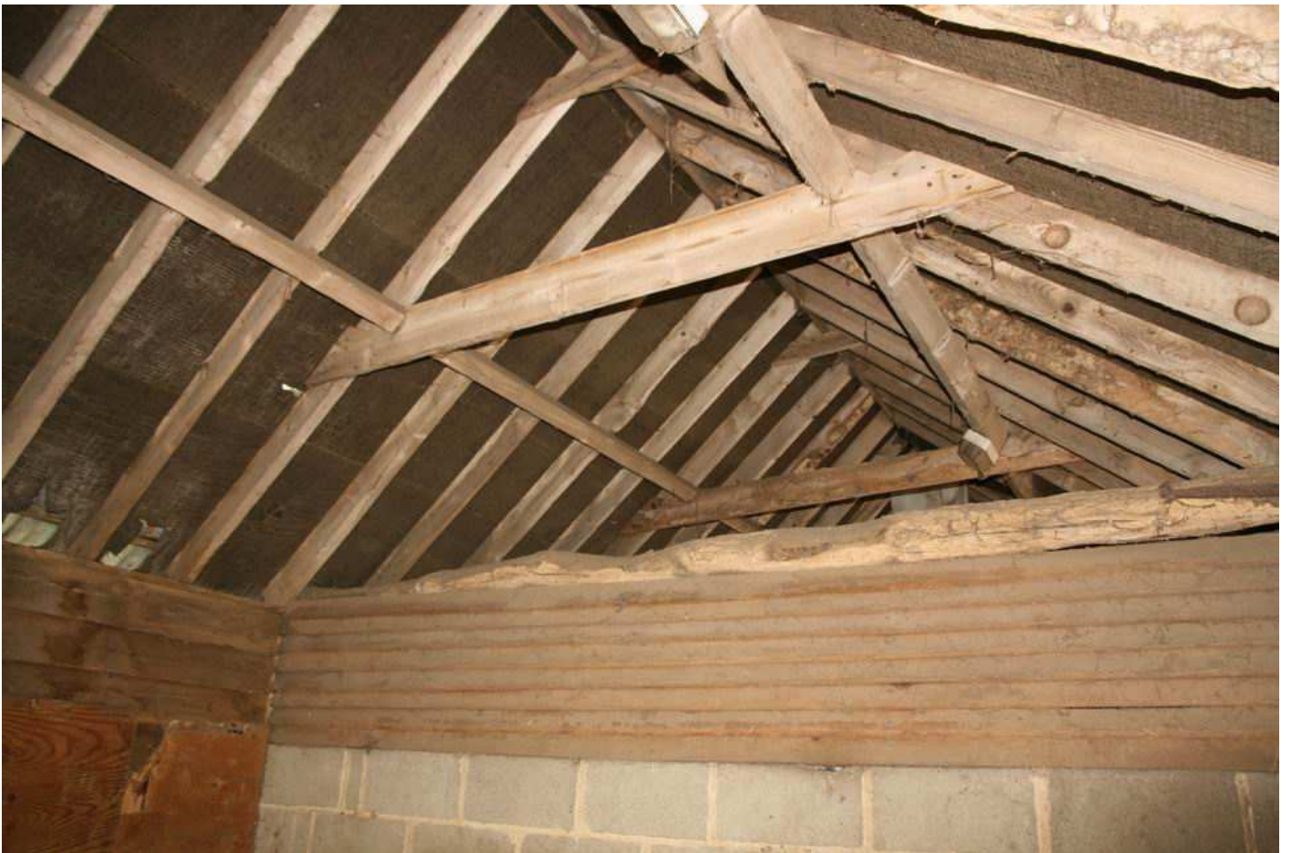
Plate 30 - Building 5, roof structure
