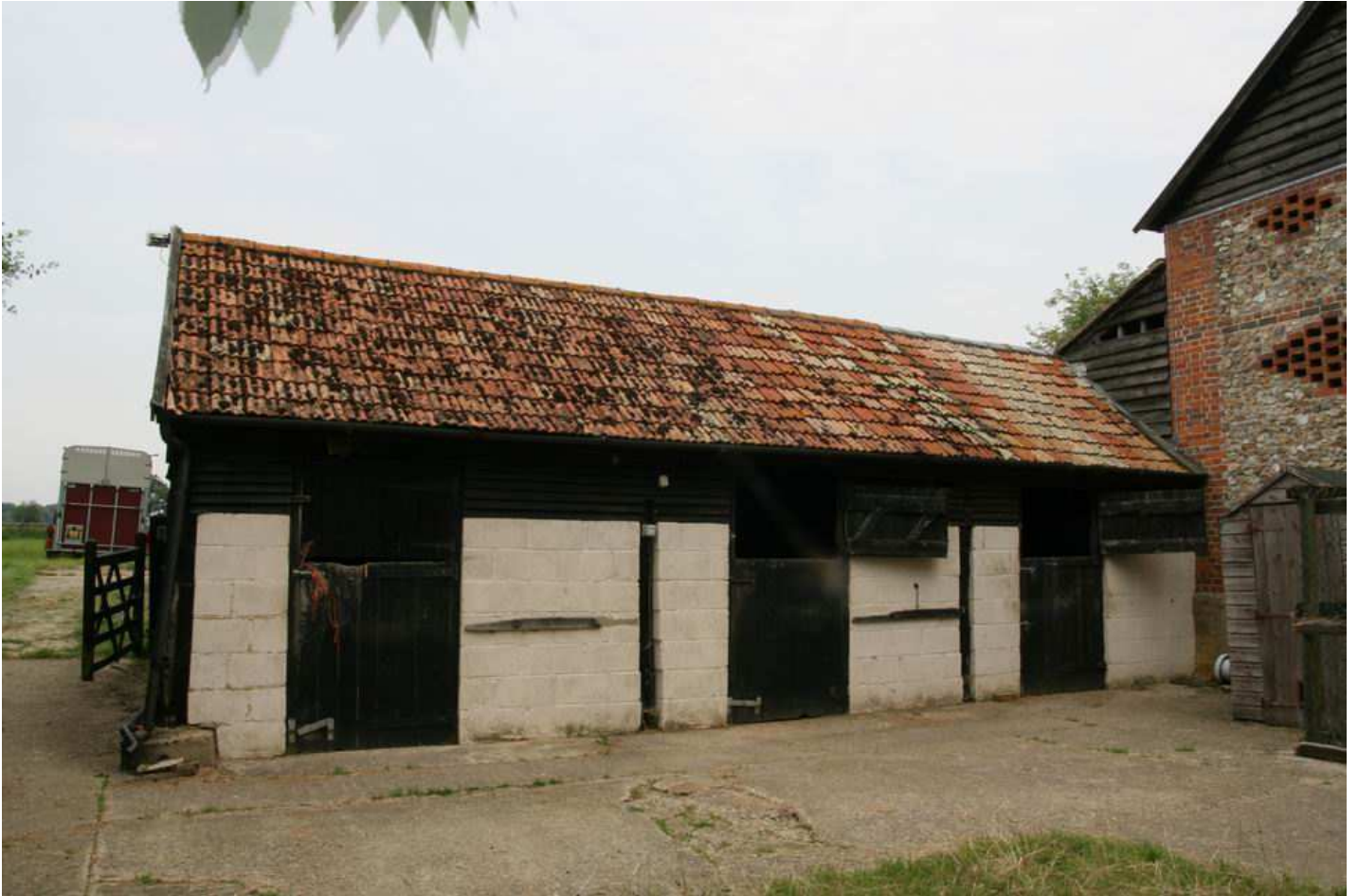
Plate 11 - Building 5, SE elevation
