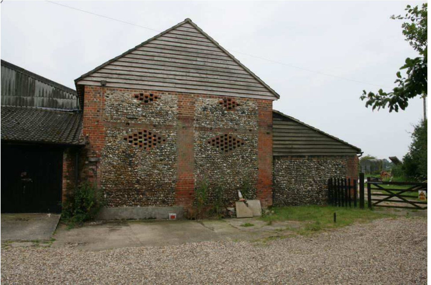
Plate 01 - Building 1, NE elevation
