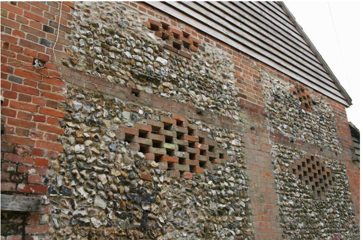
Plate 02 - Building 1, detail of ventilation panels, NE elevation
