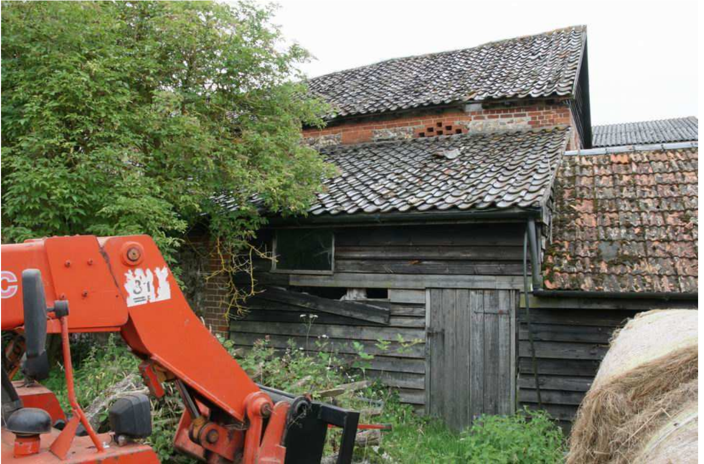
Plate 09 - Building 4, NW elevation
