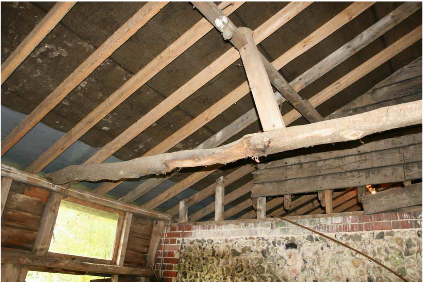
Plate 28 - Building 4 roof structure
