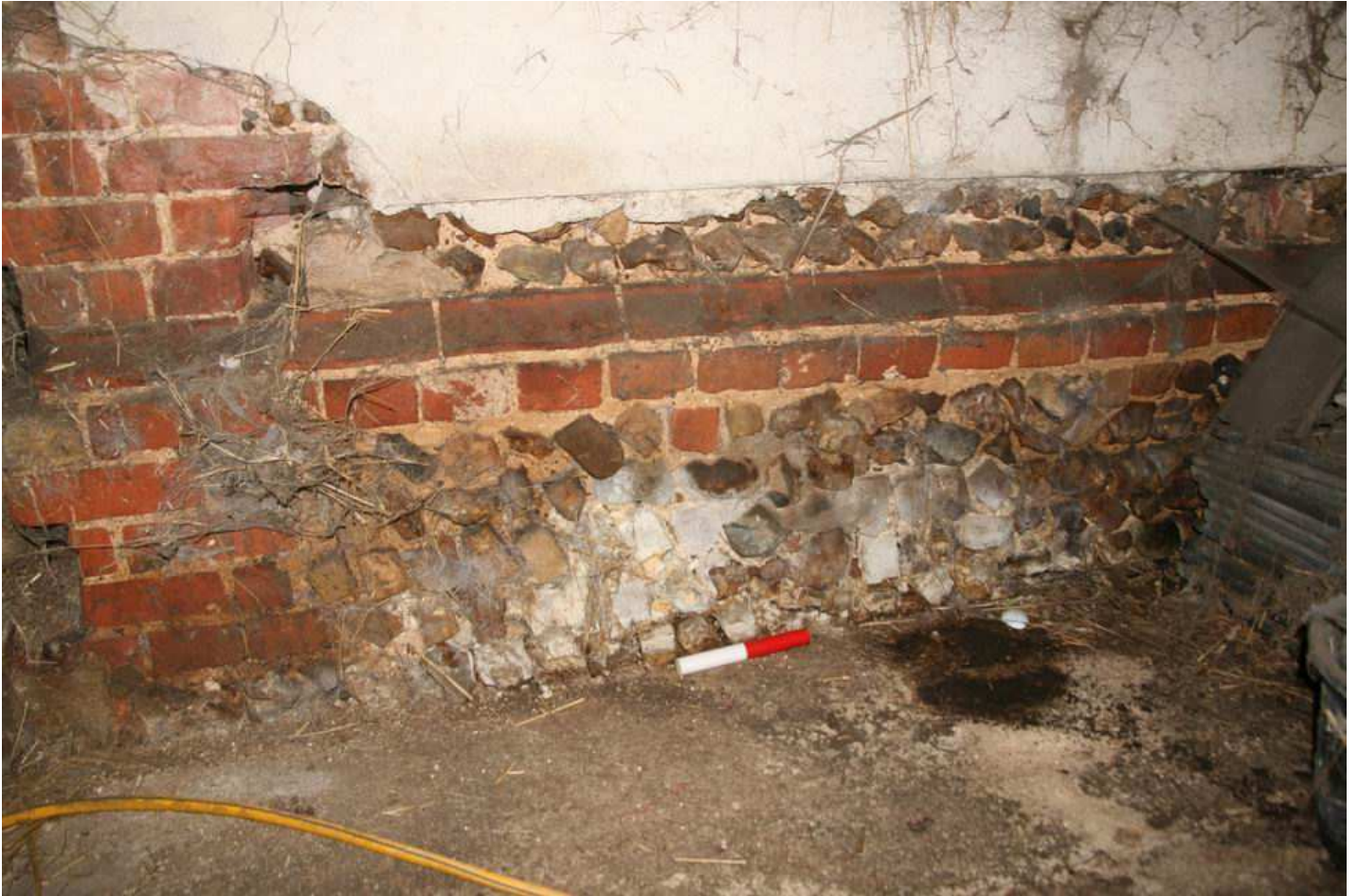
Plate 13 - Building 1, plinth detail SE elevation,
