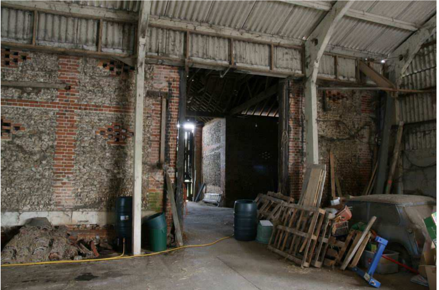
Plate 15 - Building 1, SE elevation (N end)
