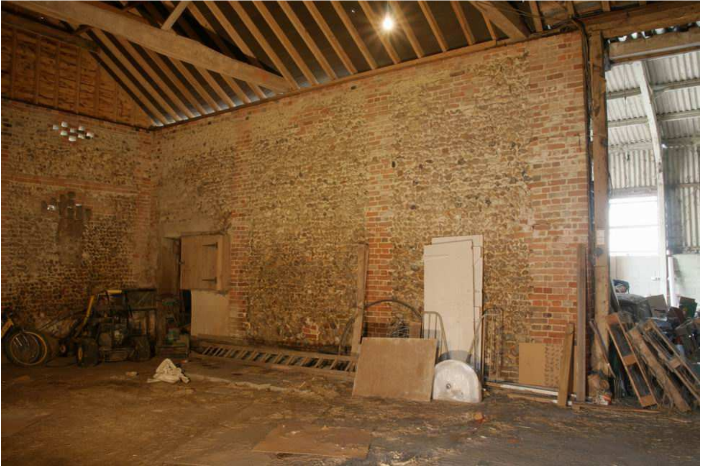
Plate 19 - Building 1, SE interior elevation (N end)
