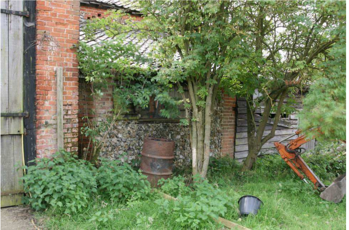
Plate 07 - Building 3, NW elevation
