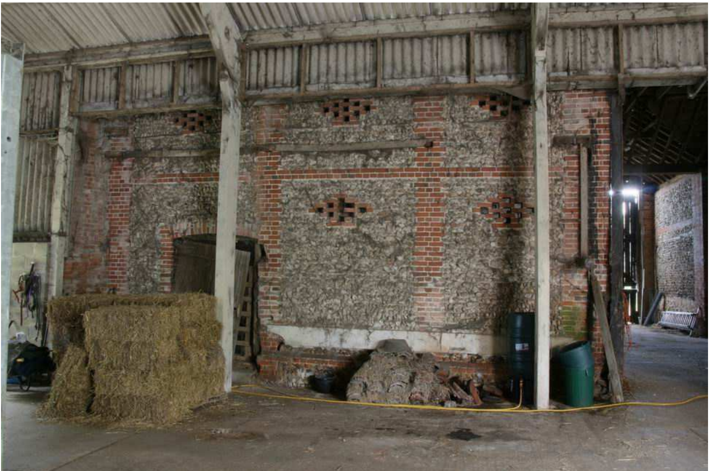
Plate 14 - Building 1, SE elevation (S end)
