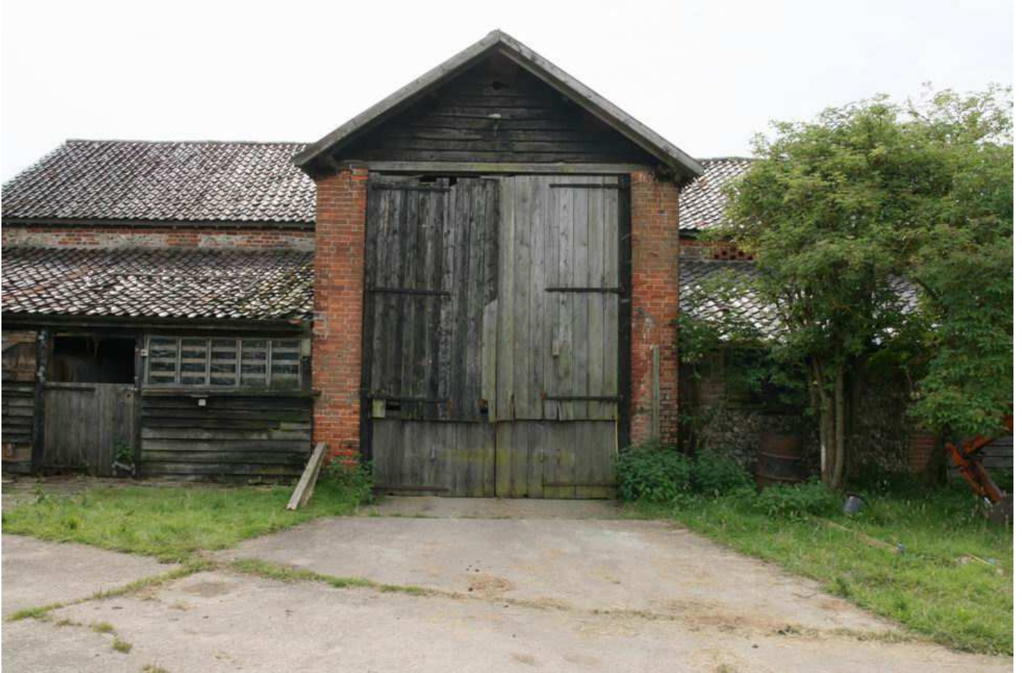
Plate 05 - Building 1, midstrety looking SE
