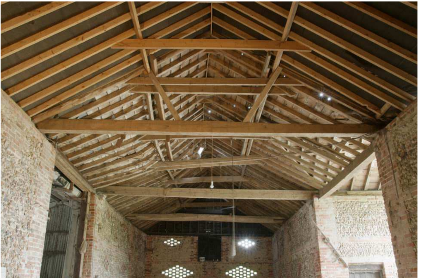
Plate 18 - Building 1 roof structure
