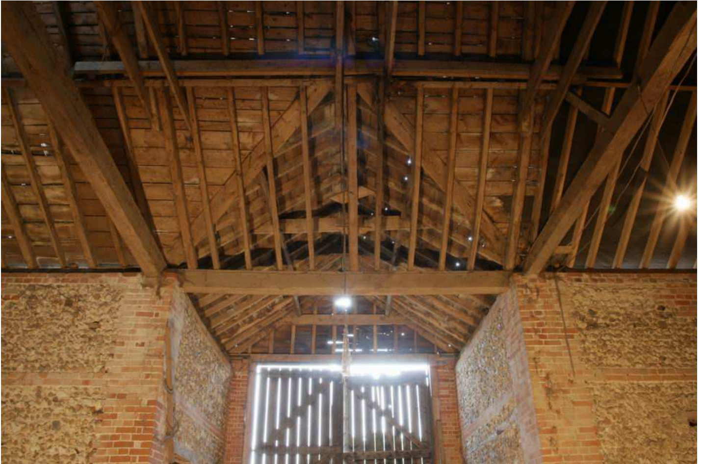
Plate 21 - Building 1, midstrey roof structure
