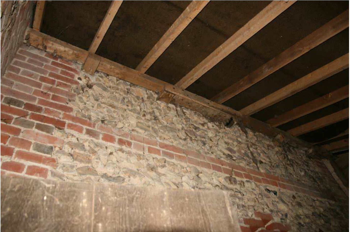
Plate 25 - Building 3 roof structure
