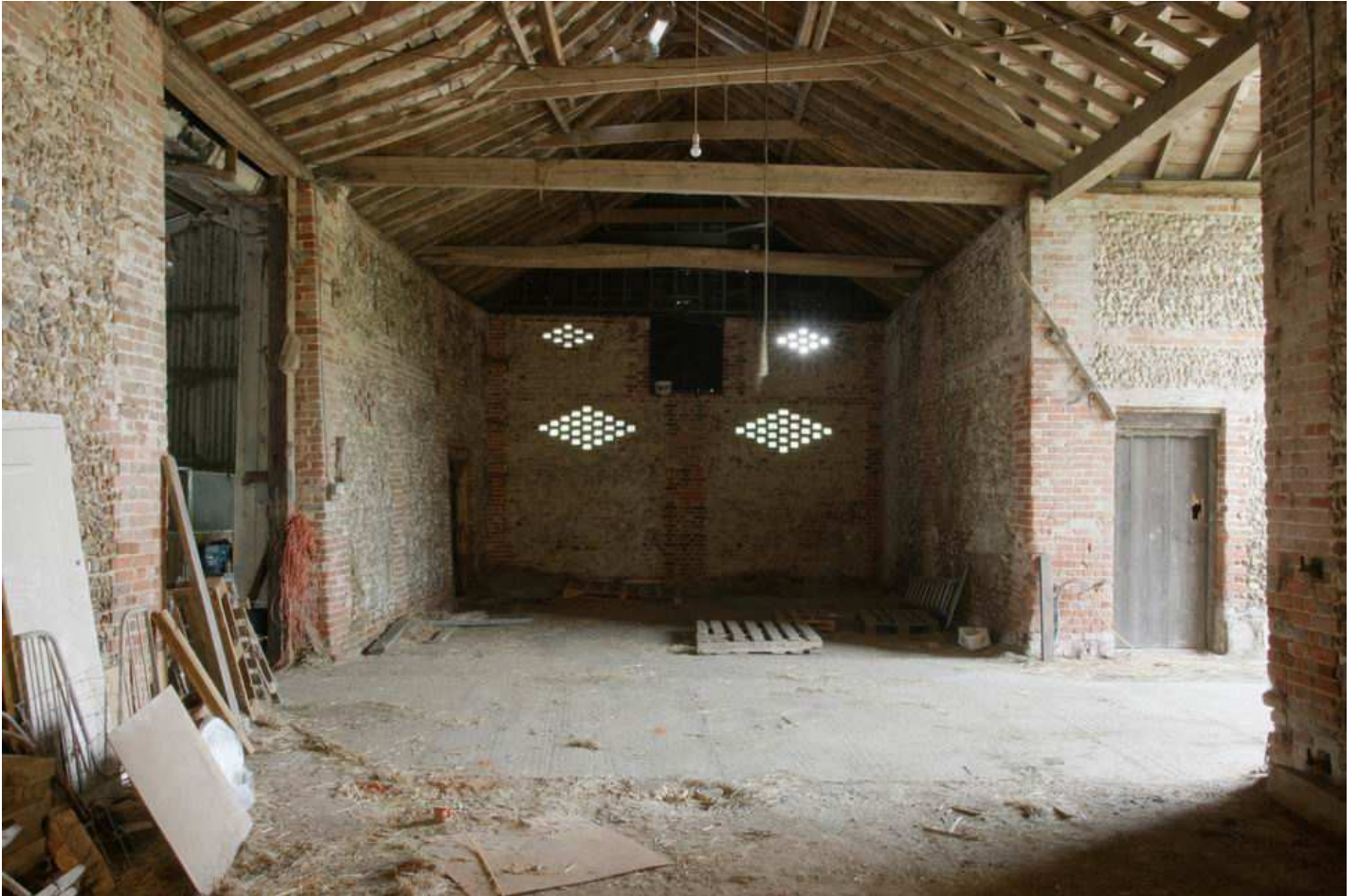
Plate 17 - Building 1, interior looking SW
