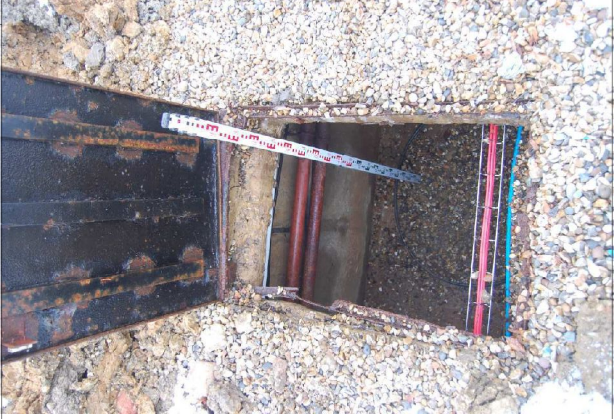
Plate 10: [3301] looking NE into hatch
