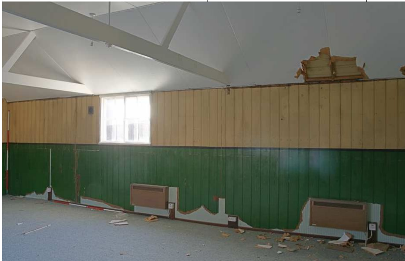
Plate 9: The Hall, south-west interior elevation
