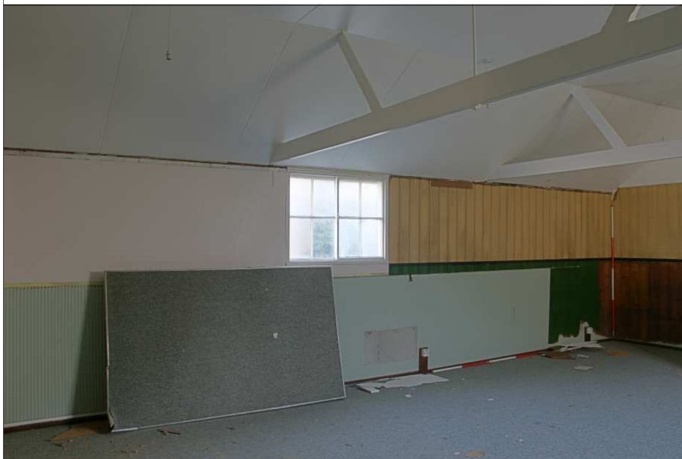
Plate 10: The Hall, north-east interior elevation
