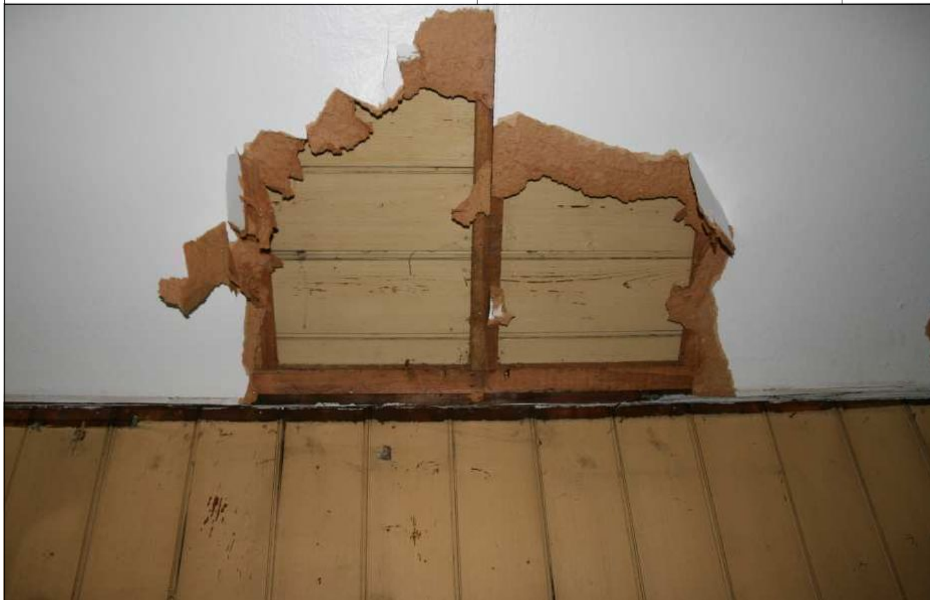
Plate 11: The Hall, detail of ceiling, showing area of panelling below fibre board covering
