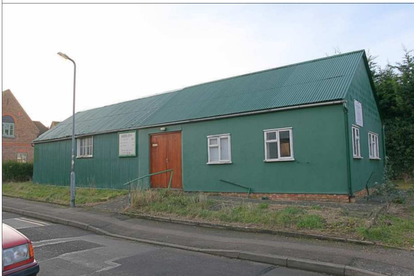
Plate 2: North-east exterior elevation, looking S
