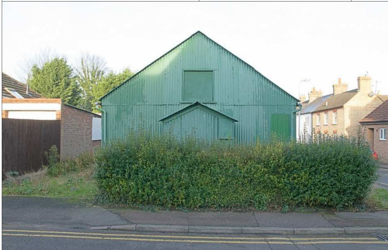
Plate 1: Front (SE) exterior elevation, looking NW
