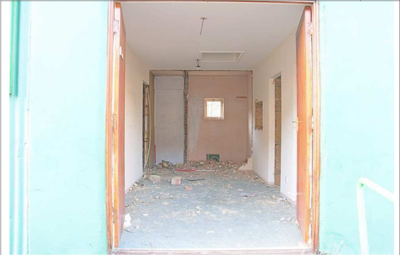
Plate 5: Lobby through main entrance, looking SW
