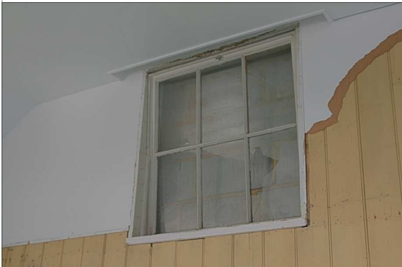
Plate 8: Detail of window in the north-western interior elevation
