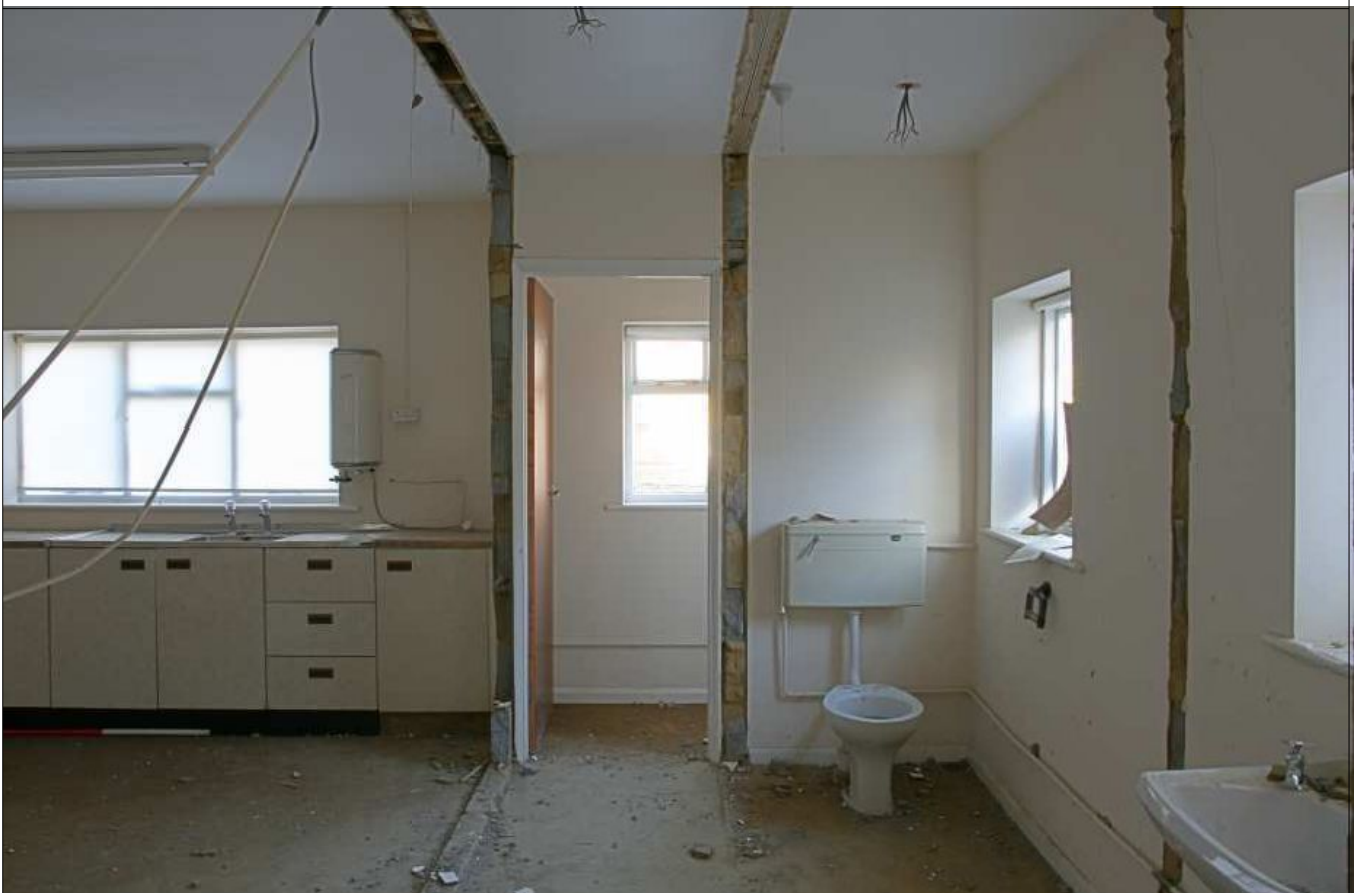
Plate 6: Kitchen & WC to north-west of the lobby
