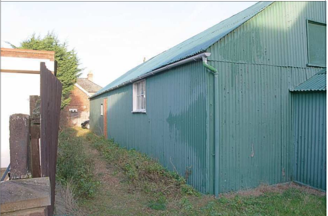
Plate 4: South-west exterior elevation, looking N
