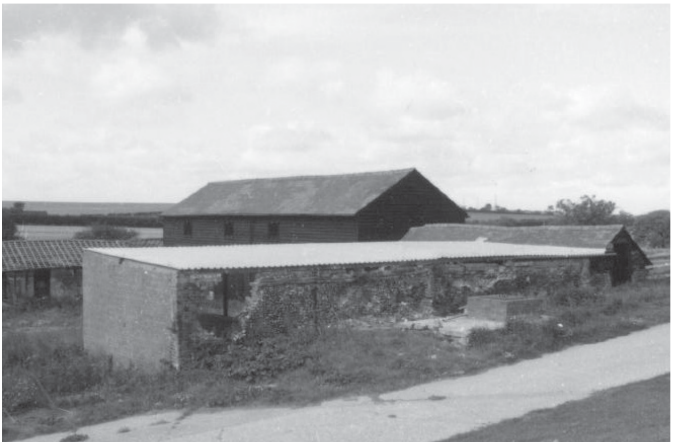
Plate 2b: Barns 1 & 1a, western elevation
