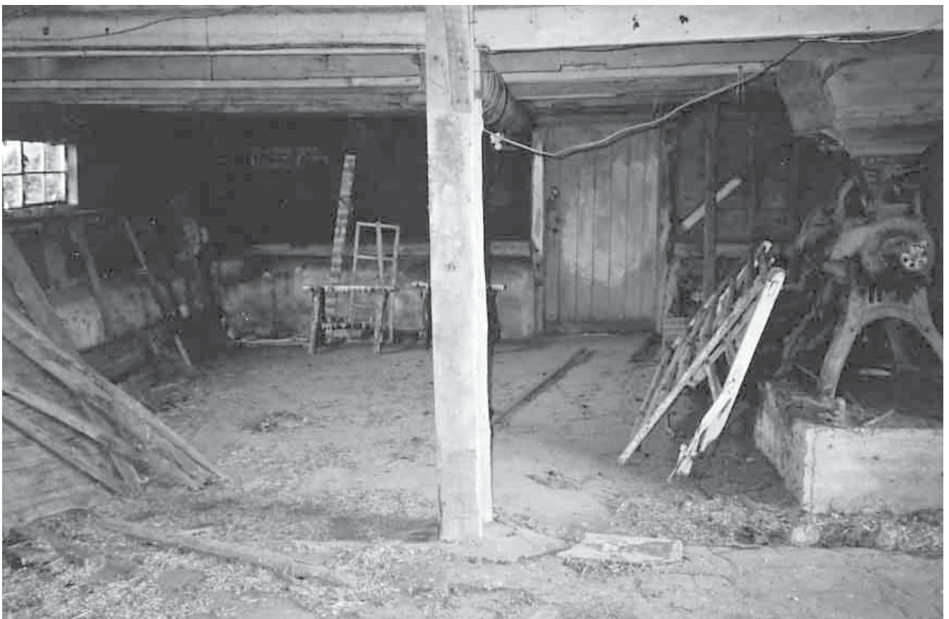
Plate 6b: Barn 2, Bay 1 ground floor before renovation
