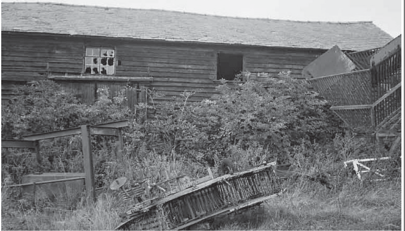
Plate 3a: Barn 2, southern elevation before renovation
