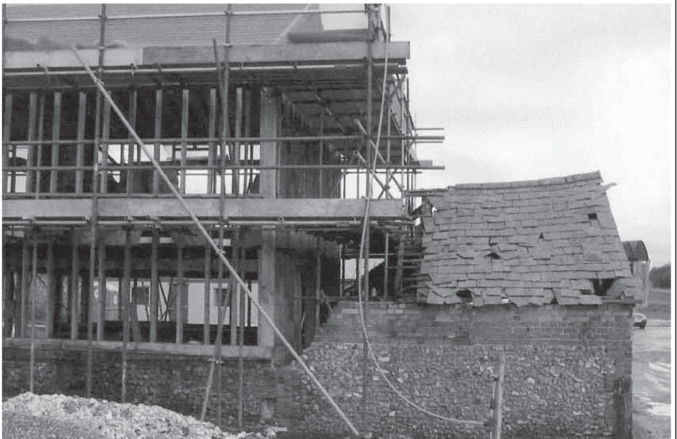
Plate 8b: Barn 3a, junction with Barn 2 during renovation
