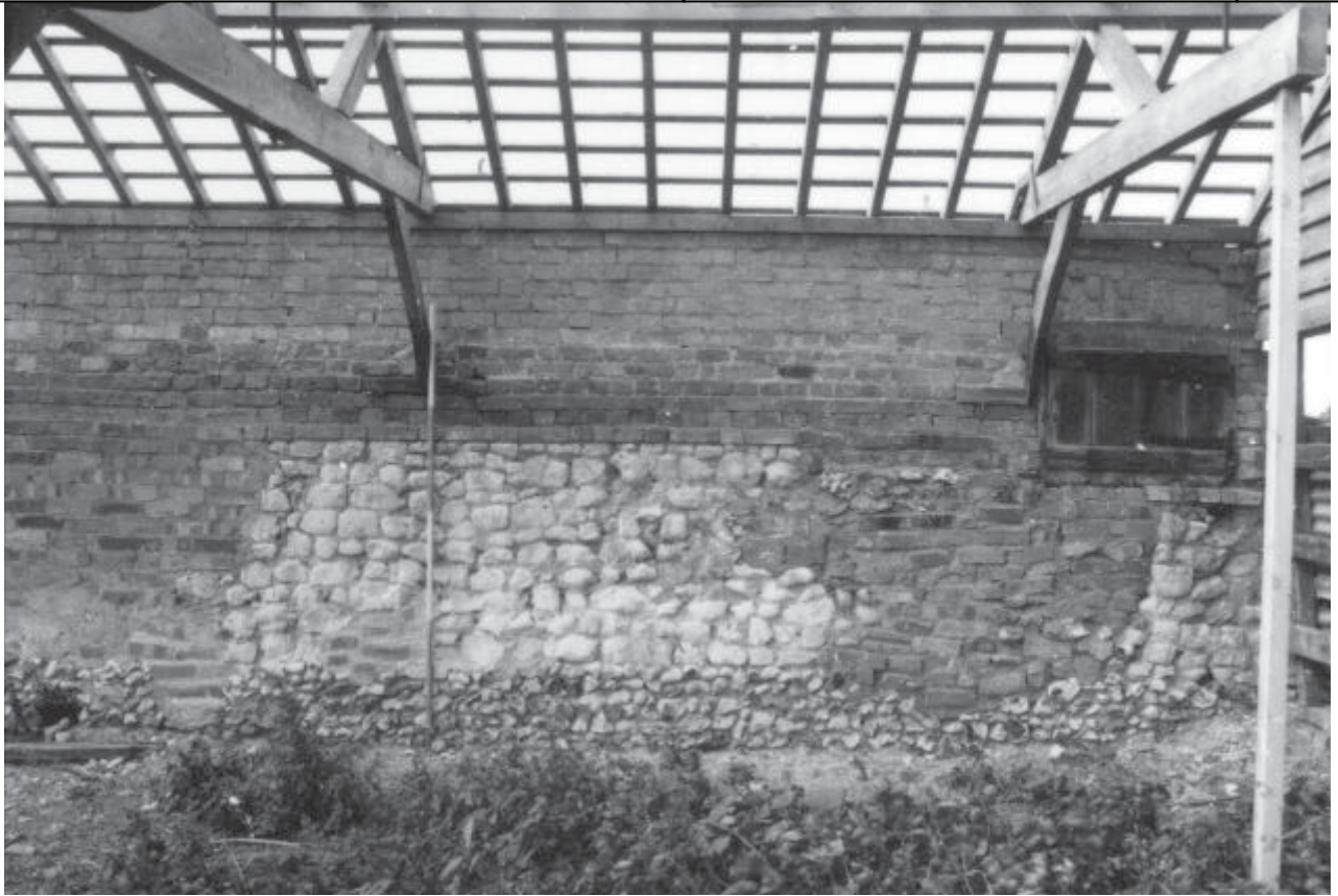
Plate 8a: Barn 3 detail of internal wall construction
