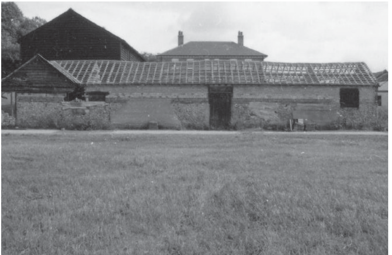
Plate 7b: Barns 3 & 3a, western elevation
