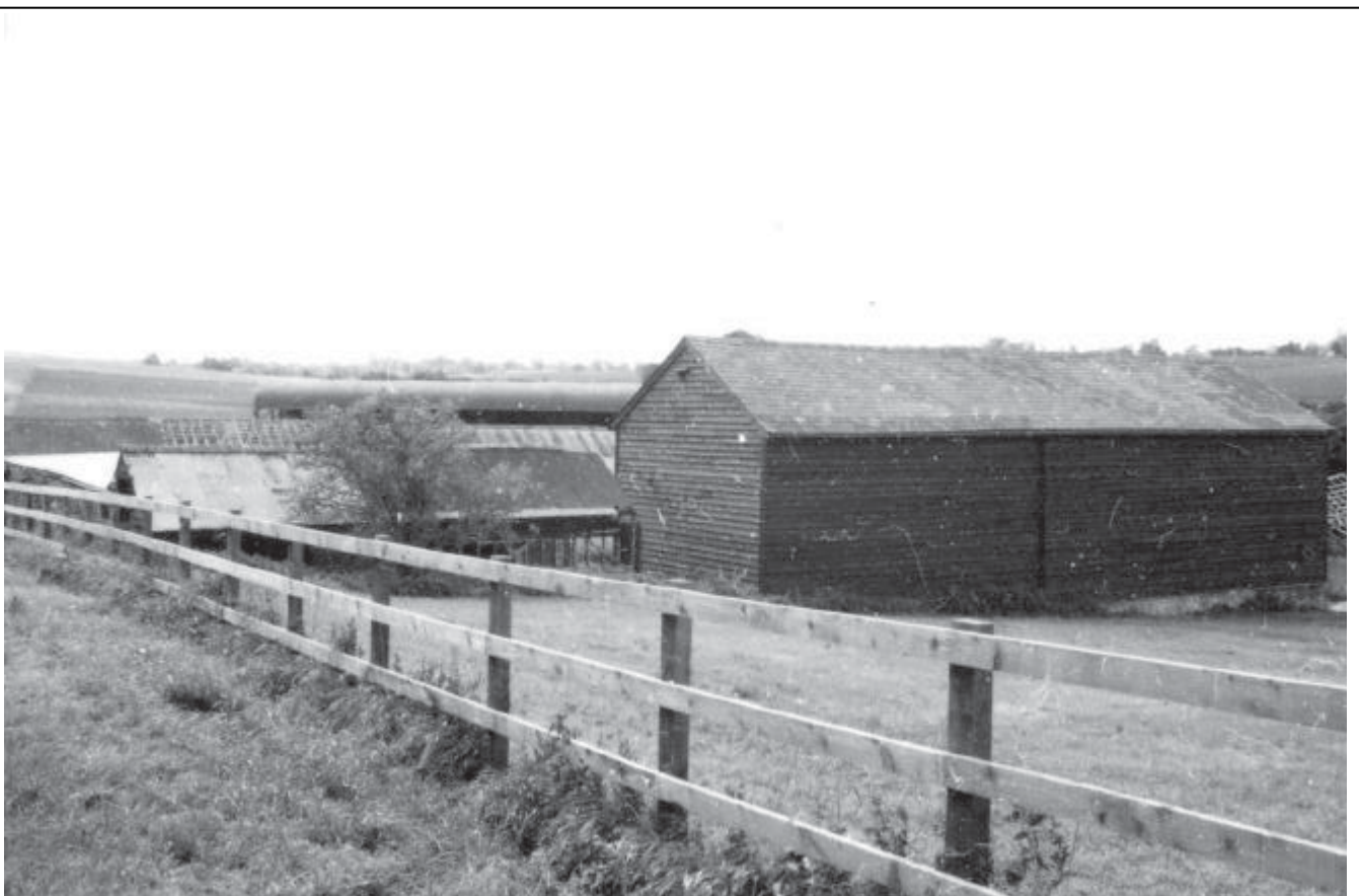
Plate 4b: Barn 2, northern elevation after renovation
