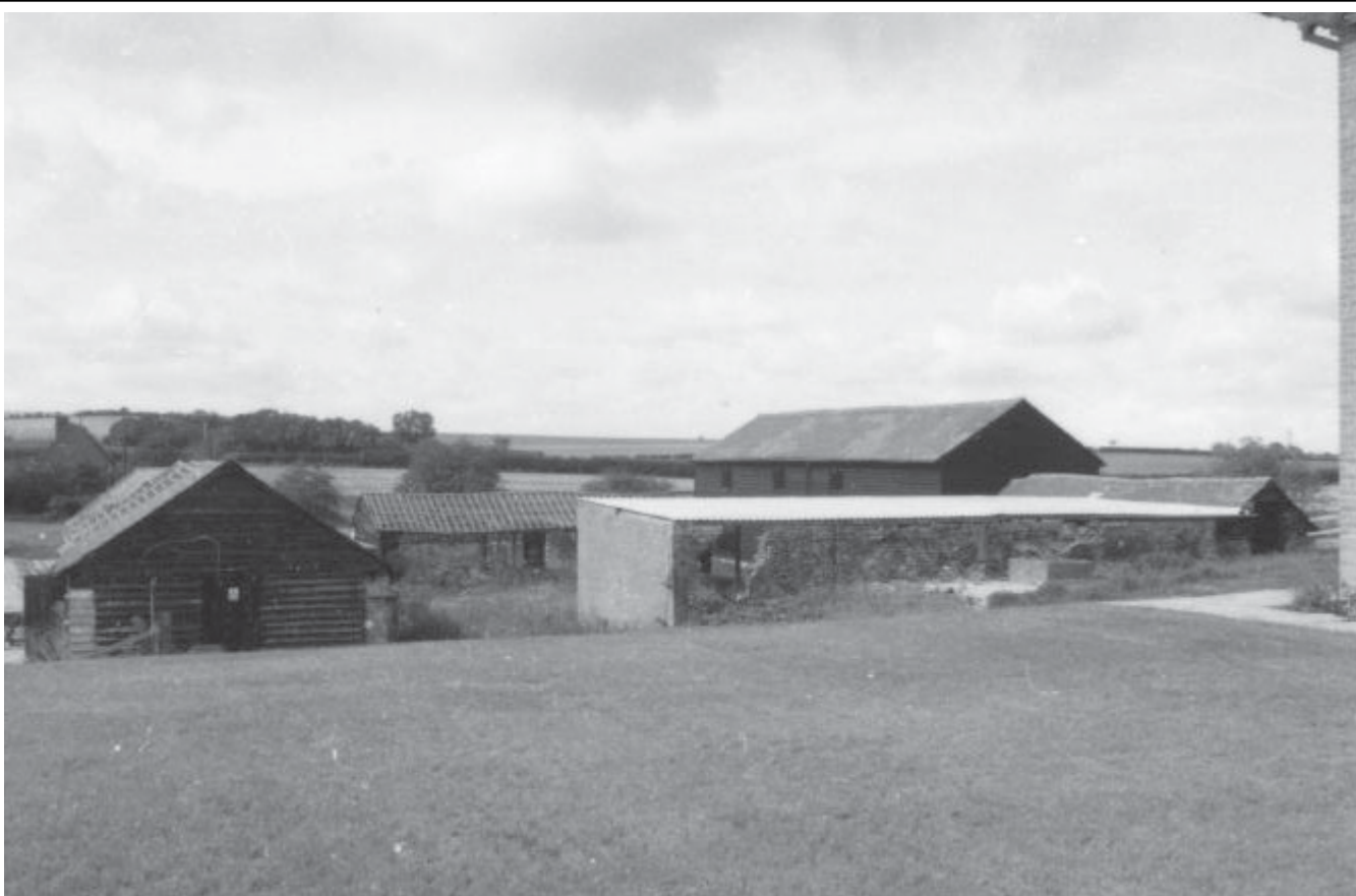
Plate 1b: General view of site from the east
