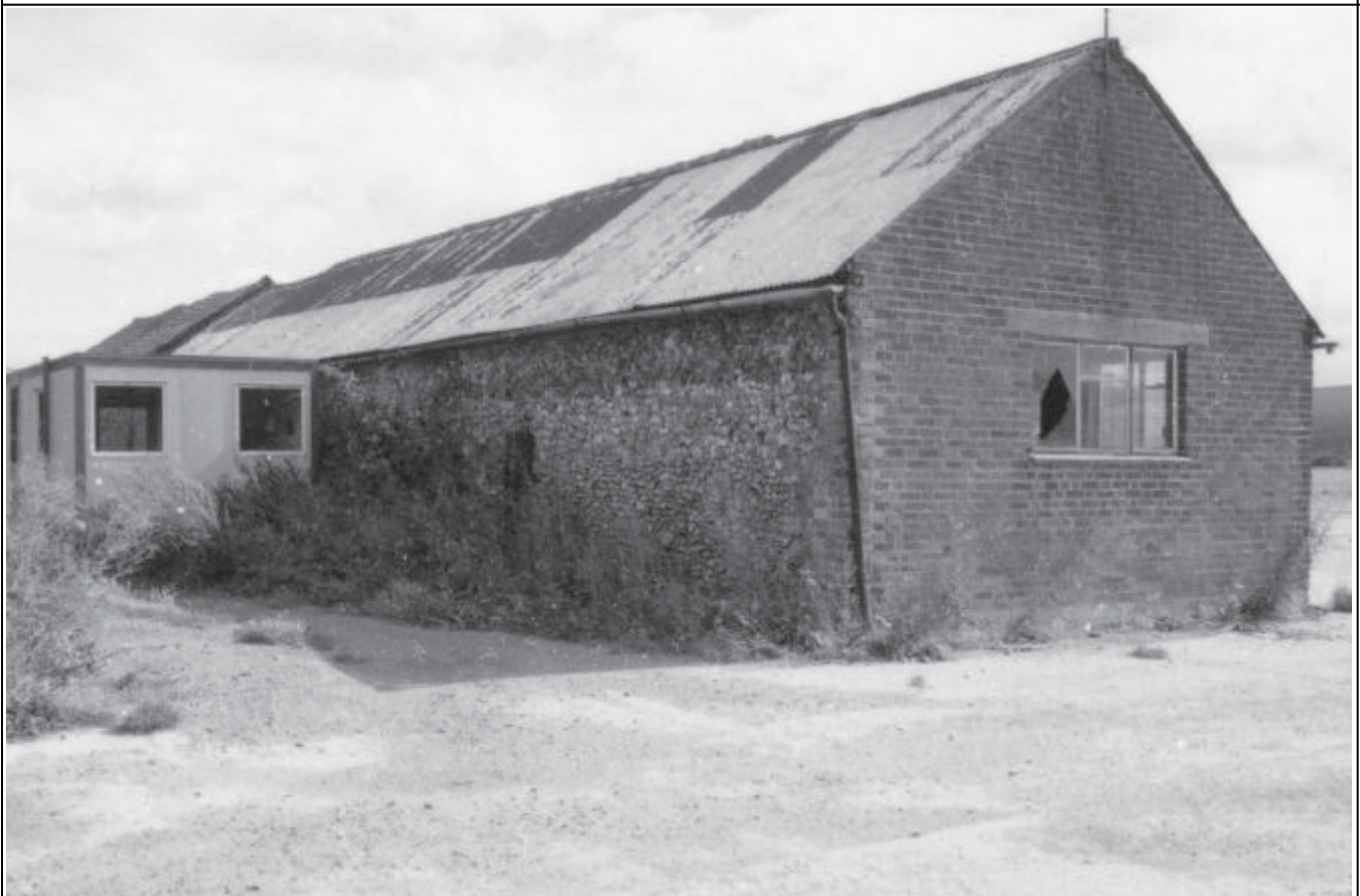
Plate 9b: Barn 4, northern and western elevations
