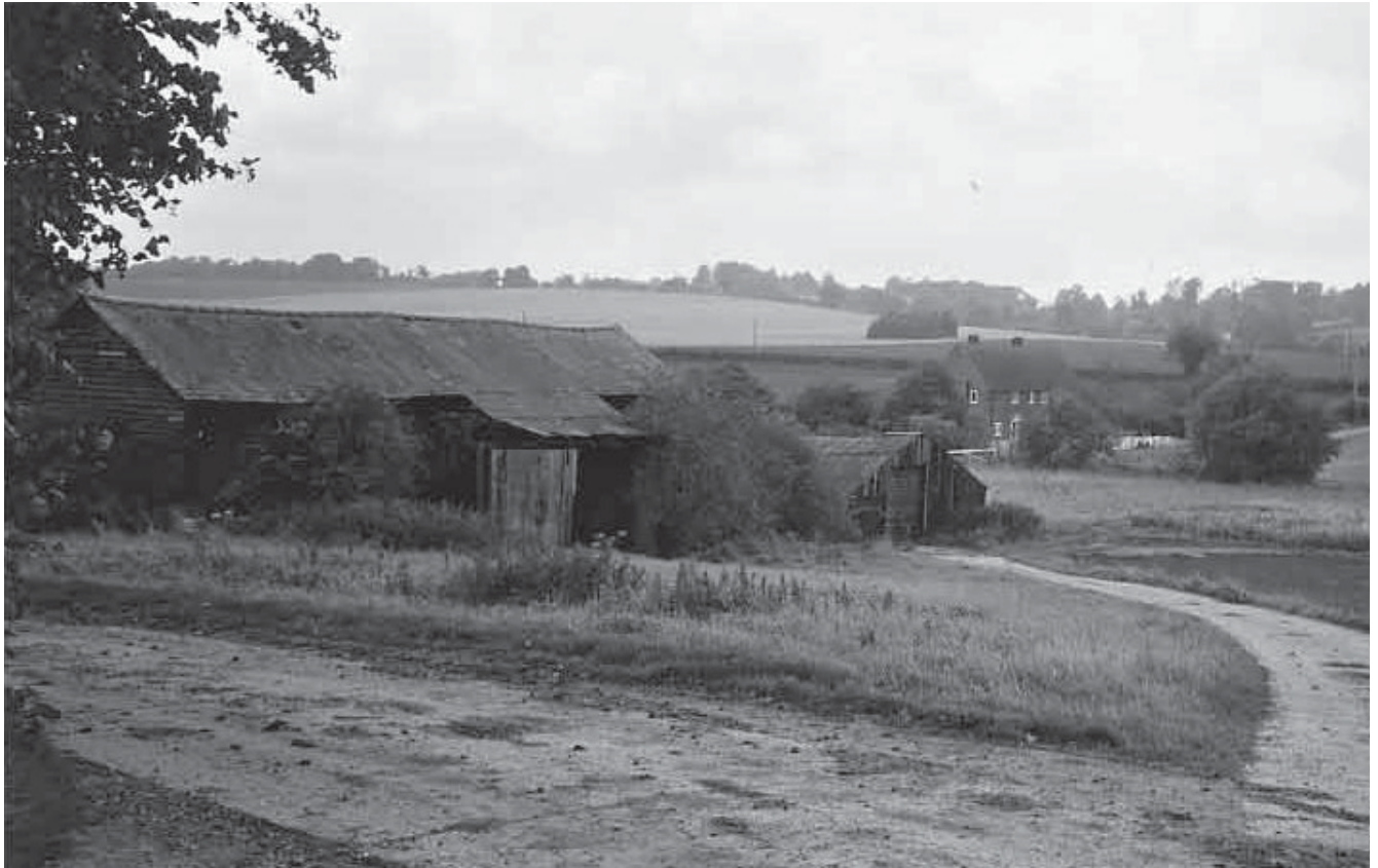
Plate 4a: Barn 2, northern elevation before renovation
