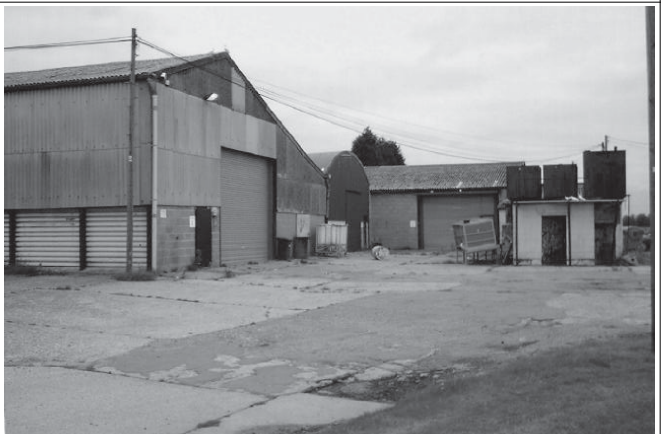
Plate 2b: Units 1, 1a and 2 from the south-east
