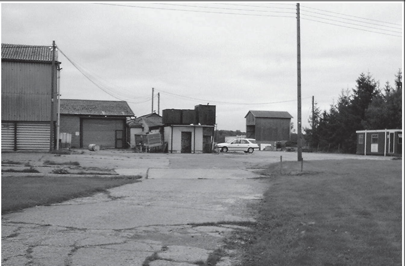
Plate 1b: General view of site from the south
