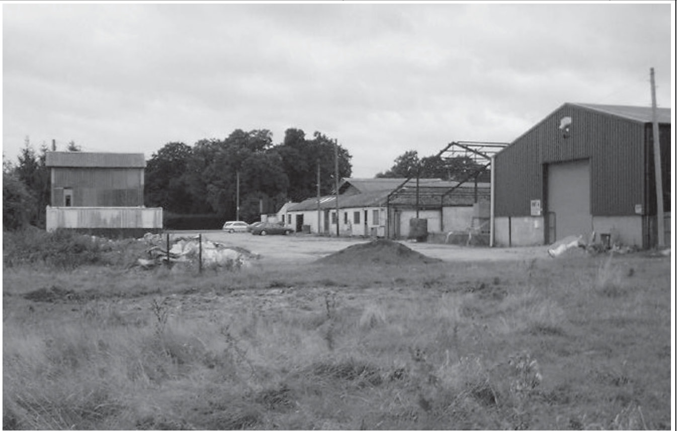
Plate 2a: General view of site from the north
