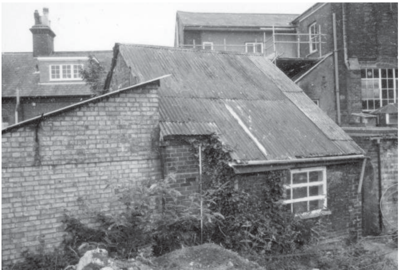
Plate 2b: General view from the north
