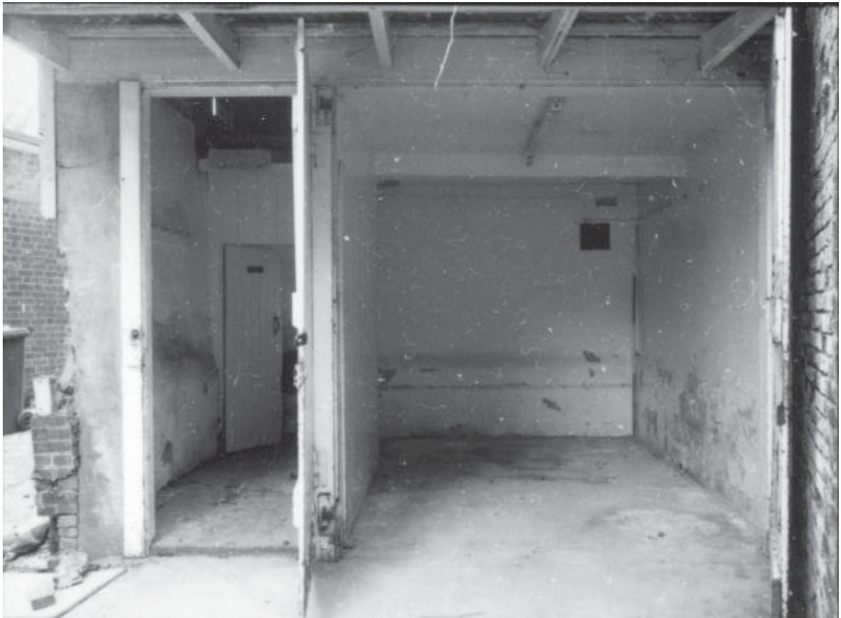
Plate 1b: Southern elevation from the south
