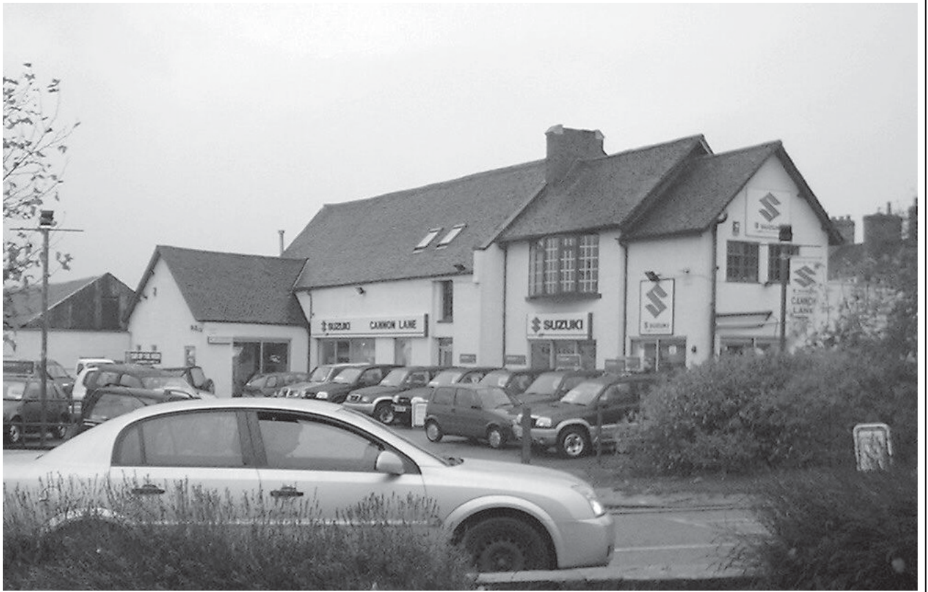
Plate 11: Building 15, northern and western elevations
