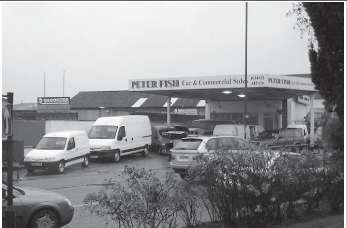
Plate 12: Building 16, northern elevation
