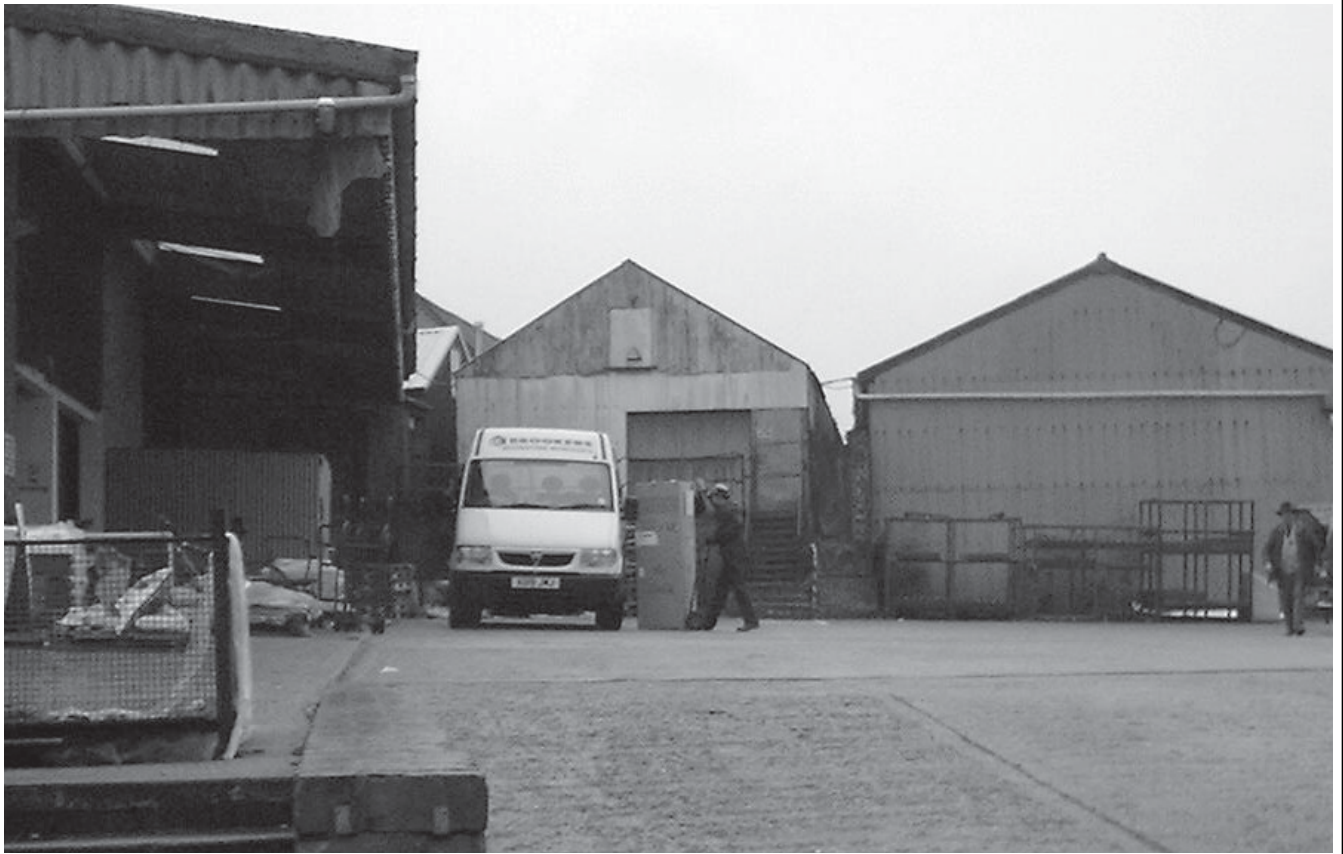
Plate 7: Upper yard, looking west
