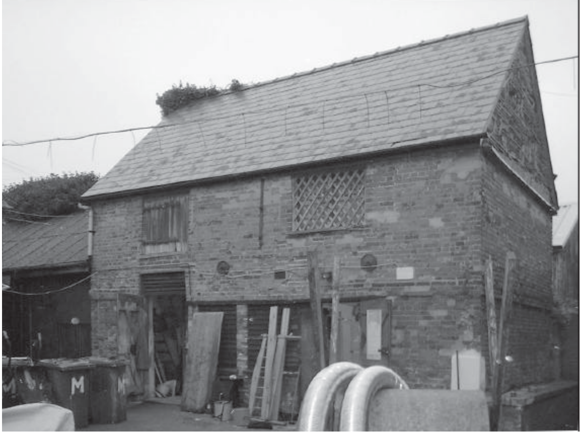
Plate 9: Building 12, southern and eastern elevations
